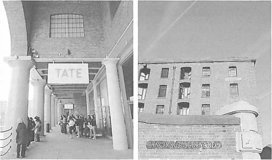
Figure 3.4 Galleries and apartments now occupy nineteenth-century industrial infrastructure in Liverpool
