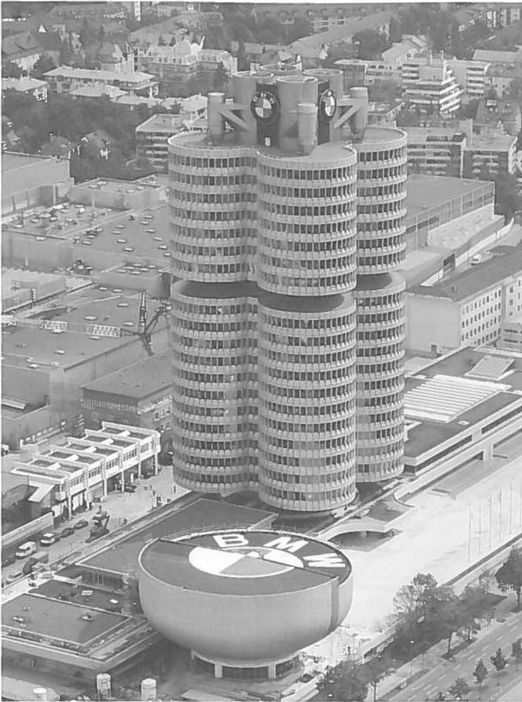
Figure 11.1 The BMW headquarter office in Munich, Germany
