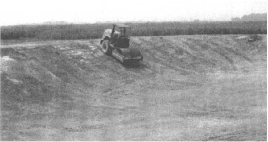
FIGURE 6-12. *Final Smooth Rolling of FGD Material.*
