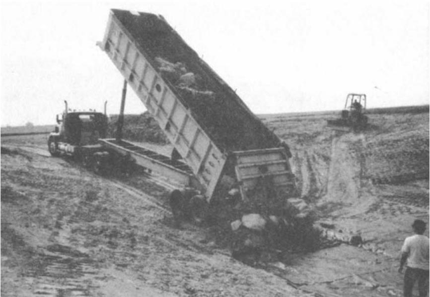
FIGURE 6-9. Truck Unloading FGD Material.
