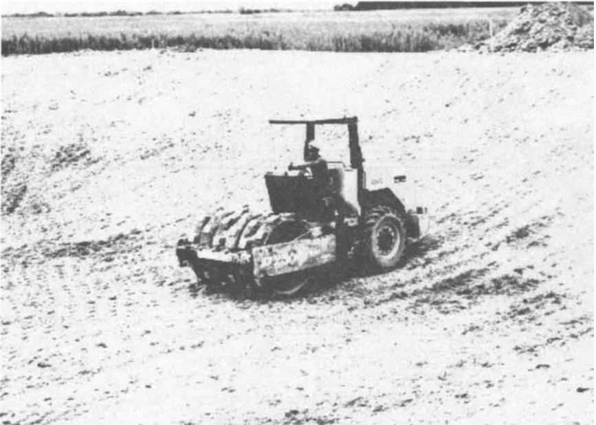
FIGURE 6-6. Compaction of Onsite Clay.
