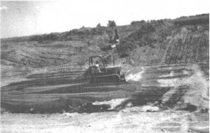
*FIGURE 6-8. Spreading of Sand.*
