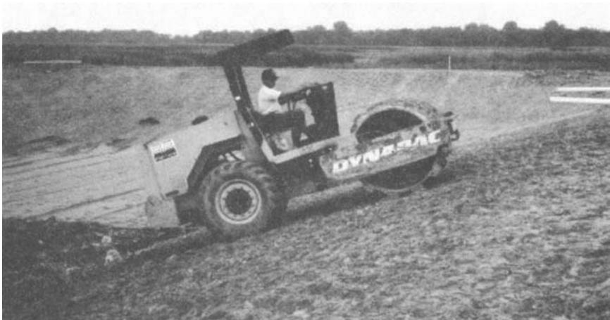
*FIGURE 6-11. Compacting FGD Material on a Side Slope.*
