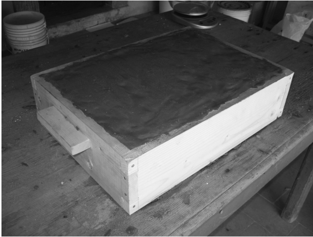
Figure 16.2 The production of an adobe block. The wooden mold is manually filled with wet earth.
