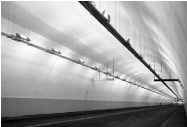
15.2 Umberto I tunnel in Rome.
