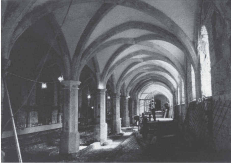
67 Windsor Castle. Undercroft below St George's Hall. Until the fire of 1992 this space was cluttered with seventeenth-century and later partitions. Refurbishment has revealed a double-aisled vaulted basement of a splendour and scale comparable with Fountains Abbey, Yorkshire. (Photograph: English Heritage and Royal Palaces.)
