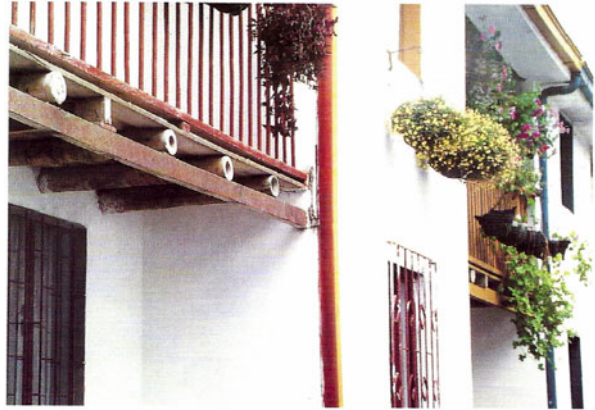
Fig. 9.20 City houses with bamboo construction and plastered walls in Manizales, Colombia (Liese and Kumar 2003)
