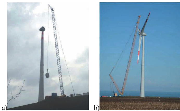
Figure 46. Installation of the nacelle a) and of the rotor b).
