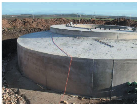
Figure 42. Foundation block before lateral backfilling.
