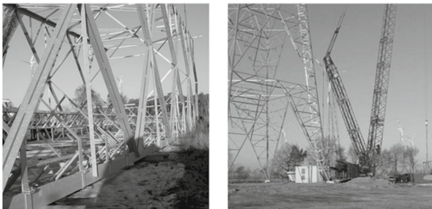
Figure 28. Erection of a lattice tower
