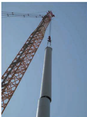
Figure 45. Installation of the 25m steel segment.
