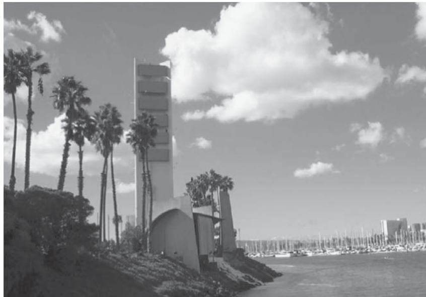
Figure 20 Oil and gas drilling in the Los Angeles area. A camouflaged rig on Island Grissom, a manmade drilling island near Long Beach, CA. Photo by J. Jepson (California Department of Conservation 2007)
