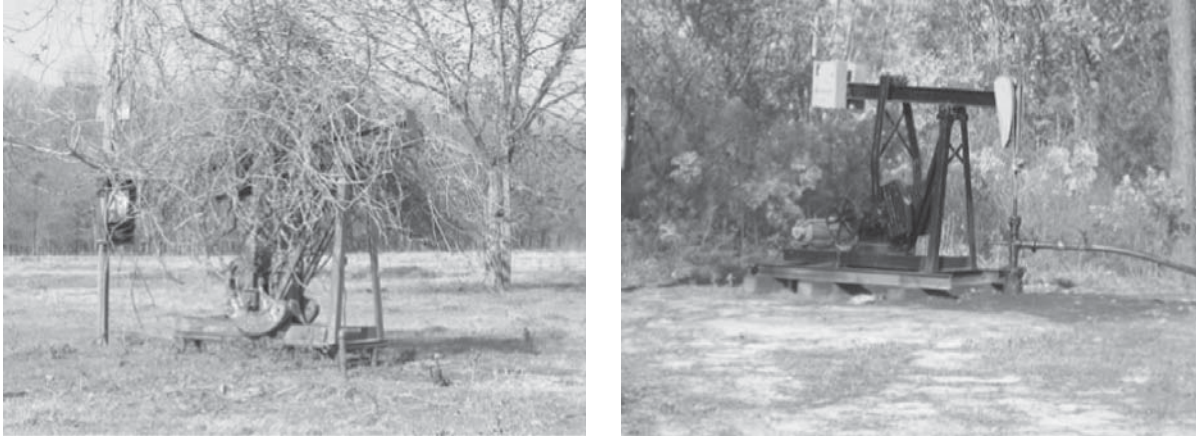
Figure 24 (a) A typical orphaned well, (b) A well after reactivation (California Department of Conservation 2007)
