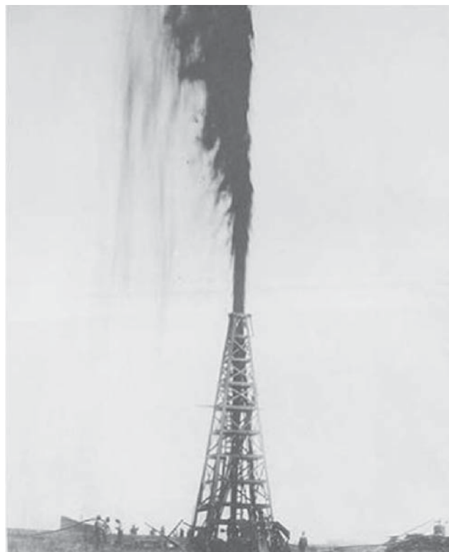
Figure 11 A gusher (uncontrolled flow of oil and gas after oil-bearing strata is ruptured by drill bit) used to be common site at most successful drilling, circa 1900 (Energy Industry Photos)
