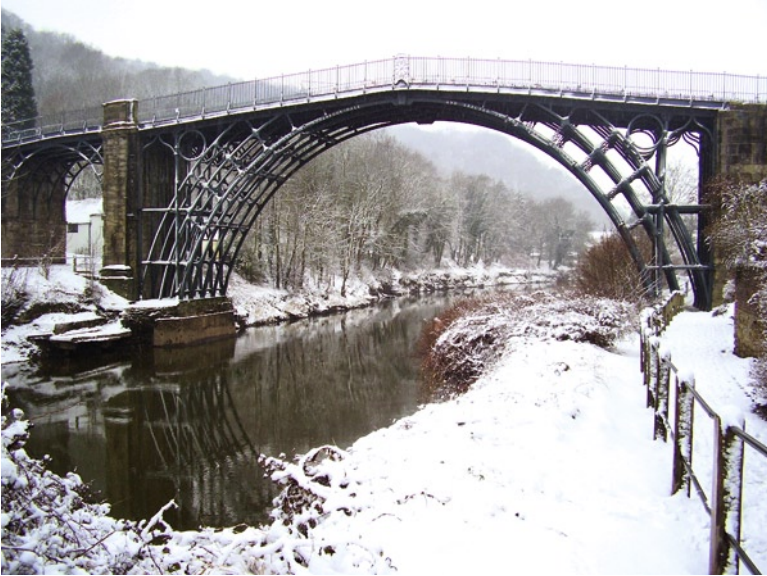
Fig. 3.5 The iron bridge (Shropshire). (Photo: Paul Belford)
