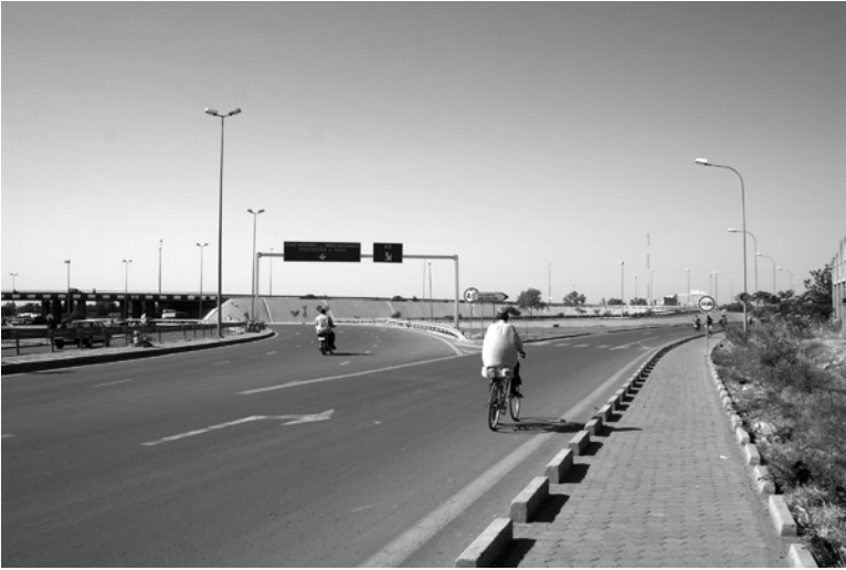
Figure 6.3 Southern interchange, Ouagadougou. Photo by Jonas Haenggi.
