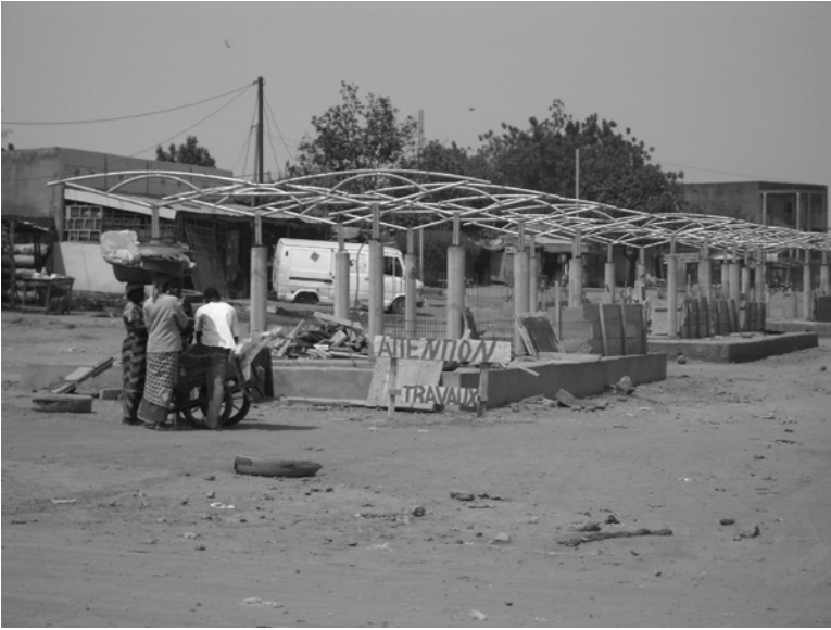
Figure 4.5 The new market of Gounghin under construction. Photo by Ola Söderström.
