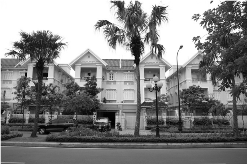
Figure 5.2 A street in Ciputra Hanoi International City. Photo by Stephanie Geertman.
