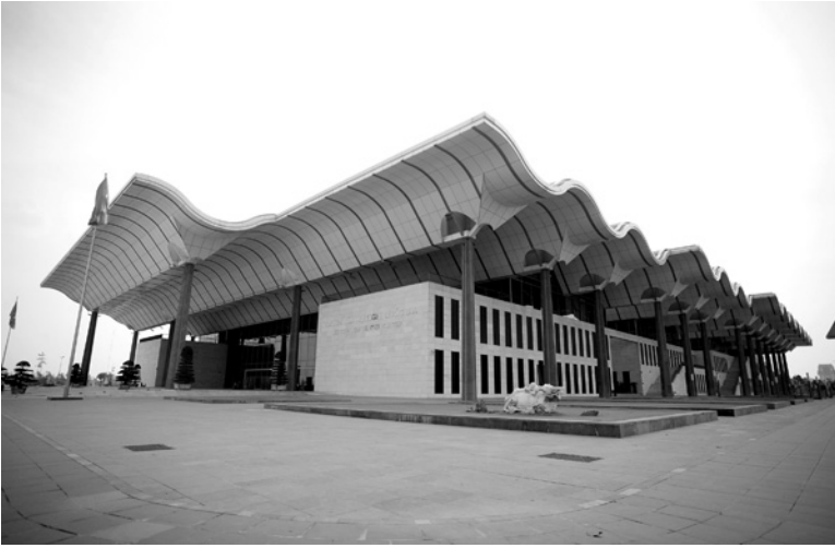
Figure 5.8 NCC's undulating roof, Hanoi. Photo by Chu Giap.
