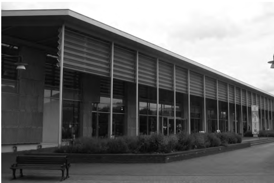
Figure 20.26 Main south façade of Heelis Building, Swindon, UK
