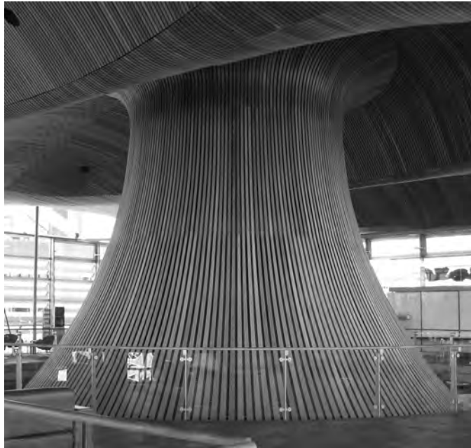
Figure 20.24 The funnel acting as the stack effect for the Siambr viewed from the public space
