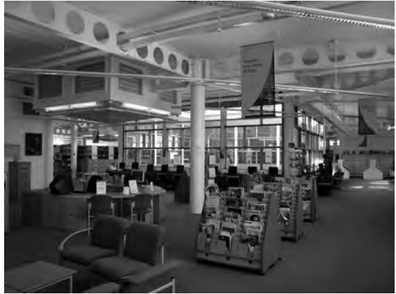
Figure 27.7 View of the third floor showing the central lightwell, exposed thermal mass, castellated beams and dedicated ventilation stacks
