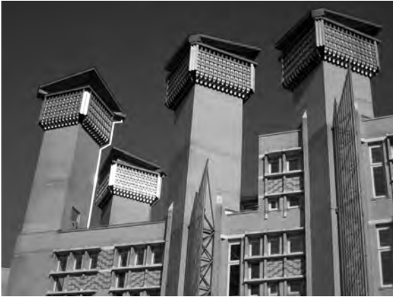
Figure 27.6 View of south façade showing perimeter stacks, shading fins, deep window reveals and overhangs
