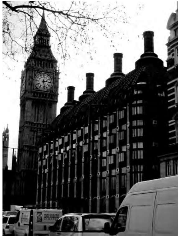
Figure 17.14 Portcullis House, London
