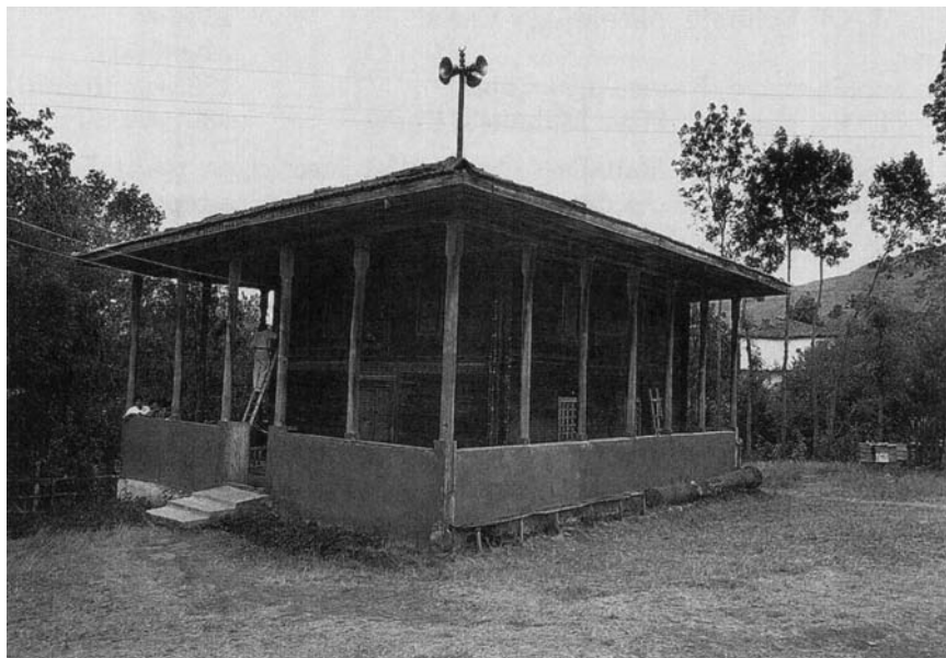
Figure 4.2. Samsun, Kavak, Bekdemirköy, Camii. Boards below the moulding were cut after 1585. Boards above the moulding were cut in 1876. (P. I. Kuniholm, ADP)
