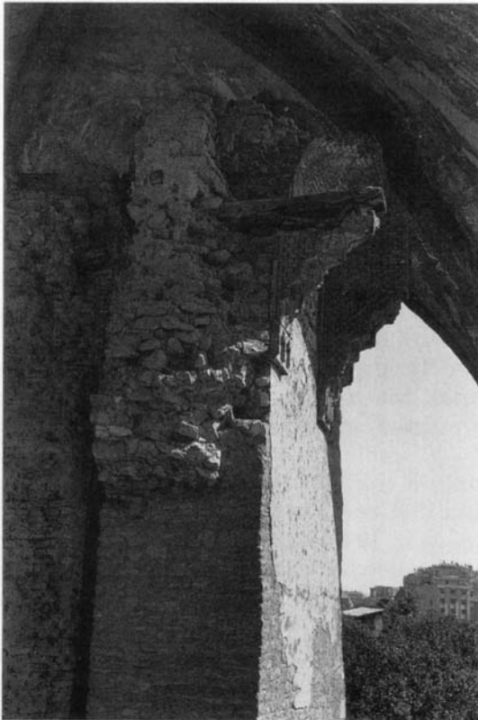
Figure 4.22. Konya, Selçuklu Sarayı. Lower portion of the tower. Last preserved ring is 1174. (P. I. Kuniholm, ADP)
