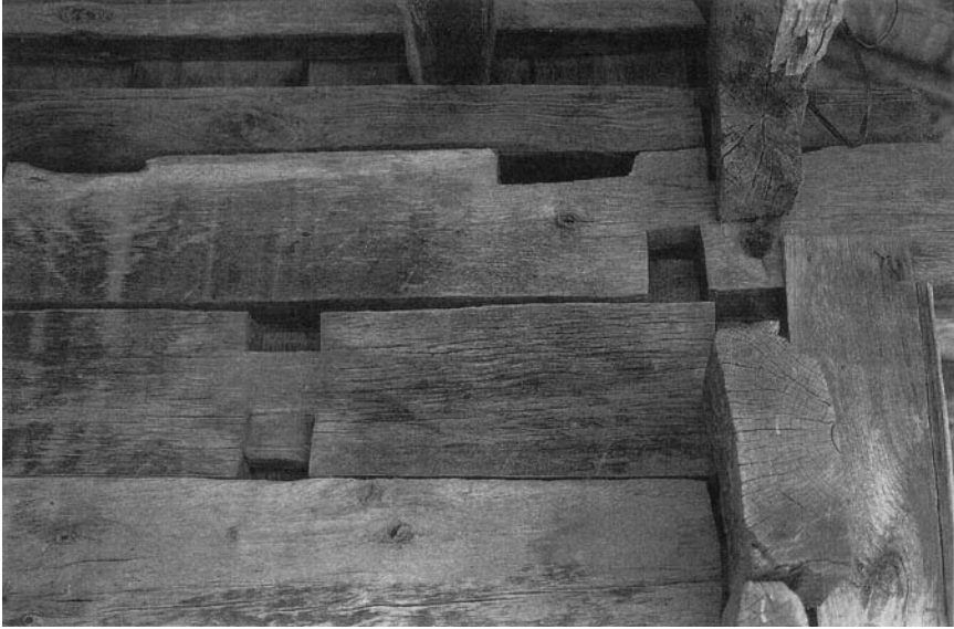
Figure 4.13. Ordu, Ünye, İkizce, Eski Cami, detail of northeast corner. Reused timbers with end dates spread out over 127 years from 1395 to 1522. (P. I. Kuniholm, ADP)
