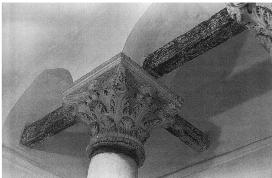
Figure 4.14. Bursa, Yesil Camii, alcove next to the front door. The beams have a last-preserved ring from 1413. (P. I. Kuniholm, ADP)
