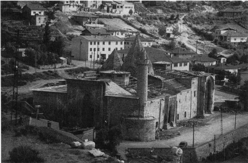
Figure 4.7. Divriği, Ulu Cami, current roof repairs. (P. I. Kuniholm, ADP)
