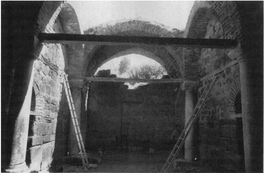
Figure 4.20. Afyon, Sincanlı, Boyaliköy Medresesi, interior. The oak tie-beams, wall-stretchers, and door-lintels were cut in 1206. The “beam” in the foreground is a poured concrete replacement. (P. I. Kuniholm, ADP)
