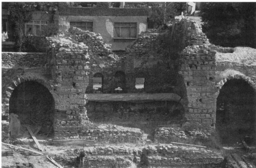
Figure 4.16. Bursa, I. Yildirim Beyazıt Darü'ssıfasi, detail of south end with timbers cut in 1400. (P. I. Kuniholm, ADP)
