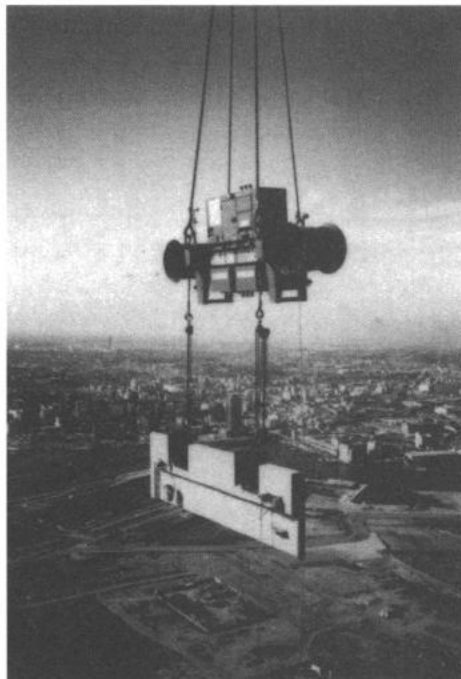
Figure 17.7 Actively controlled crane used during construction of the Yokohama Landmark Tower.
