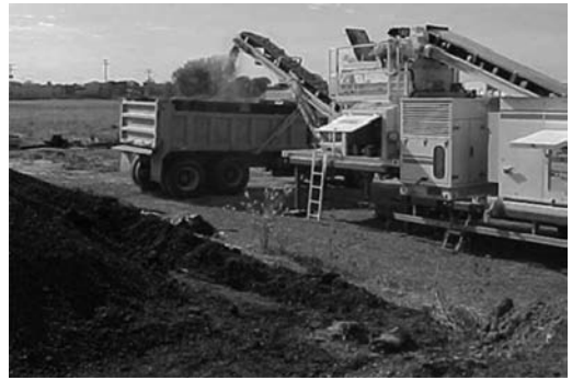
Figure 11. Foamed asphalt stabilized material production (Romanoschi et al., 2004).
