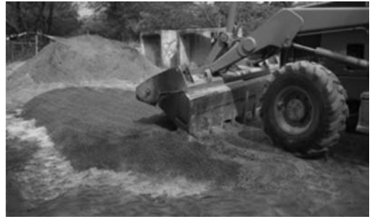
Figure 7. Mixing RCC materials.
