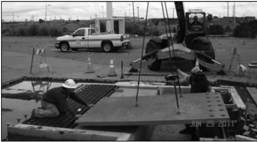
Figure 4. Deck joint installation.
