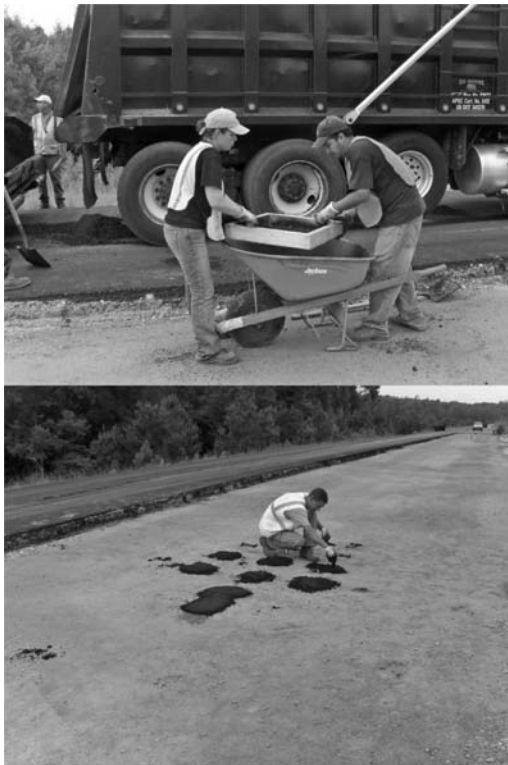
Figure 2. Procedure followed to protect the gauges during construction.
