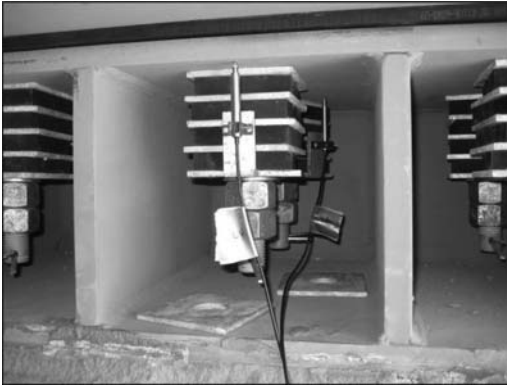
Figure 11. LVDTs for monitoring washer movements (Instrument #3 and #4 in Figure 7).
