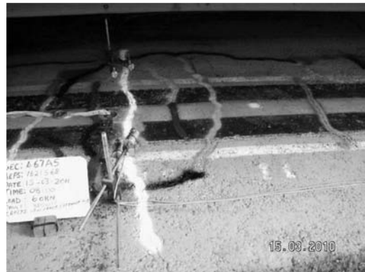
Figure 16. Circular crack formation toward the end of the test.
