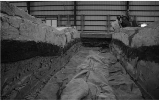
Figure 8. MRC-W test trench.
