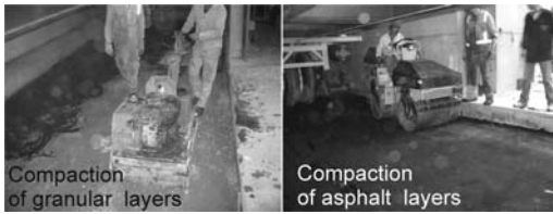
Figure 9. Compaction of the pavement layers with small equipment.
