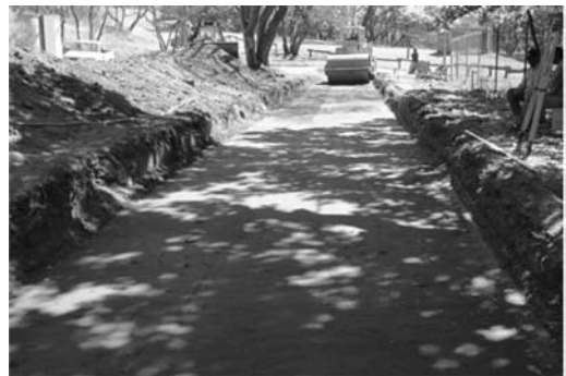
Figure 3. Subgrade preparation and compaction.
