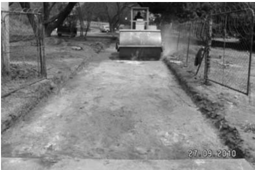
Figure 6. Compacting base with roller compactor.
