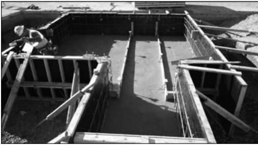
Figure 3. Formwork for test structure.
