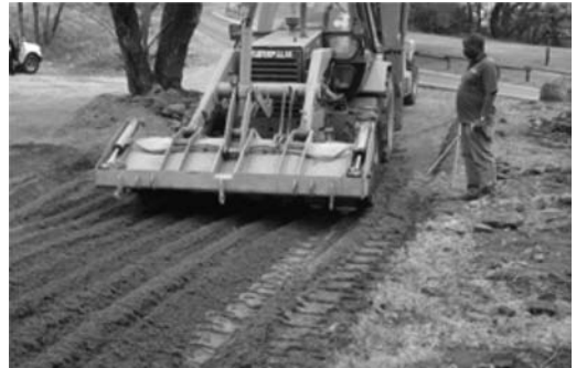
Figure 8. Spreading RCC materials.
