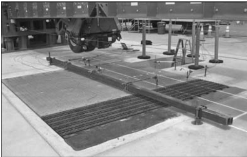
Figure 6. Test structure prior to start of testing.
