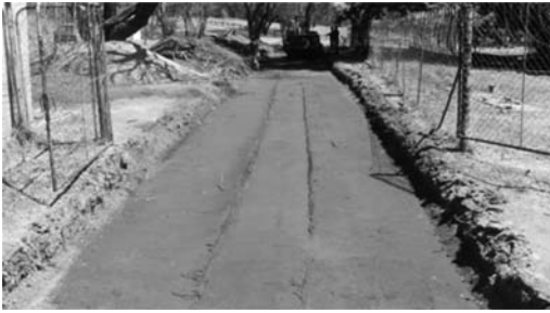
Figure 4. Subbase construction.
