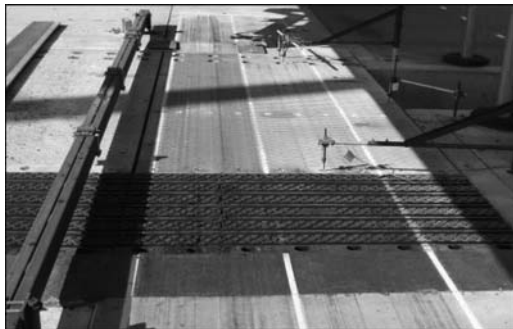
Figure 24. General view of structure after testing.
