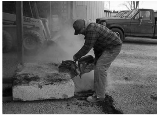
Figure 20. Cutting of dowelled slab at contractor's yard.
