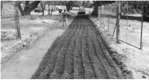
Figure 5. Mixing cement and fly ash with in situ material.
