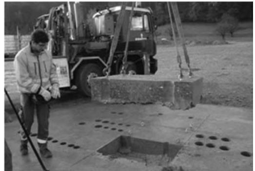
Figure 8. Extraction of asphalt slab from test pavement.
