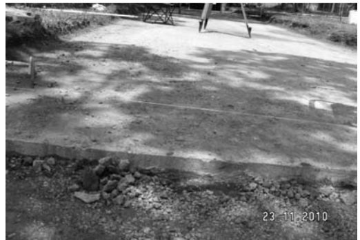
Figure 9. RCC layer after Phase 1 construction (mechanical equipment).
