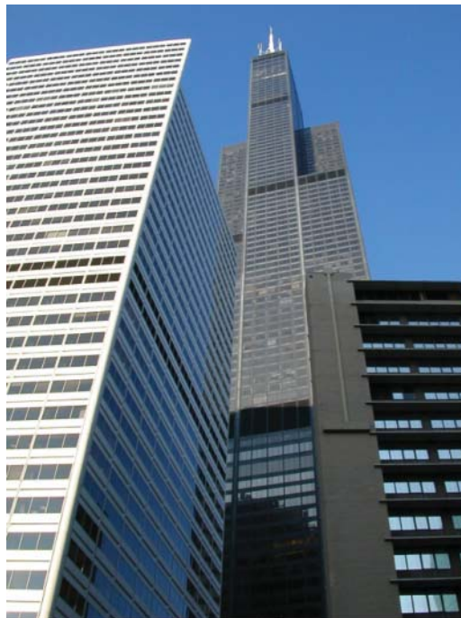
Fig. 3.8 The Willis Towers.
