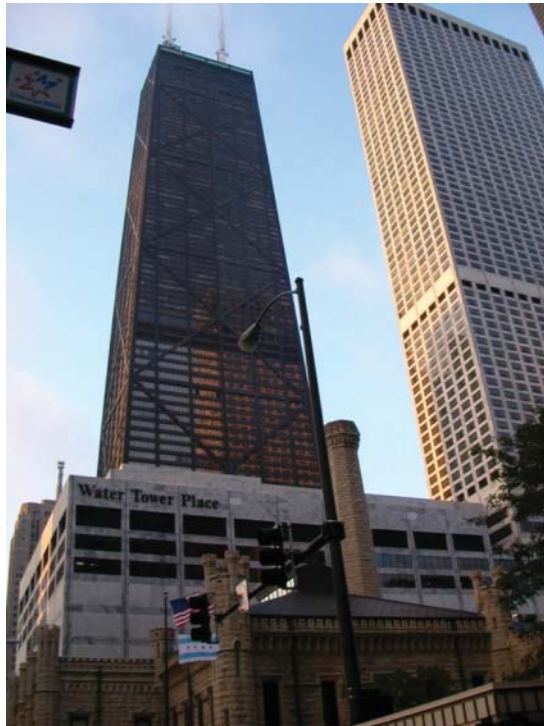
Fig. 3.6 John Hancock Center in Chicago.
