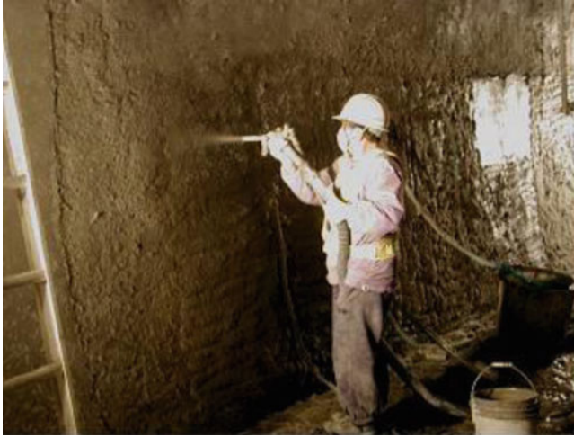
Fig. 3.14 Execution of R/ECC liner reinforcing construction
