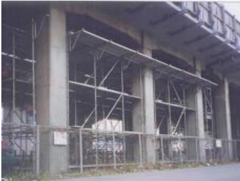
Fig. 3.20 Railway viaducts for test construction
