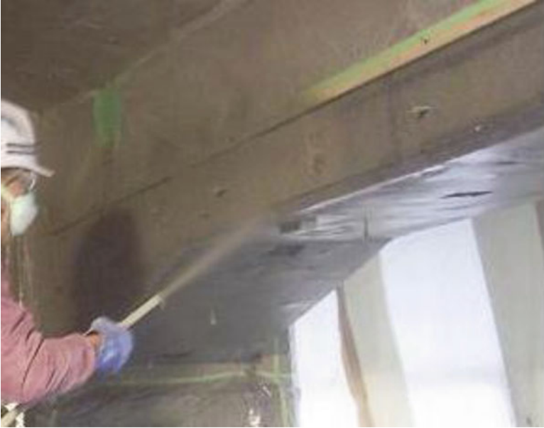
Fig. 3.21 Execution of test construction
