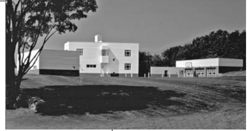
© Anthony Ames, Architect
