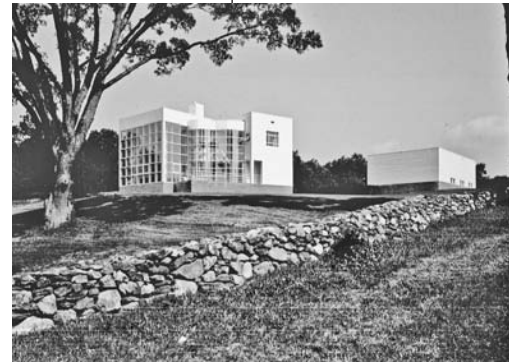
© Anthony Ames, Architect
