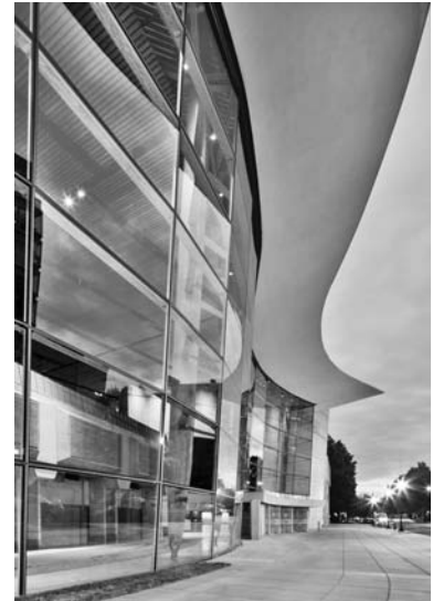
View of front entrance— looking north
