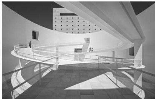
This three-floor podium building (left), silent in its forms, includes two levels below ground. The three levels are connected by circular ramps within an elliptical central courtyard.
