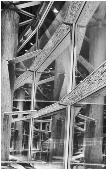
Close-up of wood curtain wall
