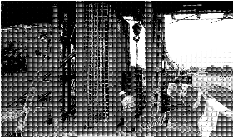
Figure 4 Typical repair of a bridge pier using stainless steel reinforcement
