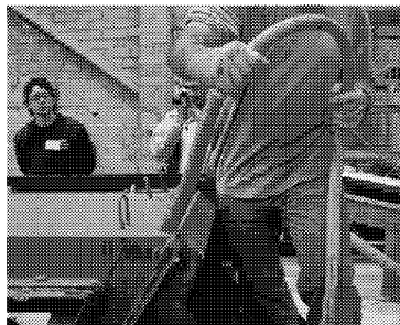
Figure 5 Needle vibration used in the compaction of the conventional concrete
