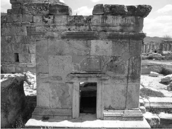
Figure 5.4 The mausoleum of Flavius Zeuxis; the inscription above the door records his seventy-two trading journeys to Italy
