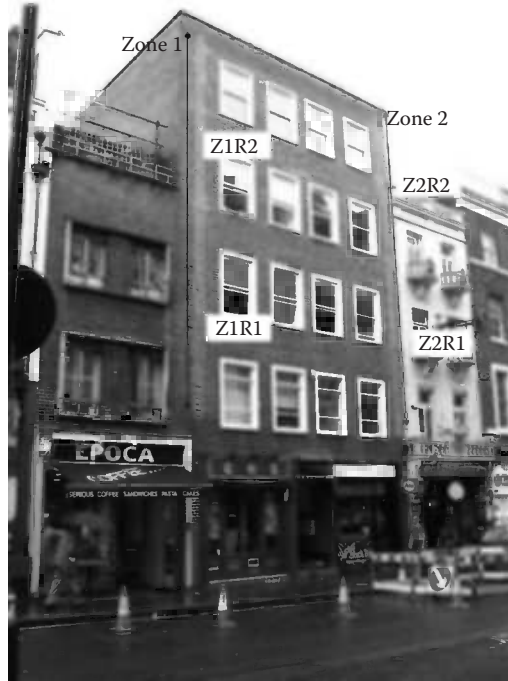
Figure 8.2 Two zones of a simple impressed current cathodic protection system applied to a Georgian brick building in a conservation area in London.
