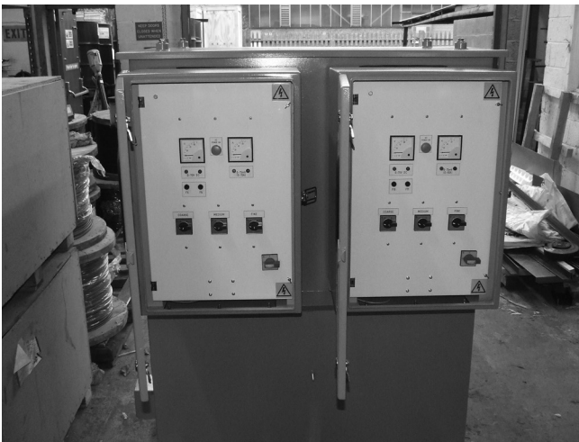
Figure 10.4 Conventional transformer rectifier units.
