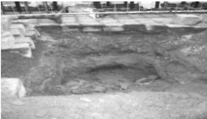
Figure 12.5 Investigation of the ceiling from the top.
