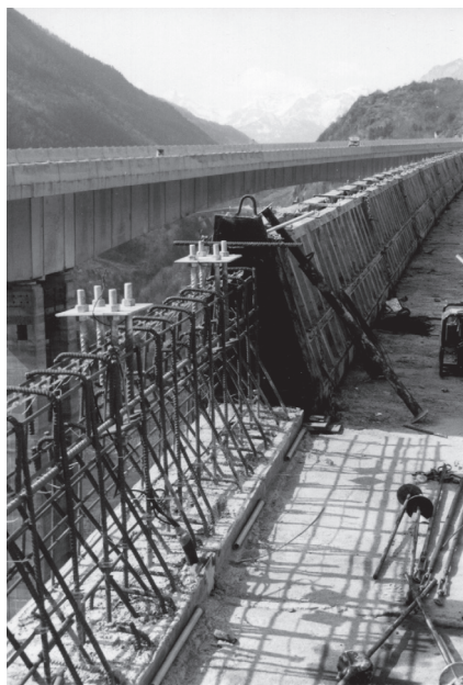
Figure 9.5 CP integration to new bridge safety barriers.
