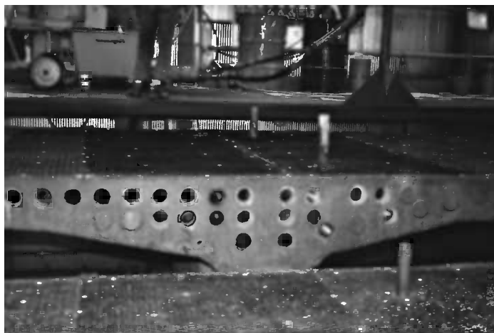
Figure 9.4 Italian bridge segments with integrated deck CP.
