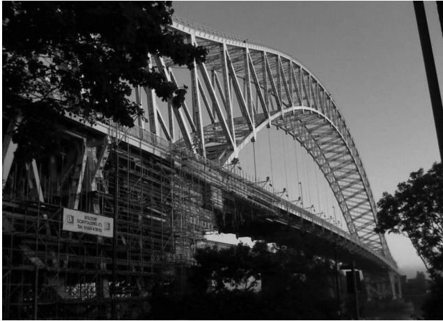
Figure 12.14 Silver Jubilee Bridge.
