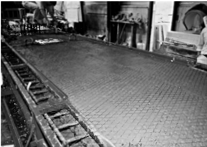
Figure 9.3 CP anode integrated within precast deck slab.
