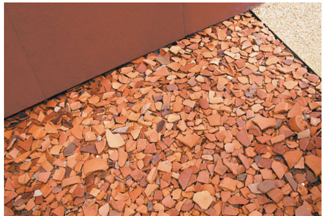
Figure 12–7 Example of shattered clay pots used as a pavement surface.
