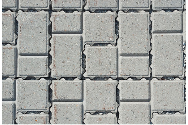
Figure 12-28 Permeable concrete pavement with gravel-filled spaces.
