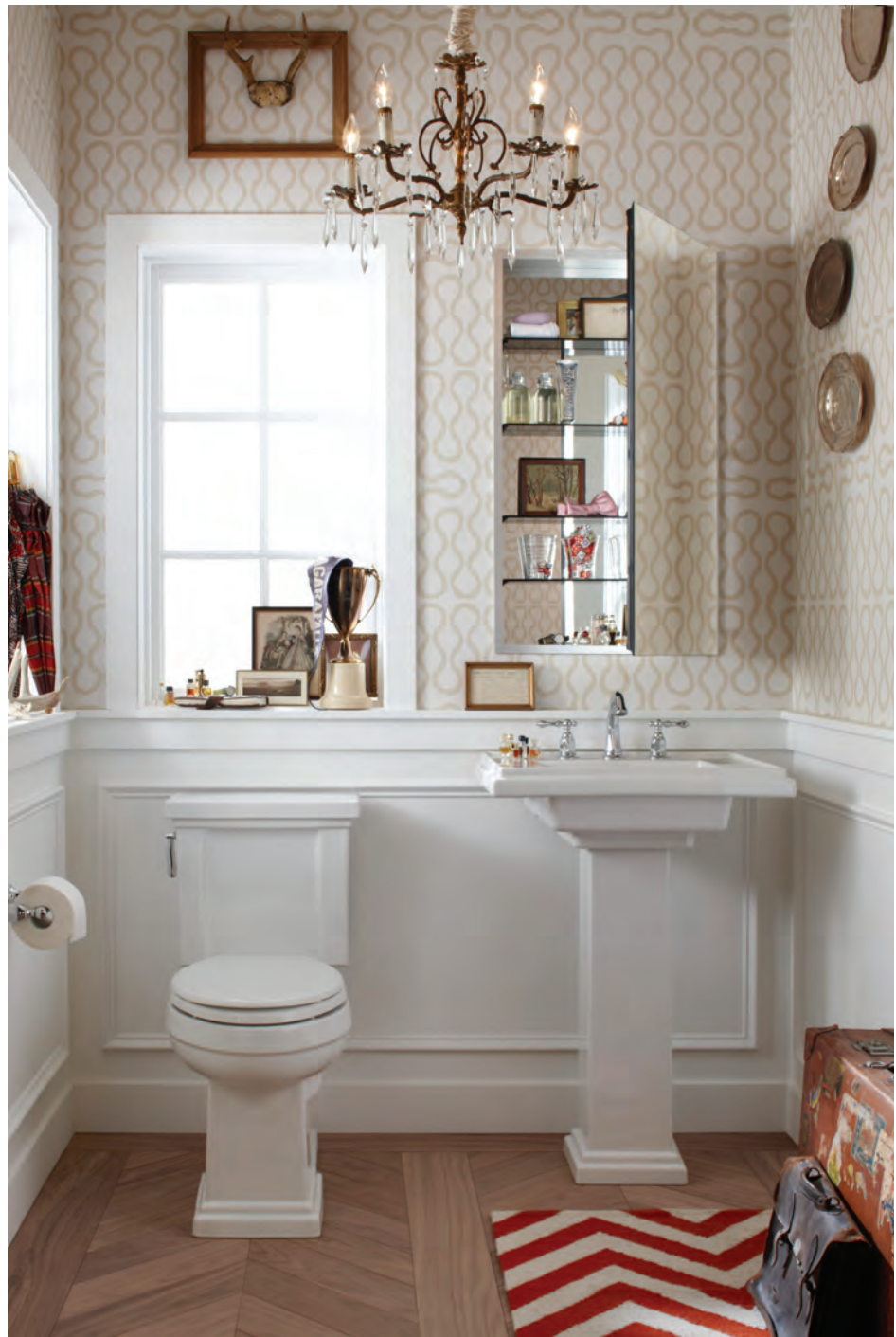
FIGURE 4.7 Pedestal lavatory: Pedestal lavatories are normally part of a suite by the plumbing fixture manufacturer. The details of the group of fixtures are repeated in the toilet and the bathtub. Courtesy of Kohler Co.
