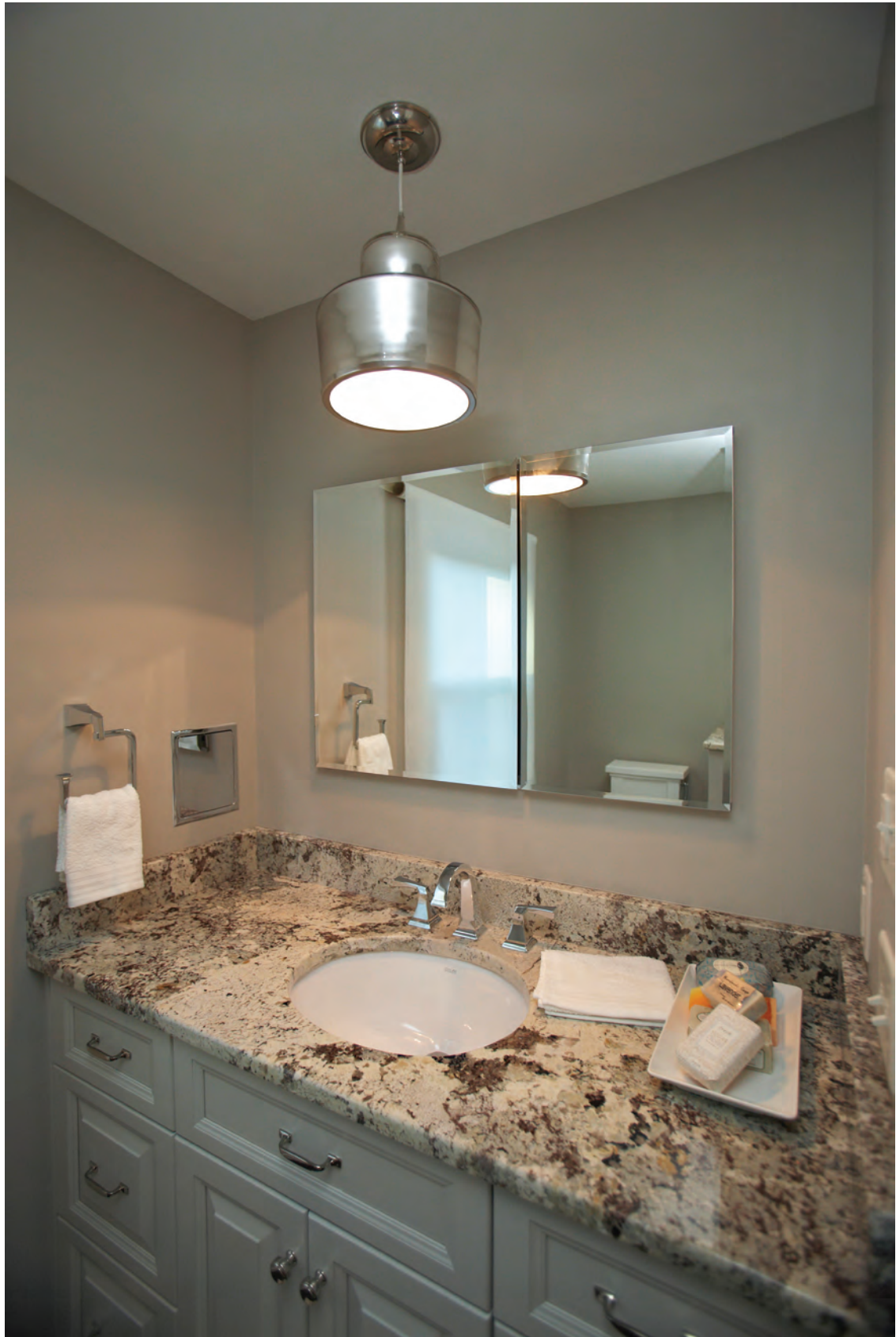
FIGURE 4.5 A lavatory installed under the vanity countertop.
