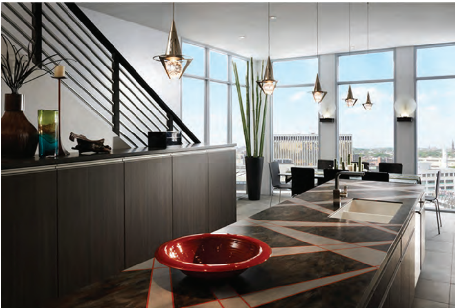
FIGURE 7.44 Solid surfacing materials can be combined dramatically because of their stable expansion and contraction properties.
