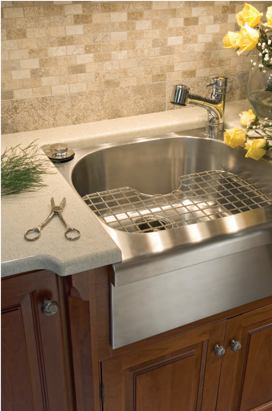
FIGURE 4.9 Mounting methods: An apron front stainless steel sink mounted below a quartz surface.
