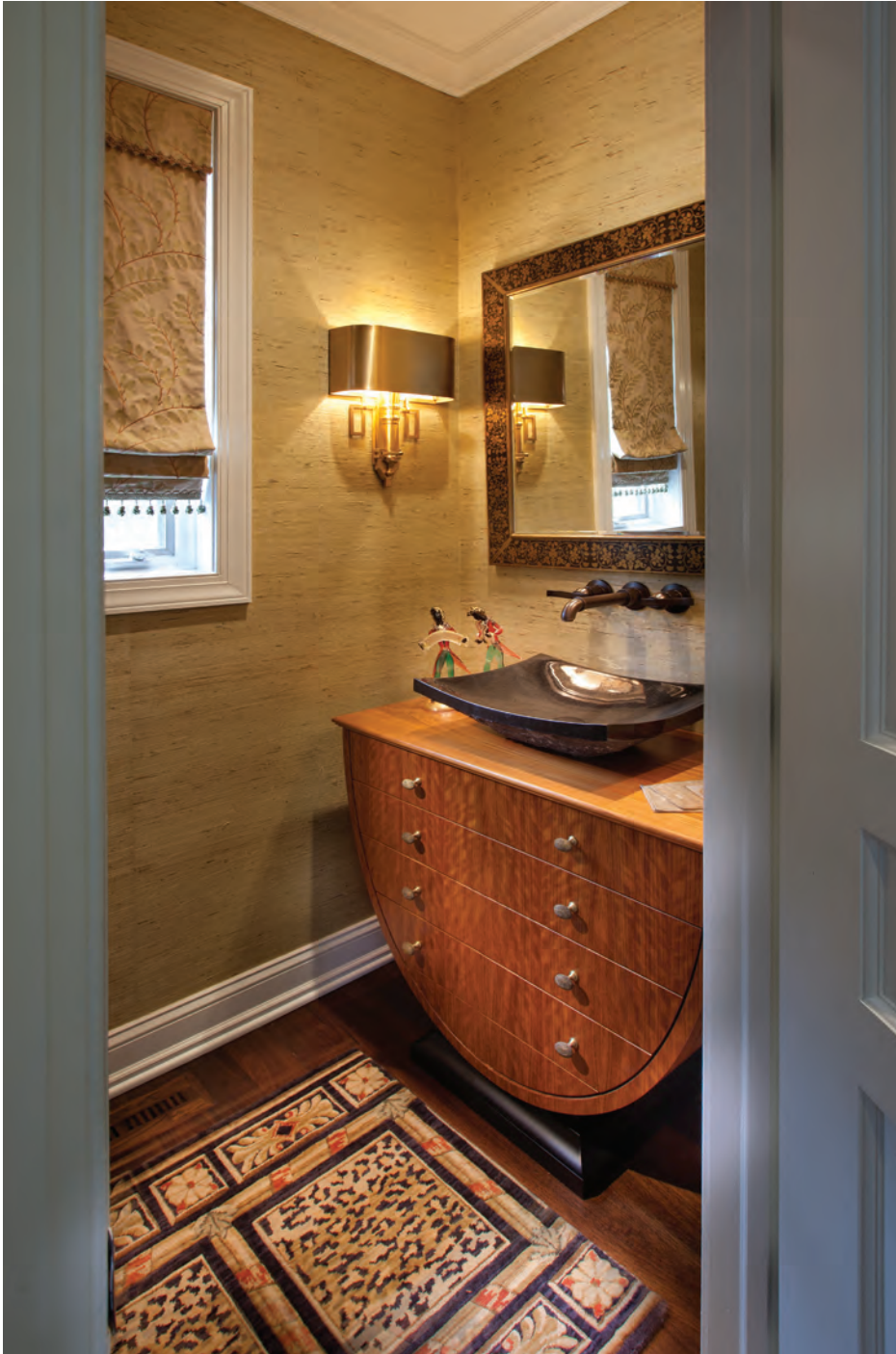
FIGURE 4.8 Vessel/above counter bowls: A stone vessel lavatory sits atop a connecting cabinet with wall-mounted faucets.
