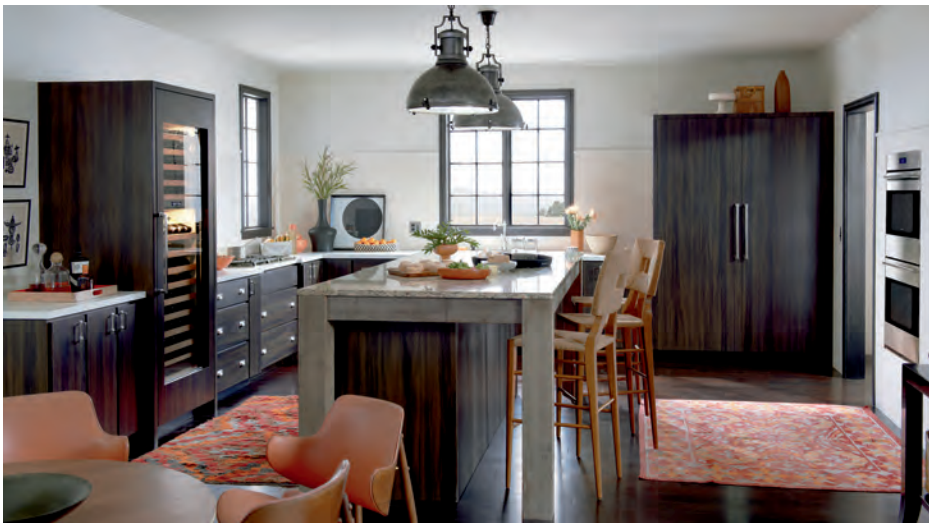
FIGURE 7.50 Granite is used as an accent on the island top. Note how the surface is supported by wood legs to the floor.
