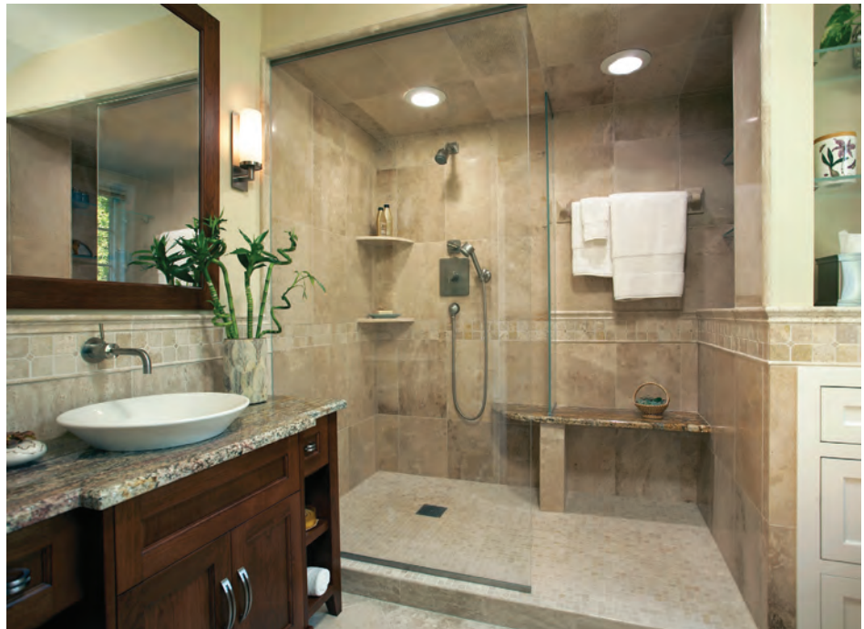
FIGURE 6.7 A curbless shower without a door. Note the shower seat extending into the shower area. Design by John Sylvestre, CKD. Photo by Karen Melvin Photography
