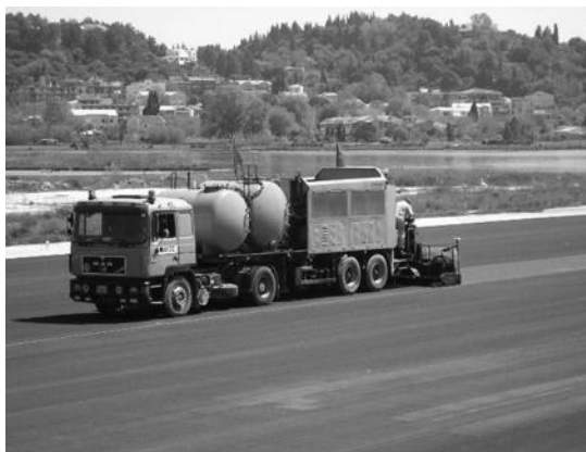
Figure 6.6 Typical slurry surfacing machine (application of micro-surfacing in airport runway).
