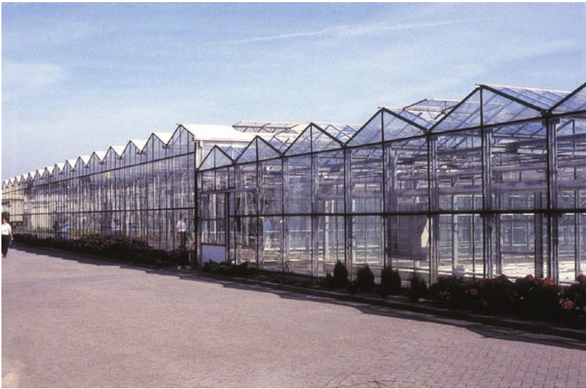
Photo 14.1. Venlo-type glasshouse, characteristic of production in the ‘Dutch agrosystem’.
