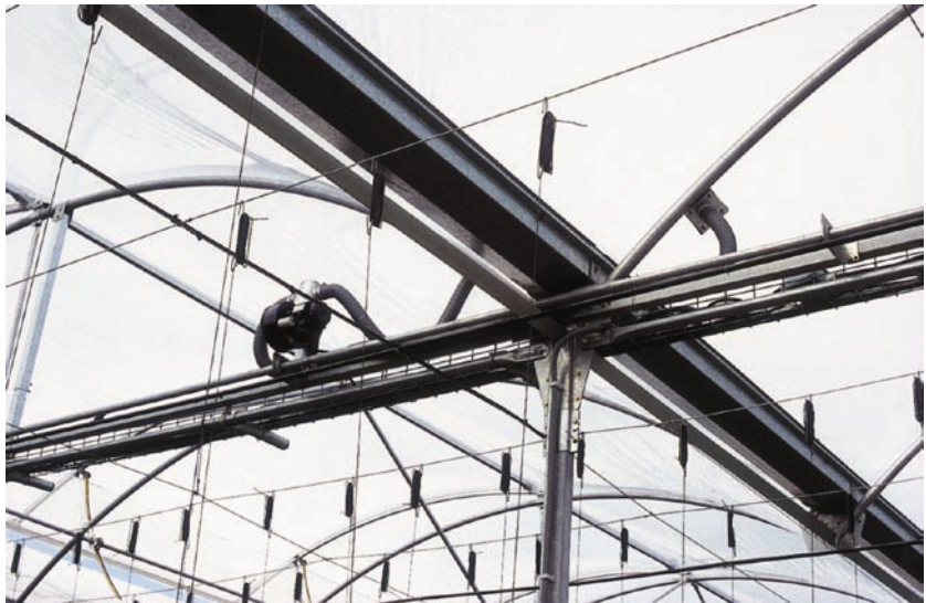
Photo 7.1. Greenhouses made of inflated double plastic film improve the insulation conditions but require special fixing systems.
