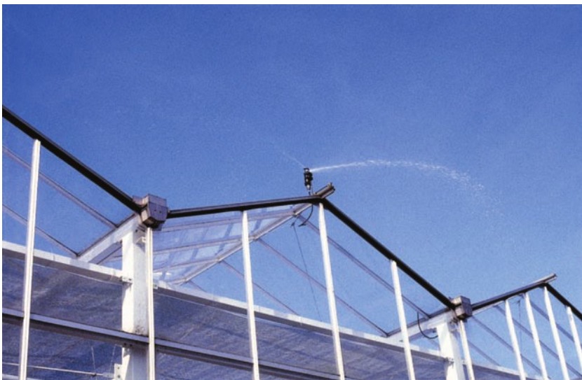
Photo 8.7. The 'irrigation' of the cover to cool the greenhouse has not been used in the Mediterranean.
