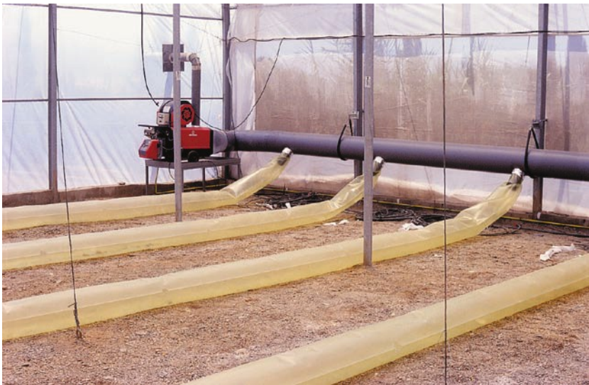
Photo 7.3. Indirect combustion hot air generator and flexible plastic air distribution pipes.
