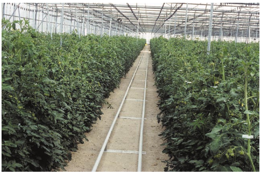
Photo 7.4. Metallic heating pipes that are also used as rails for the movement of trolleys and mechanized elements.
