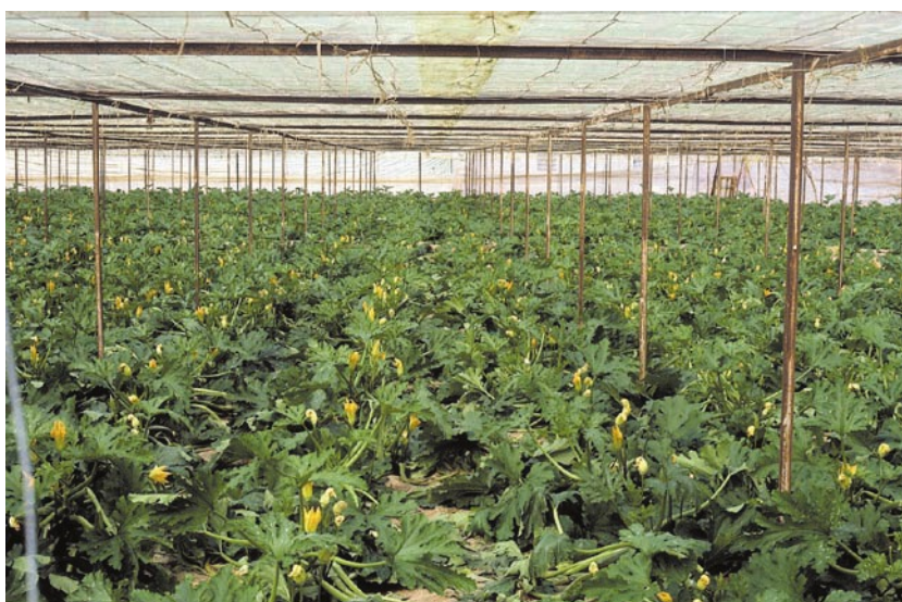
Photo 14.4. Conventional flat-roofed low-cost parral-type greenhouse.
