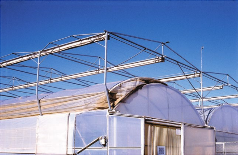
Photo 8.6. External shading device located over the greenhouse. The vents have anti-insect screens.
