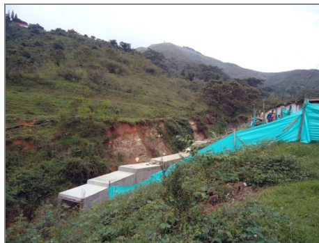
Fig. 12. Civil works on a natural environment
