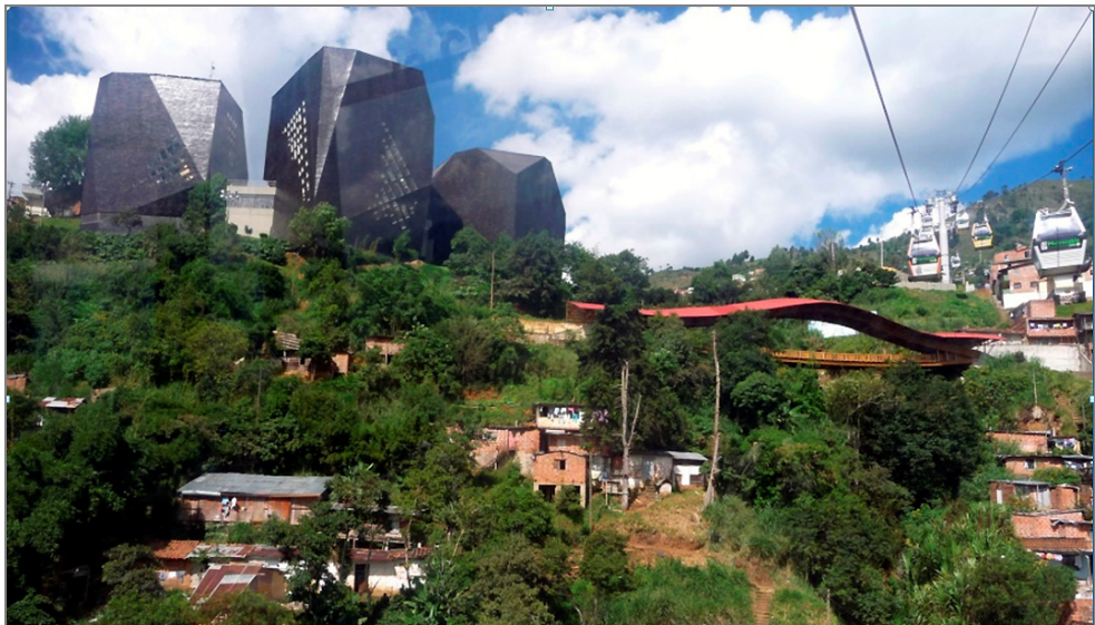
Fig. 9. España Library, Metrocable transport system, the bamboo bridge. Three of the many works recently developed as part of the program "social -urbanism", developed in the east side slope of Medellín.
