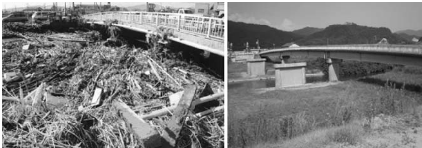
Fig. 2. Photos Showing Floating Debris from Nearby Mountains and Forests that Blocked Rivers and Damaged Bridges on the Left, and Well-Maintained Rivers and Embankments on the Right.
