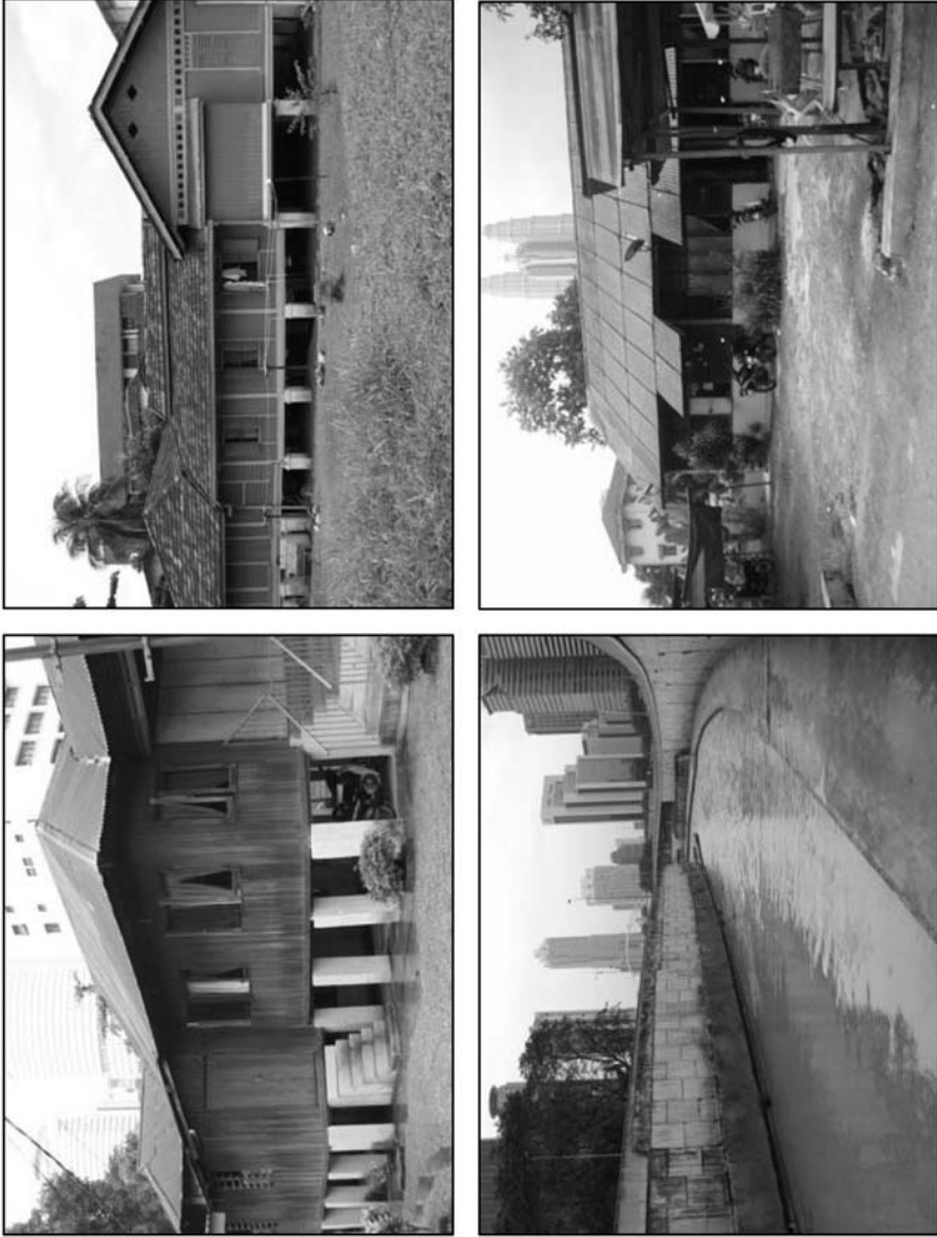
Fig. 3. Overview of Kampong Bahru. Top (Left and Right): Traditional Malaya Construction with Elevated Floor to Cope with Flood Risk in the Areas. Bottom (Left): River Passing through Kampong Bahru; (Right): Traditional Shops with a View of Twin Tower of Kuala Lumpur.
