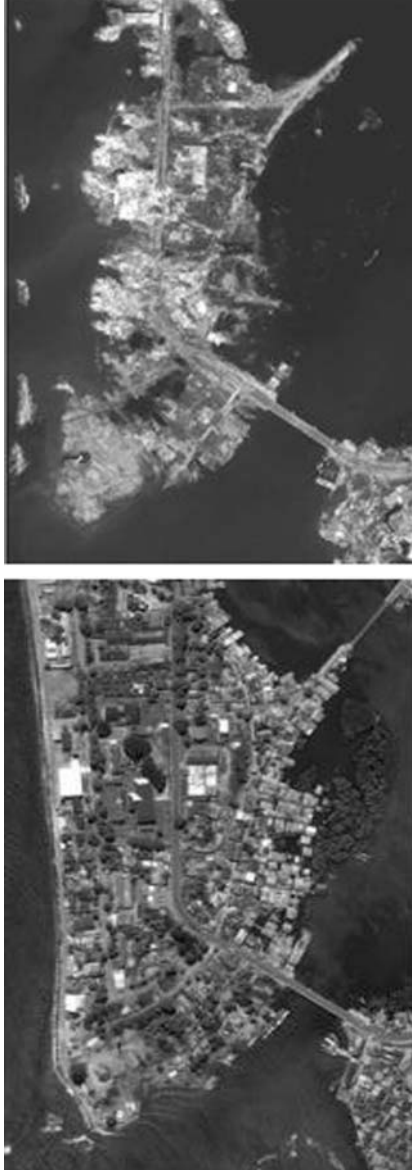
Fig. 2. Damage in Aceh Before and After the Disaster.
