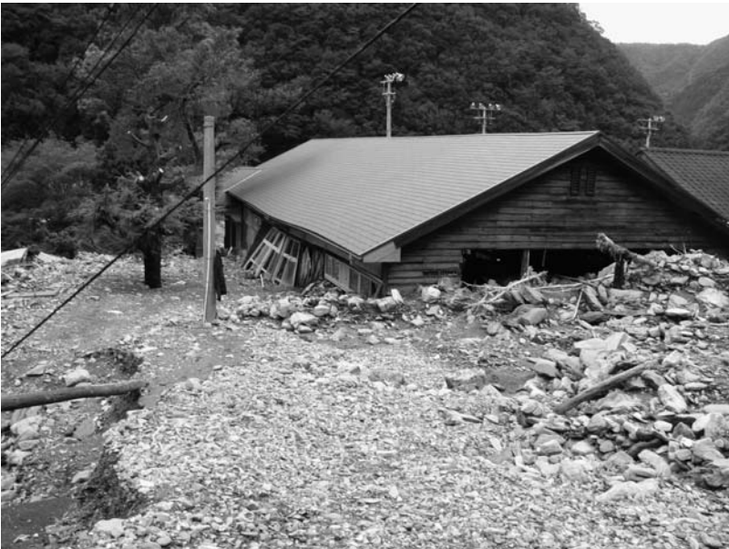
Fig. 4. Buried Shelter in Ofuki Area.
