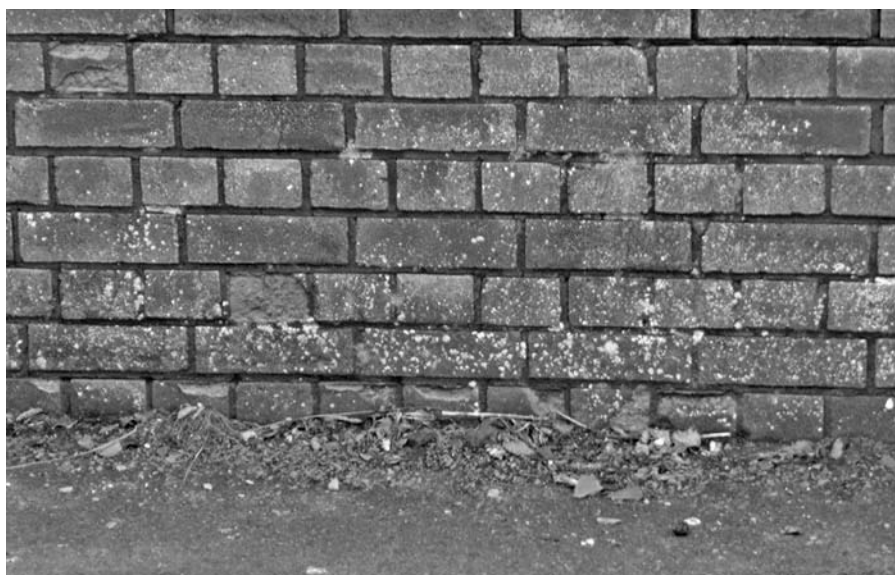
Figure 4.1. Example brickwork of a freestanding wall
