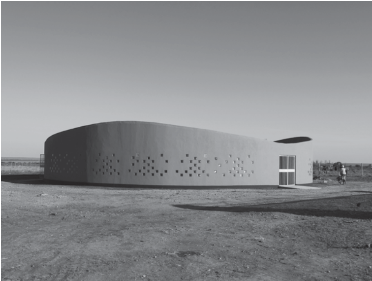
Fig. 12.19 Waterbank Girls Dormitory: a protected compound around a triangular garden courtyard
