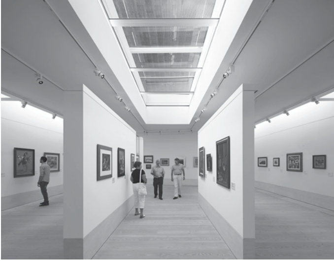
Fig. 6.23 The galleries are day-lit from the rooflights; sunlight is controlled with mid-pane louvres and retractable blinds
