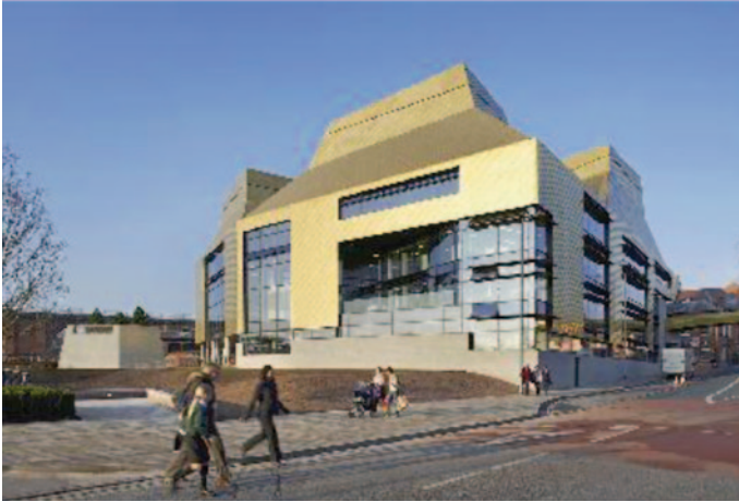
Fig. 6.16 Brise-soleils to the south elevation provide shading and help with control of road noise. The west elevation has solar control glass. (Hufton and Crow)
