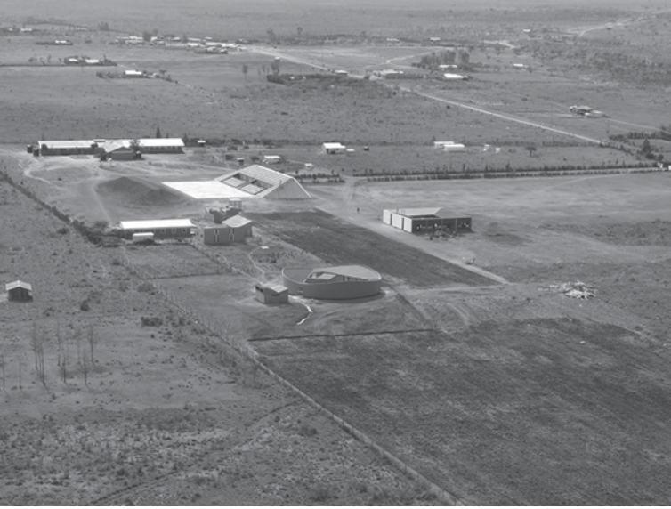
Fig. 12.14 The Waterbank Campus, aerial view showing the three principle structures: the stadium, canteen and girl's dormitory and secondary buildings, the boys dormitory, staff housing and latrines
