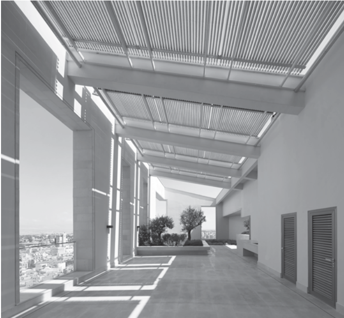
Fig. 6.25 Solar-thermal panels provide hot water to the building and shading to the roof terrace
