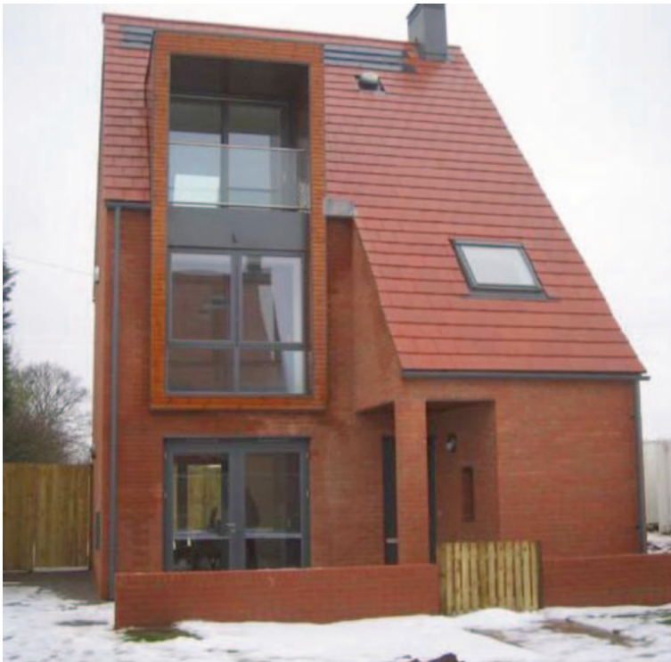
Fig. 8.6 One of the two prototype dwellings constructed at Temple Avenue. (Image by Leeds Beckett University)
