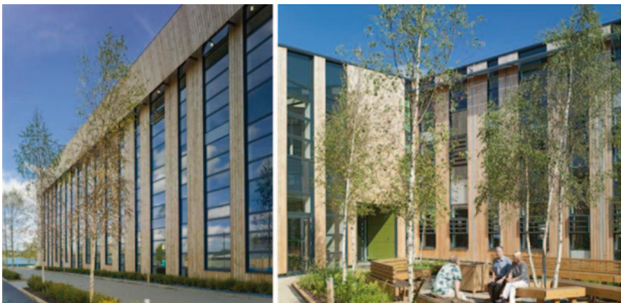
Fig. 6.8 a Large vertical panels of glazing to the north elevation with the external timber baffle to the window openings at roof level. b South elevation courtyard with external shading to the windows. (Peter Cook?)
