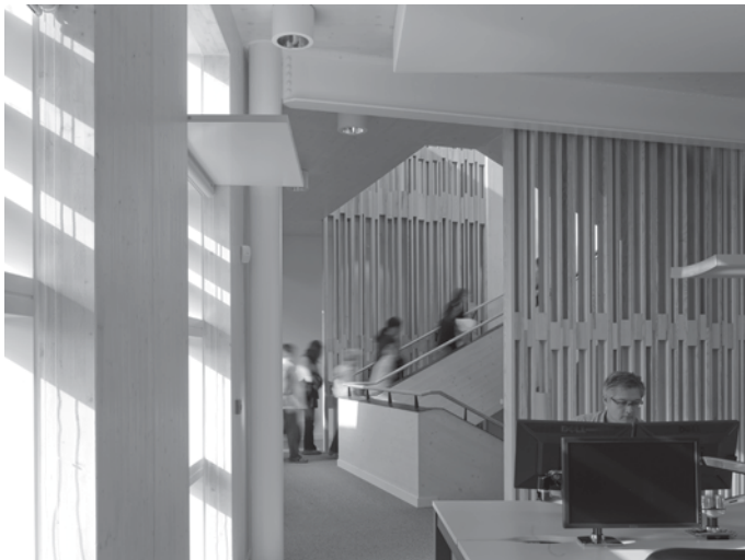
Fig. 6.11 External louvres and internal lightshelves to the south elevation help to control and improve the quality of daylight. (Peter Cook)
