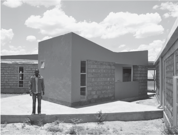
Fig. 12.20 The Matron's House in the dormitory courtyard on top of the underground water storage tank
