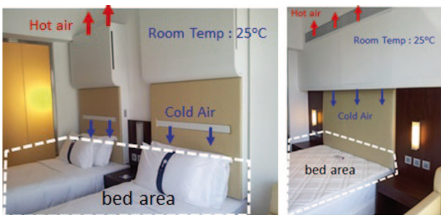
Fig. 7.10 Principle of operation of the Peltier headboard
