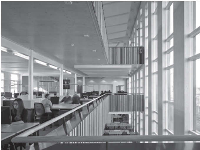
Fig. 6.14 The void allows air to rise to roof level and helps daylight to penetrate deeper into the floorplates. Wall-washing lights up the end walls. (Peter Cook)
