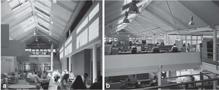
Fig. 6.6 a Sunlight is allowed to enter the main atrium to animate the space. b The office is well day-lit, but note the dark perimeter wall
