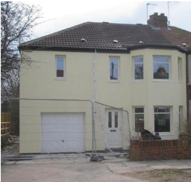
Fig. 8.13 Image of Temple Avenue retrofit property, post-retrofit. (Image by Leeds Beckett University)
