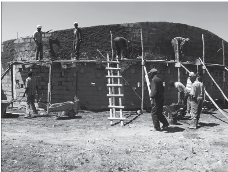
Fig. 12.16 The Waterbank Girls Dormitory under construction
