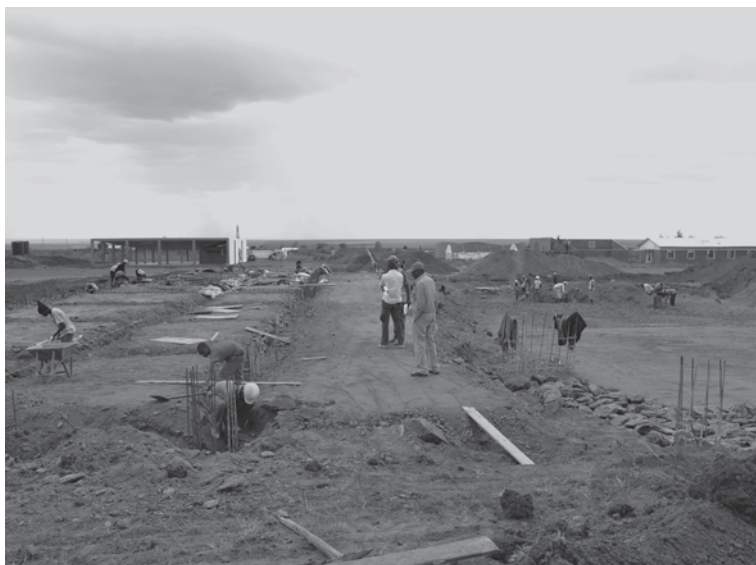
Fig. 12.13 The Waterbank Campus at the Endana Secondary School under construction
