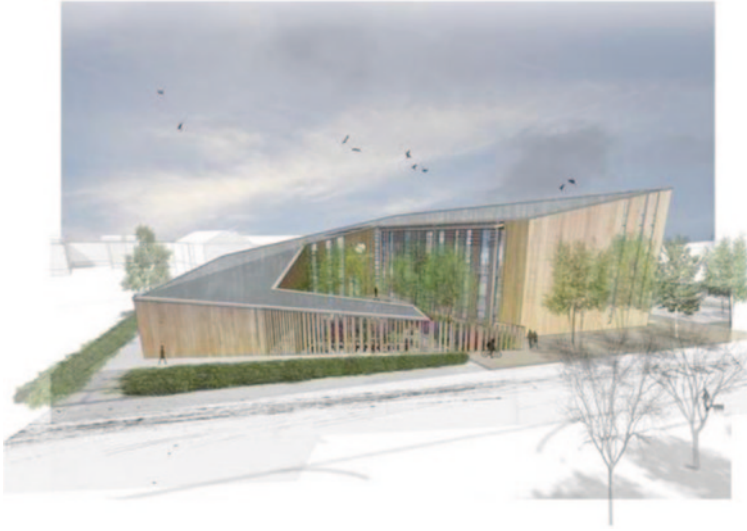
Fig. 6.9 Sketch showing like-building form and the south-facing sloping roof which could take future PVs. (FCB Studios)
