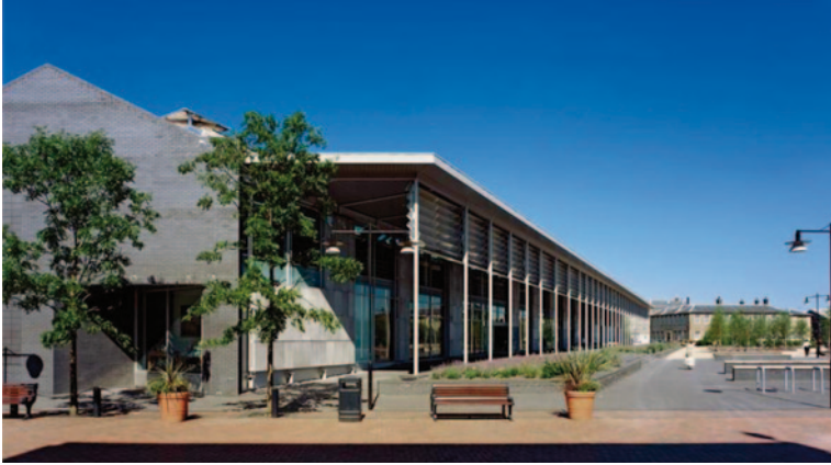
Fig. 6.1 The colonnade provides shading to the south façade
