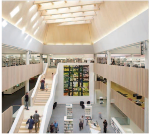
Fig. 6.19 Daylight is controlled by the structural timber baffles. Acoustic panels to the balustrades and bottom of the cones provide a good acoustic environment. Lights are hidden behind the acoustic panels. (Hufton and Crow)
