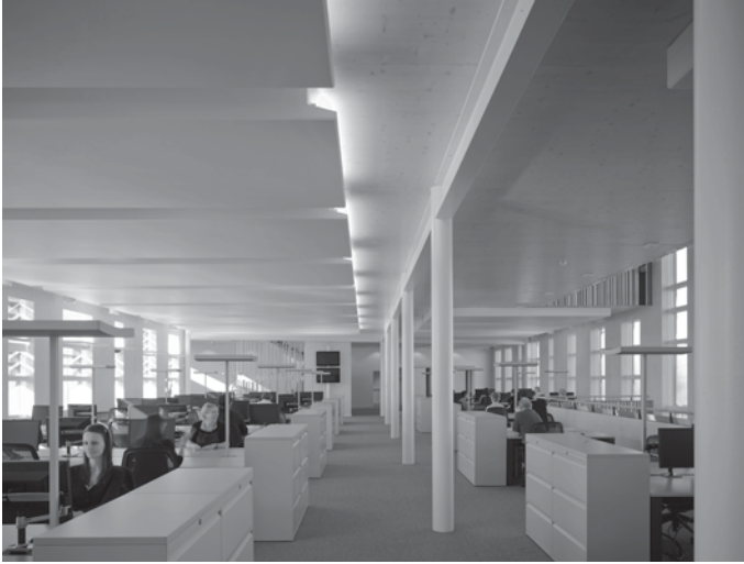
Fig. 6.12 The office floorplate has very good daylighting levels and artificial lighting to the circulation routes. The concrete radiators are painted white to help with daylighting. (Peter Cook)
