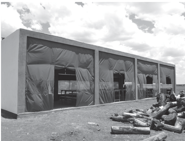
Fig. 12.17 The Waterbank Canteen with removable fabric walls used in the rainy seasons
