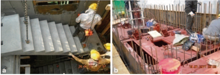
Fig. 7.4 a Precast staircase. b Metal formwork
