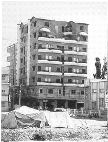
Figure 9 High rise RCC structure close to the epicenter but not damaged
