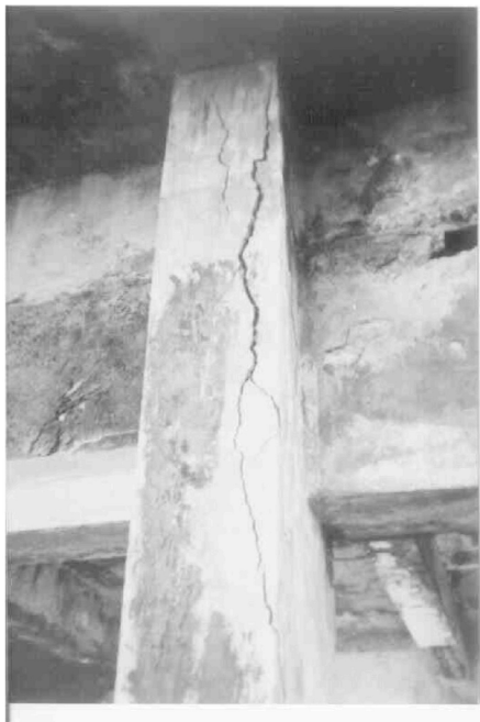
(i) Crack in column
