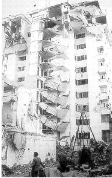
Figure 1 Building collapsed due to construction of swimming pool on the terrace besides other reasons
