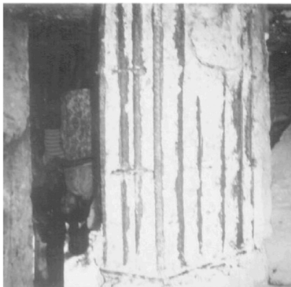
(iii) Spalling in column
