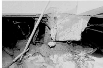
Figure 7 Shear failure of a column causing a soft storey collapse
