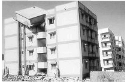
Figure 2 Dislodging of weakly connected overhead water tank
