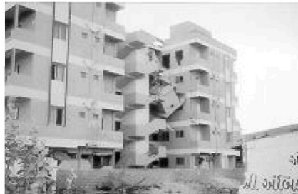
Figure 3 Dislodging of weakly connected lift machine room
