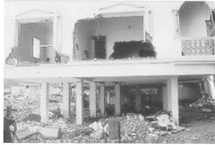
Figure 8 Large cantilever beams projecting outside the columns on the ground floor
