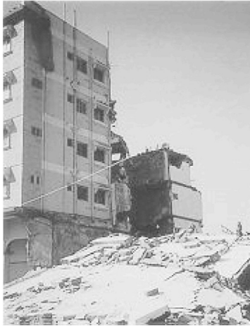
Figure 10 Three structures at same location - one totally collapsed, one badly damaged and one slightly damaged
