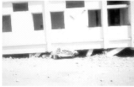
Figure 6 Weak column connections resulting in total collapse of the entire storey
