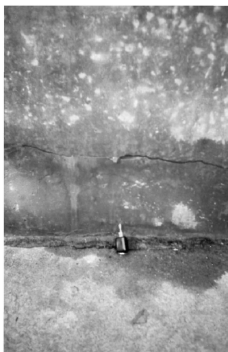
Figure 3 Cracking to wall elevation
