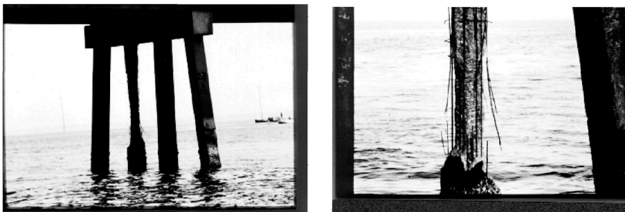
Figure 1 Four piling bent of the Bryant Patten Bridges. A jacket was removed from the second pile from the left revealing major cross section loss
