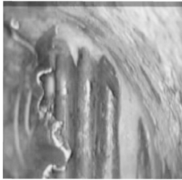
Figure 5 Still image showing tendons and grout
