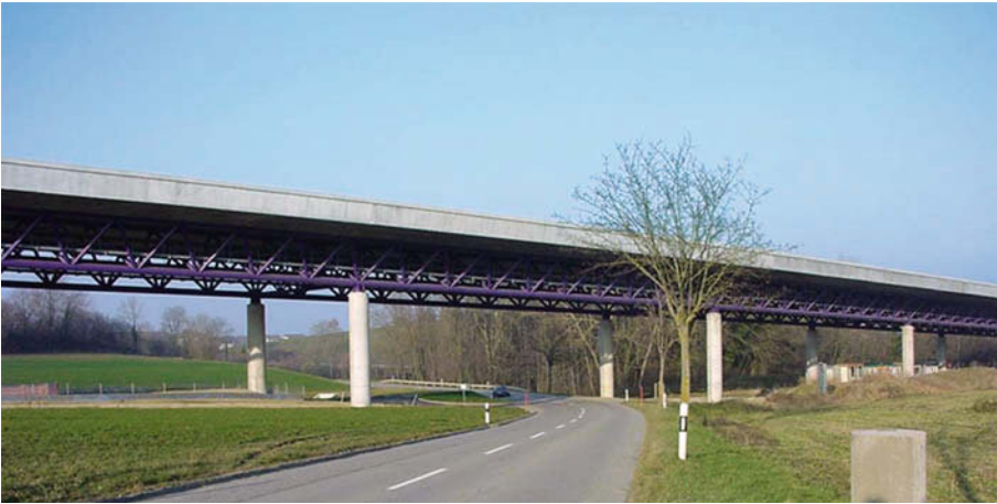
Fig. 3.19 Viaduc de Lully (CH). Engineer Hans-G. Dauner (Photo ICOM)
