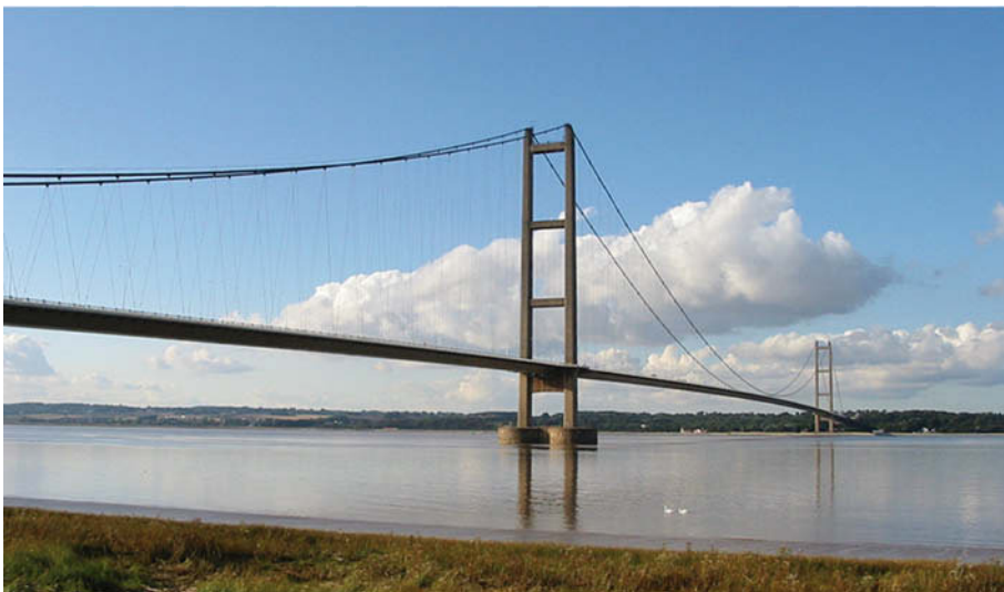
Fig. 3.12 Humber Bridge (UK). Engineers Gilbert Roberts and Bill Harvey (Photo ICOM).
