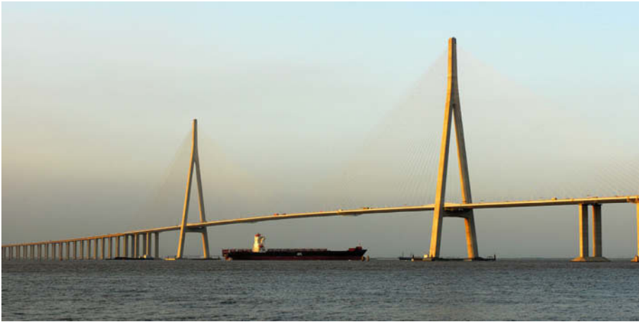
Fig. 3.21 Sutong Bridge (PRC). Engineer Jiangsu Provincial Communications Planning and Design Institute (Photo Yaojun Ge).
