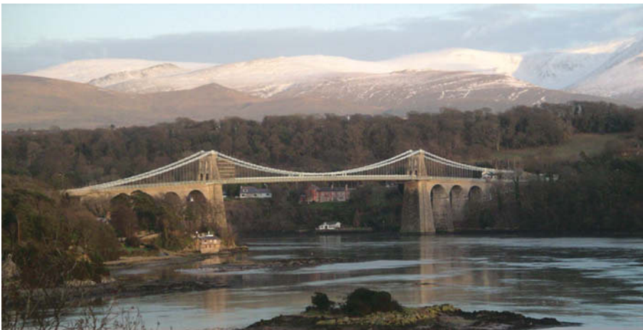
Fig. 3.1 Menai Straits Bridge (UK). Engineer Thomas Telford (Photo Mike Knapton).
