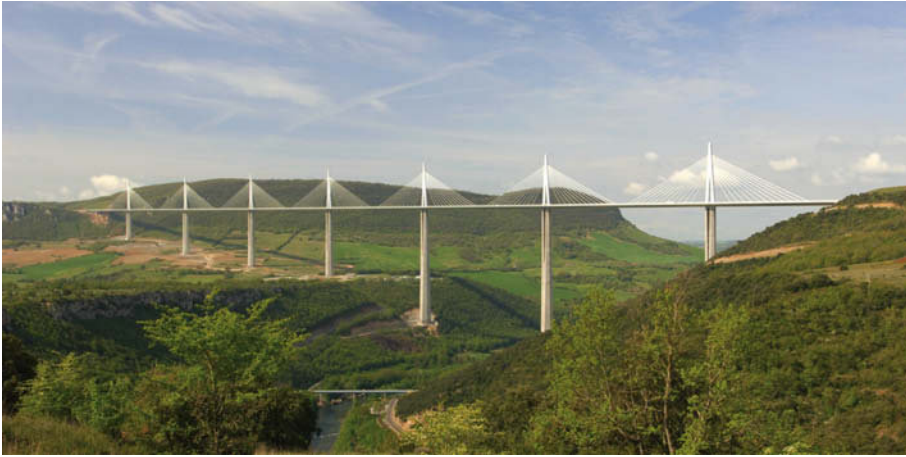
Fig. 3.17 Viaduc de Millau (F). Engineer Michel Virlogeux (Photo Daniel Jamme).
