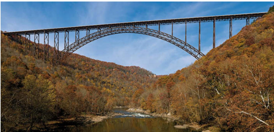
Fig. 3.14 New River Gorge Bridge (USA). Engineer Clarence V. Knudsen (Photo Jason Galloway).
