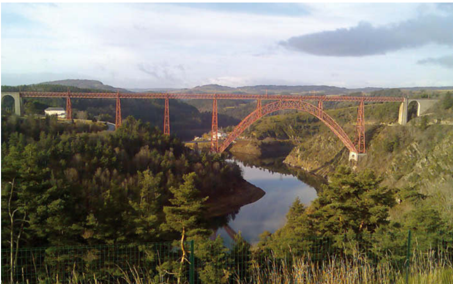
Fig. 3.6 Viaduc de Garabit (F). Engineers Maurice Koechlin and Léon Boyer (Photo ICOM).
