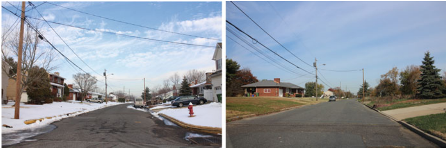
Fig. 6.5 A street in Sayerville, NJ, before buyouts in December 2013 ( left ) and after demolitions in December 2014 ( right )
