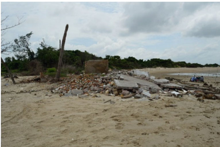
Fig. 19.4 A house collapsed due to beach erosion
