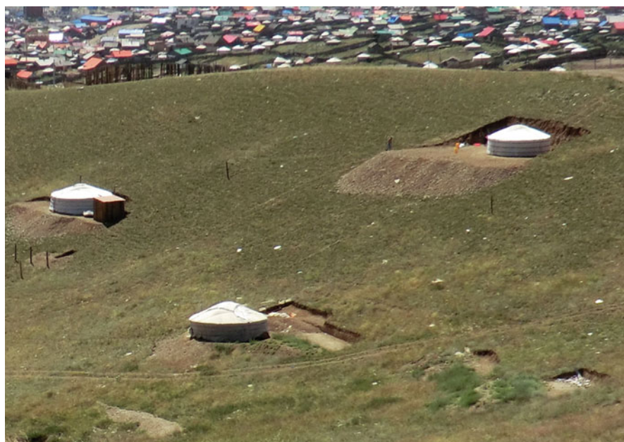
Fig. 8.5 Gers construction on steep slopes by digging and developing lands (Photo by Saizen in August 2011)
