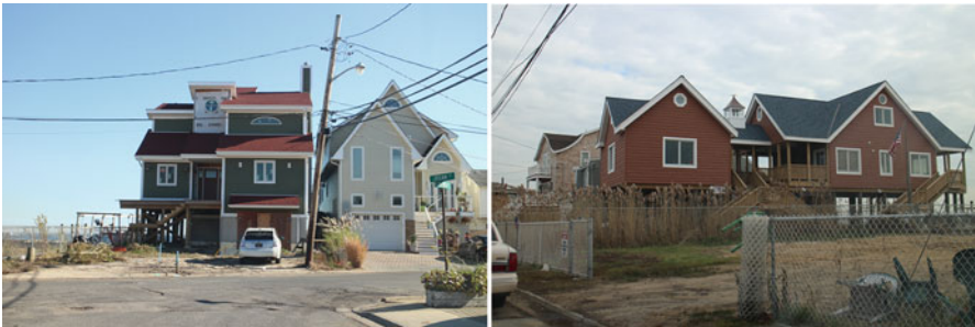
Fig. 6.3 Examples of large new houses built on lots eligible for buyouts
