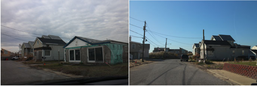
Fig. 6.2 Area in Lindenhurst, NJ, eligible for buyouts, such as the house in the foreground in December 2014 ( left ), already demolished in November 2015 ( right )
