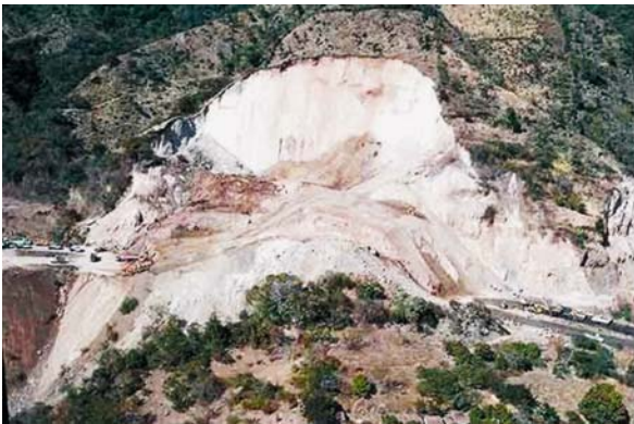
Fig. 41.3. The Pan America Highway in El Salvador was badly damaged by a landslide during the January 2001 earthquake
