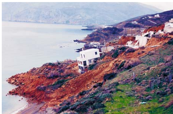
Fig. 37.8. Rotational slide in the fine neo-gene sediments in Skiros Island, triggered by heavy rainfalls
