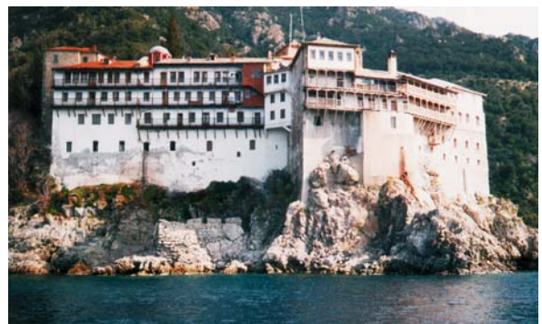
Fig. 30.4. Southern part of St. Gregory Monastery
