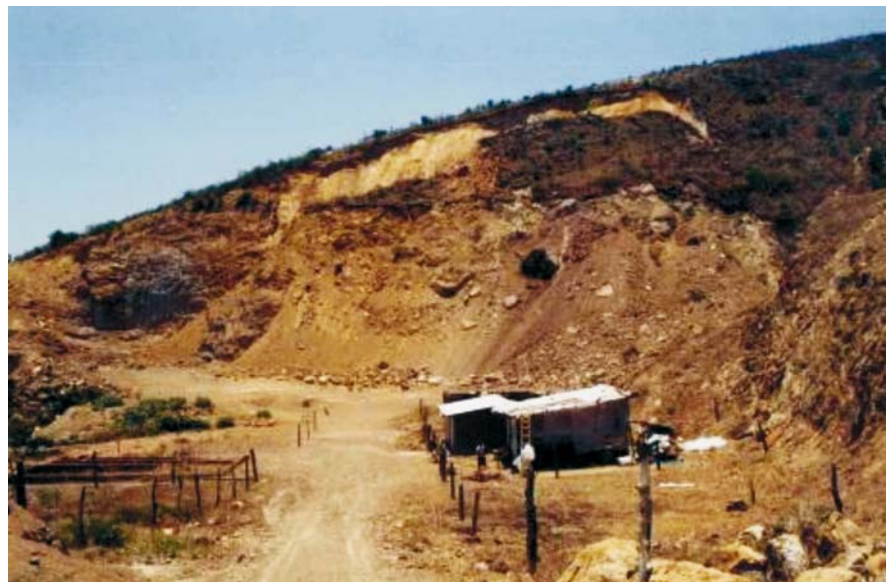
Fig. 34.2. A view of Ajuterique-Playón landslide that involving rocks of Yojoa Group. In second plan, the mass mobilized by one of the last acceleration episodes
