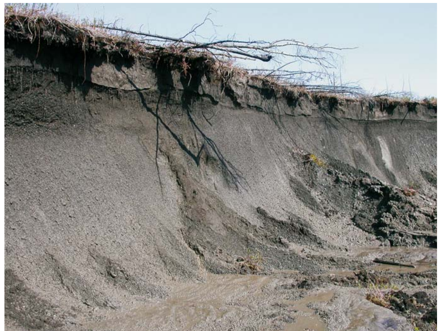
Fig. 25.5. Head scarp of a retrogressive landslide
