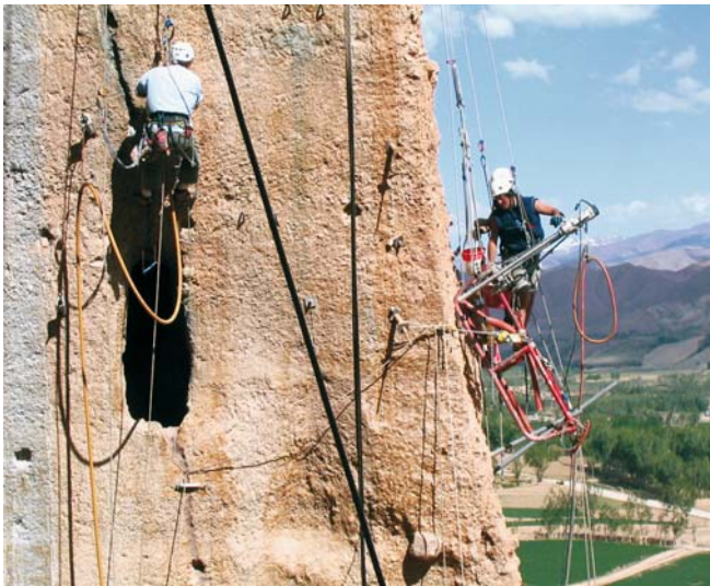
Fig. 8.5. Final consolidation with the use of professional climbers
