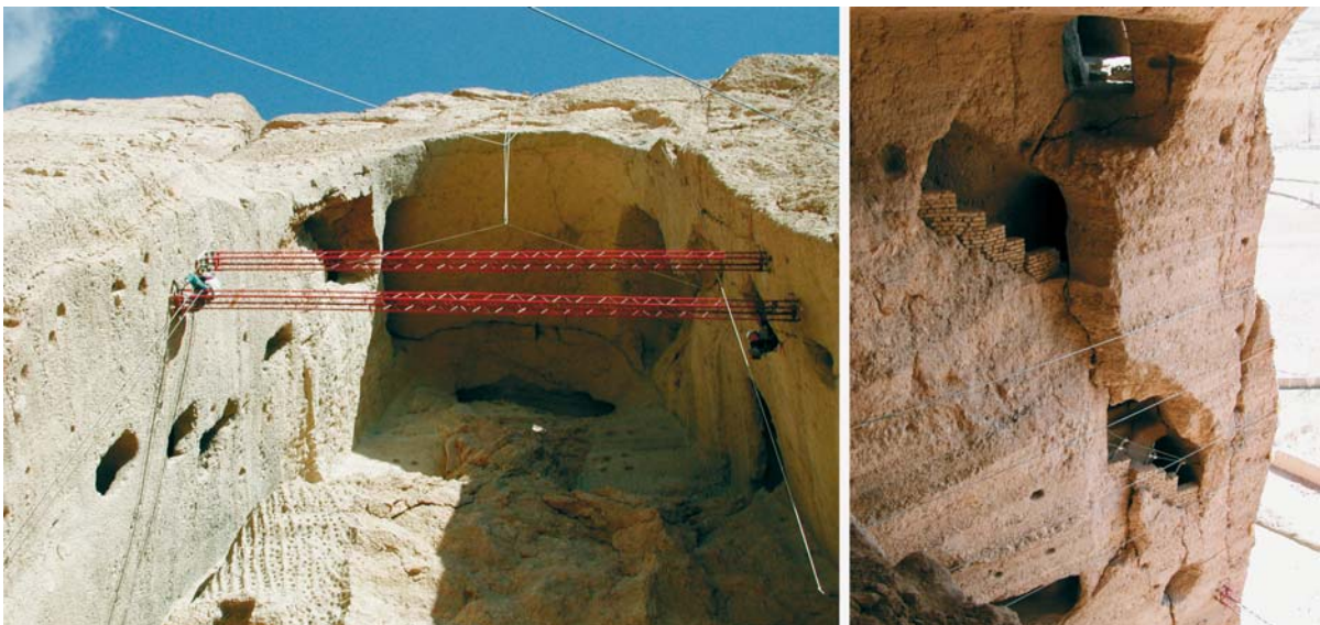
Fig. 8.4. The beam (left) and steel rope (right) for the temporary support of upper Eastern part of small Buddha
