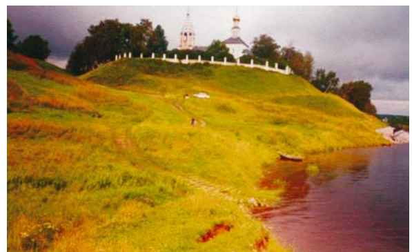
Fig. 46.5. The Blessed Virgin Church (fifteenth century, the village of Gorodnya) located on the remnant of a high slope affected by landslide process
