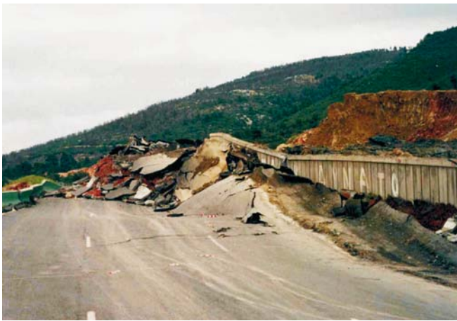
Fig. 37.6. Malakasa landslide, February 1995. Damages on the new highway from Athens to Thessaloniki. The landslide manifested in the tectonized and weathered zone of schists covered by debris
