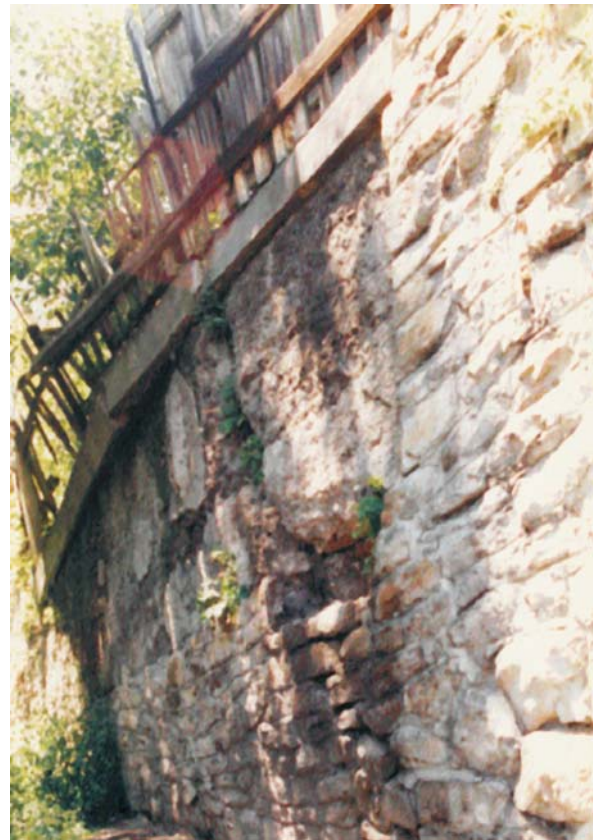
Fig. 45.4. Earth pressure on a retaining wall
