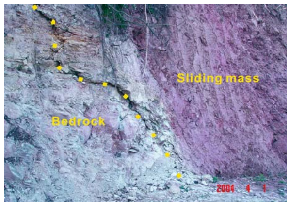
Fig. 40.4. Crack at the right boundary of block 1 outcropped at a roadside
