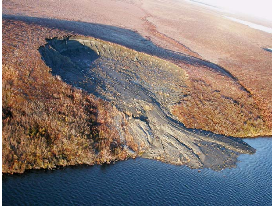
Fig. 25.4. A typical deep retrogressive failure
