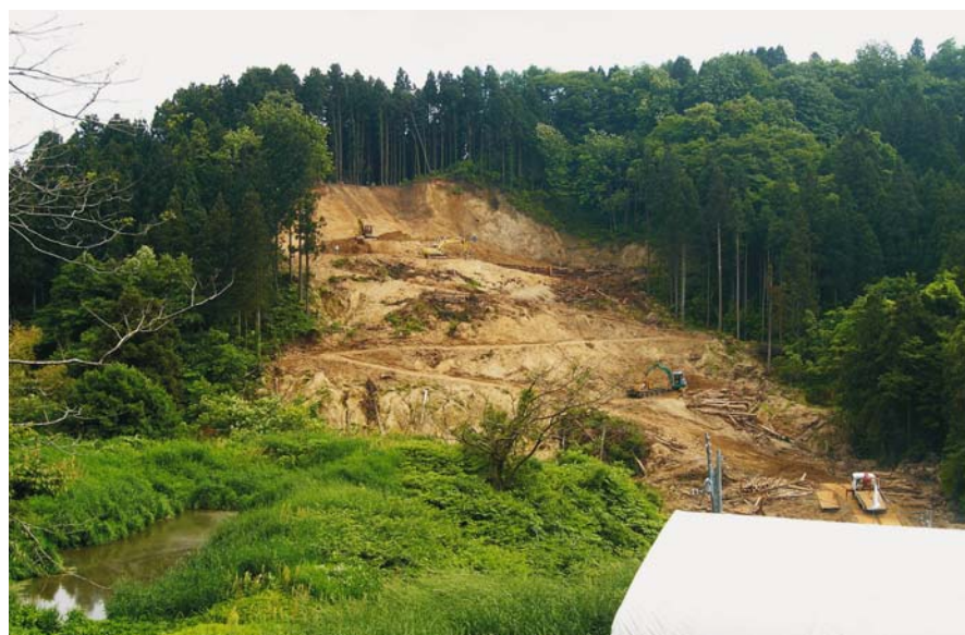
Fig. 16.1. Site of rainfall-induced landslide at Sakashi-dani in Niigata, Japan, in 2004
