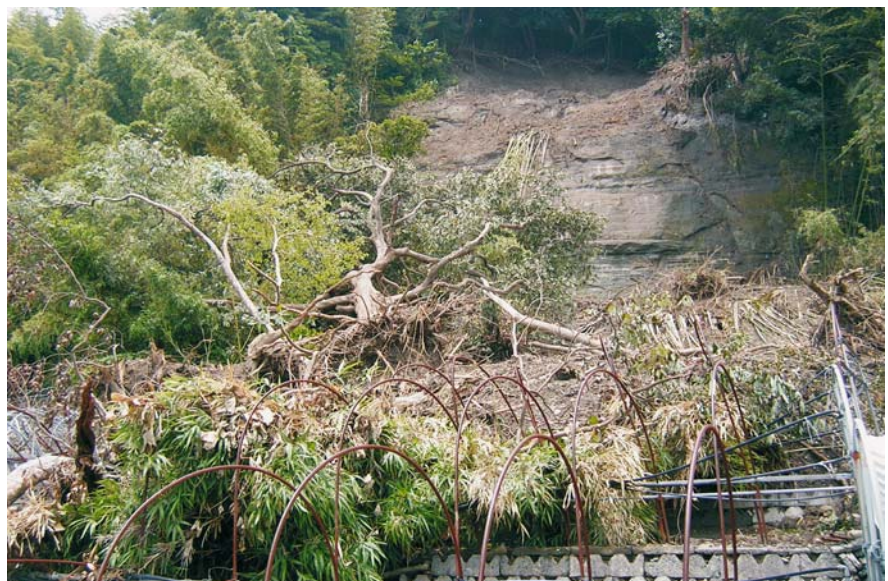
Fig. 16.3. Small slope failure in Shizuoka, Japan, in 2004
