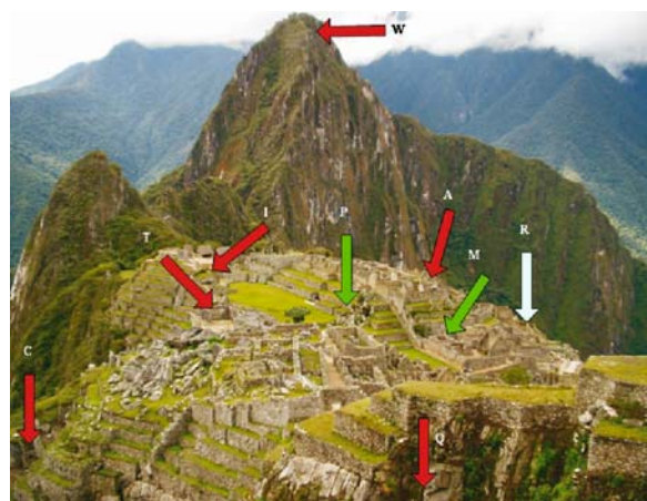
Fig. 4.1. Photo of Machu Picchu archaeological site with localization of dilatometric measurements. C: Cave (measuring site C1); T: Principal Temple (T1, T2, T3); I: Intiwatana (I1, I2, I3); P: Plaza (P1); W: Huayna Picchu (W1, W2, W3); A: Acclawasi (A1); M: Wairana o Mirador (M1, M2, M3, M4); R: Rodadero (R1, R2, R3); Q: Qhata (Q1). Qualitative evaluation of trends of movements. Red color: irreversible movements; green color: without any irreversible movements; light blue: cannot be still interpreted
