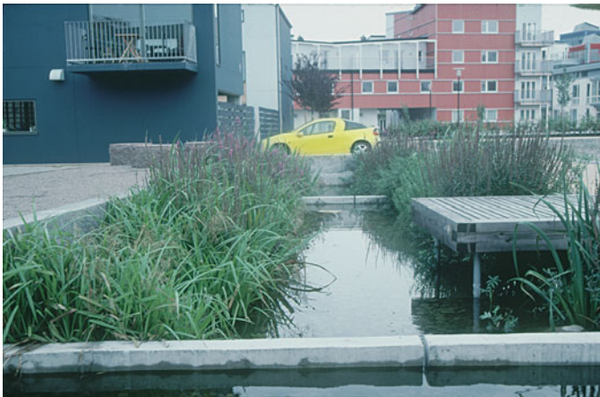
Fig. 15.13 Local infiltration of rainwater is, as well as green roofs, important elements in the ecological concept of the Western Harbour area in Malmö (Photo: Kjell Nilsson)
