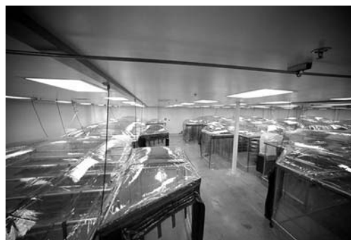
Fig. 34-2 Multiple HEPA-filtered mass air displacement flexible film “rooms” inside a large room.
