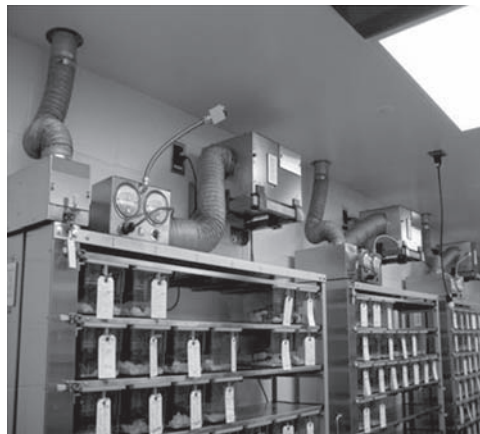
Fig. 20-16 Schematic and photograph of an individually ventilated cage rack of the room supply, direct exhaust type. In the system shown, exhaust is provided by the building's system and therefore, no rack exhaust blower is provided. Exhaust stability is ensured with the use of a PICV. Schematic courtesy of Phoenix Corporation, Inc.
