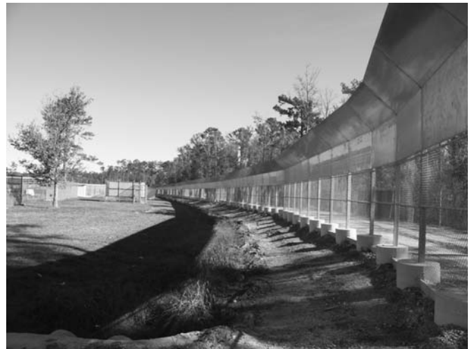
Fig. 21-11 Unscalable perimeter fence.
