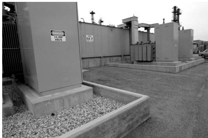
Fig. 14-1 Electrical substations have been raised by placing them on concrete slabs and surrounding them with concrete curbs to protect them from flood damage.
