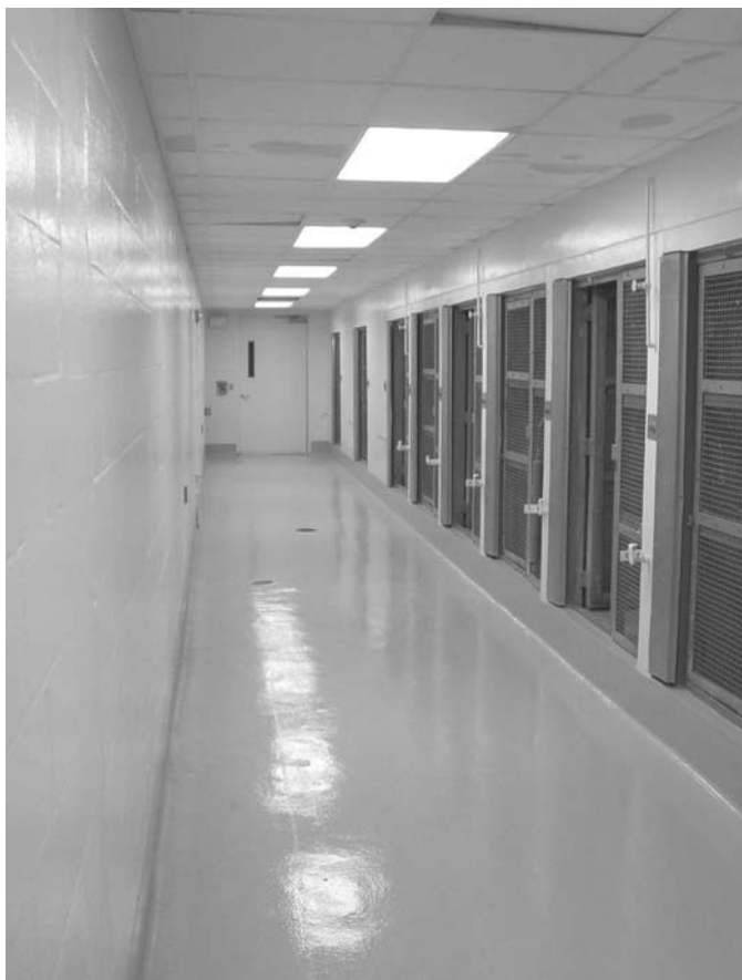
Fig. 21-8 Indoor view of indoor/outdoor runs.
