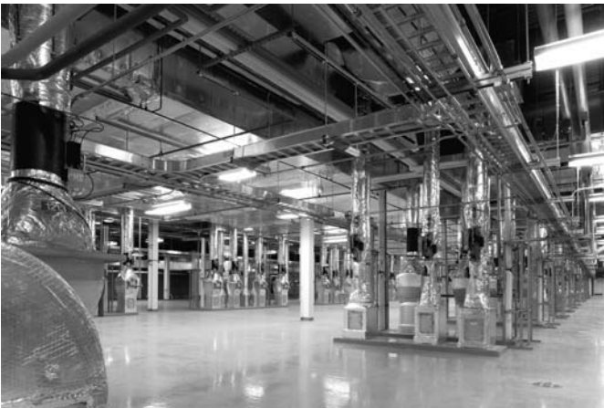
Fig. 4-19 Interstitial space provides access for adjustment of HVAC equipment.
