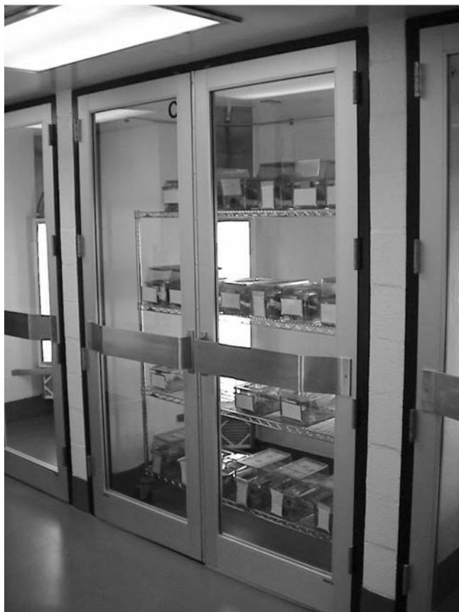
Fig. 15-4 Small animal cubicle with hinged doors and vertical mounted fluorescent lights in back corners.
