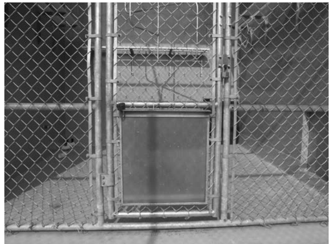
Fig. 21-17 External door to run with chute port.
