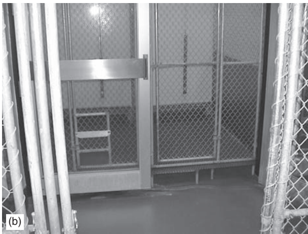
Fig. 15-16 Cubicles with fixed raised floors: (a) two adjacent large animal cubicle pens with different types of raised floors, fiberglass T-bar slats and vinyl-coated expanded metal; (b) raised vinyl-coated expanded metal floor showing a stainless-steel leg of the stainless-steel frame that supports the raised floor.
