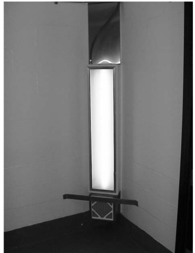
Fig. 15-9 Back corner of small animal cubicle showing a triangular air duct (in this case an exhaust duct with a filter, but it could be designed as a supply air duct) extending from the ceiling to the floor with a fluorescent light fixture mounted on it.
