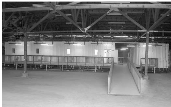
Fig. 16-3 Modular rodent housing buildings installed in a warehouse.
