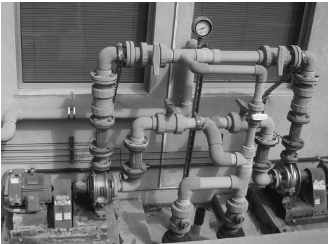
Fig. 23-5 Pump station located outside of the building but next to an office window. Several years after installation, this pump became a source of vibrations and harsh noise in the adjacent office space.
