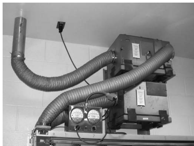
Fig. 20-11 Wall-mounted supply and exhaust blowers. The exhaust blower is directly connected to the building's exhaust system.
