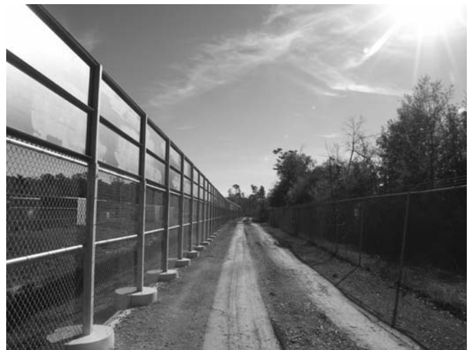
Fig. 21-12 Perimeter security road.
