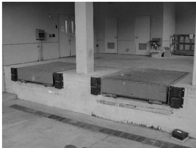
Fig. 12-3 Loading dock with dual hydraulic lifts allowing for more than one vehicle to access the dock simultaneously.
