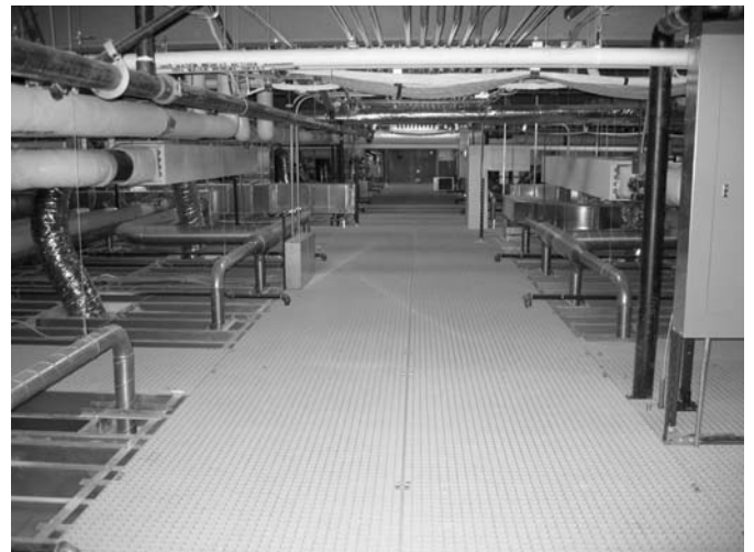
Fig. 13-3 Example of partial interstitial space with walkways (Washington University School of Medicine, St Louis, Missouri).
