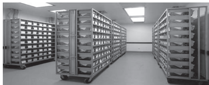
Fig. 20-12 Schematic and photograph of individually ventilated cage racks of the direct supply, direct exhaust type. PICVs (two per rack) are located in interstitial space above.
