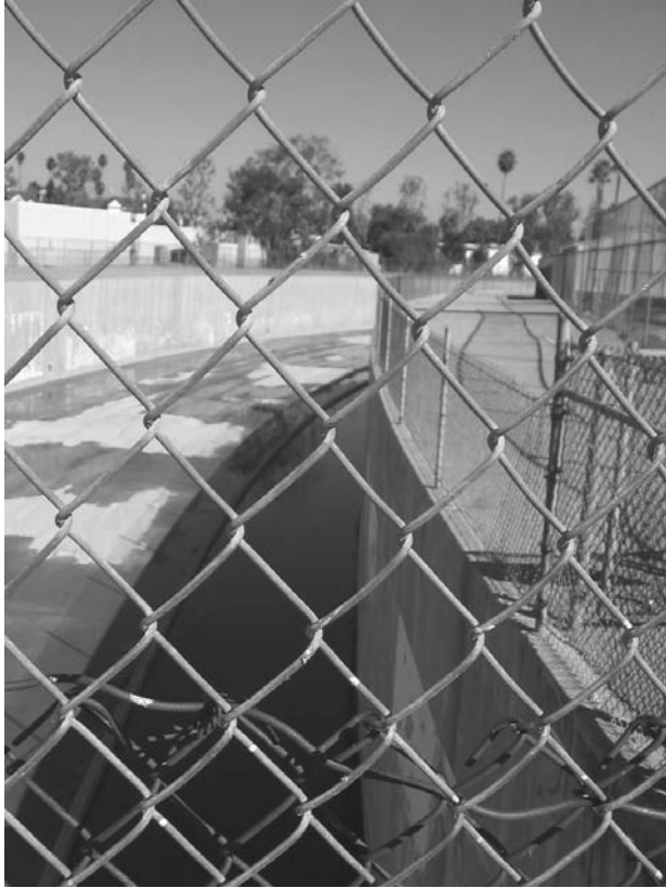
The Concrete Channel of the Los Angeles River. The Los Angeles River was once the primary water source for the Los Angeles basin, but frequent flooding led some to search for a solution to control the unpredictable river flows. Since the late 1930s, the river has been primarily a flood control channel. Environmentalists and others hope that the river can soon be returned to its more natural state. PHOTO BY IRENE KLAVER.
