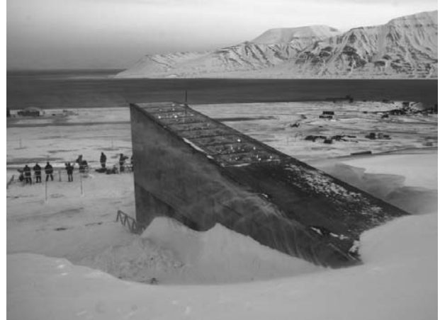
Doomsday Vault, Norway. The Svalbard Global Seed Vault, known as the “doomsday” vault, was officially opened in February 2008, to protect millions of food crops from climate change, wars, and natural disasters in the remote Arctic location. Several seed banks exist around the world, in order to protect against an accidental loss of genetic diversity. AP IMAGES.
