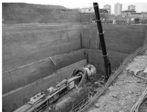
Figure 1. Soil Nail Retaining Wall and TBM Entering Tunnel.
