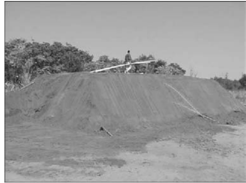
Figure 14. Trial slope embankment.
