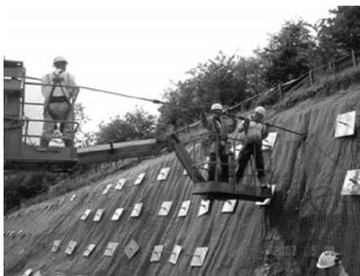
Figure 10. Instrumented nail installation.
