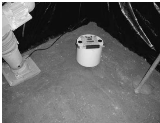
Figure 9. Manual compactor and GeoGauge equipment.
