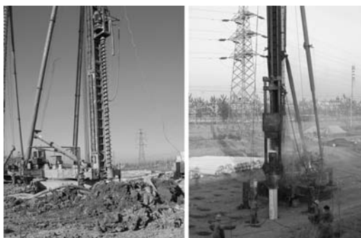
Figure 2. Continuous flight augers and centrifugally precast concrete driven piles.
