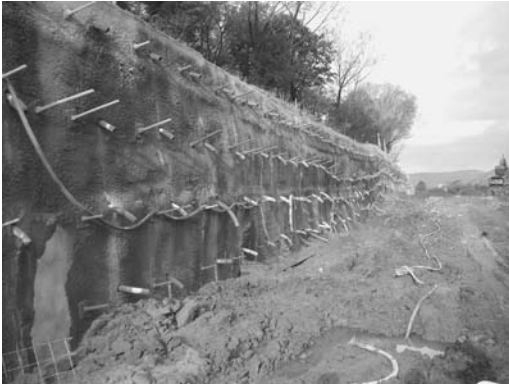
Figure 1. The photo of the cut with applied primary support system.
