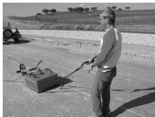
Figure 2. Partial view of the trial embankment with execution of a GPR profile.
