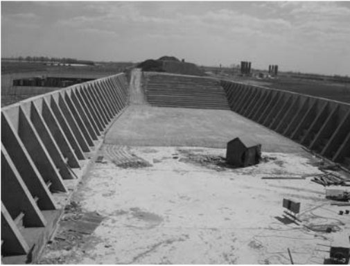
Figure 4. Construction of retaining walls.
