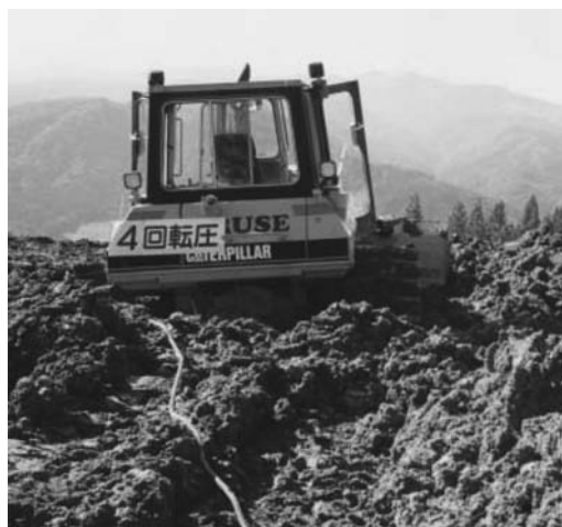
Figure 1. Decline of trafficability in poor soil ground (Shigematsu et al., 2001).
