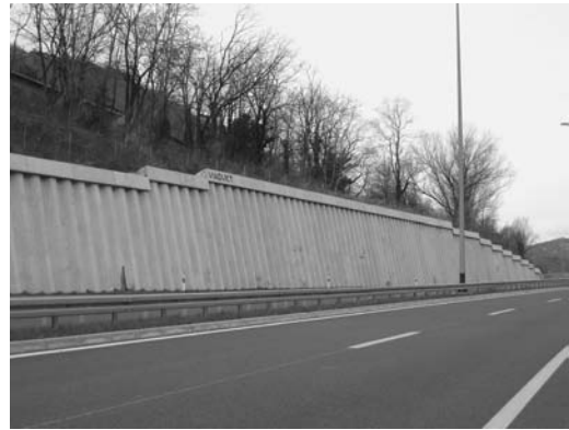
Figure 3. The photo of the cut with applied secondary support system.
