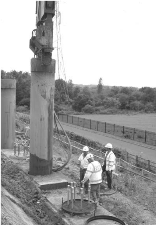
Figure 4. Constructing Retaining Wall Piles.
