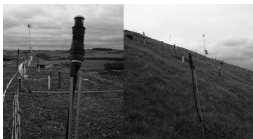
Figure 9. Rainfall sprinkler component of climate control system.
