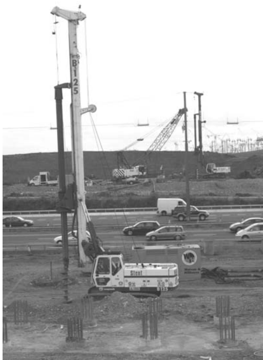
Figure 2. Piling Rig next to Live Motorway.
