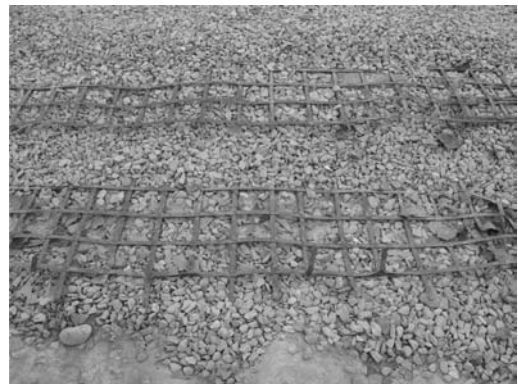
Figure 8. Embedded geogrid.
