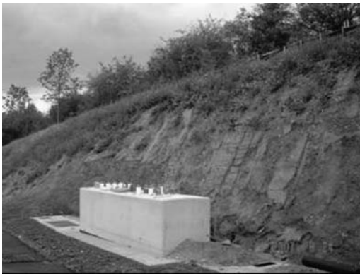
Figure 13. The nailed slope after covering by geocell and top soil.
