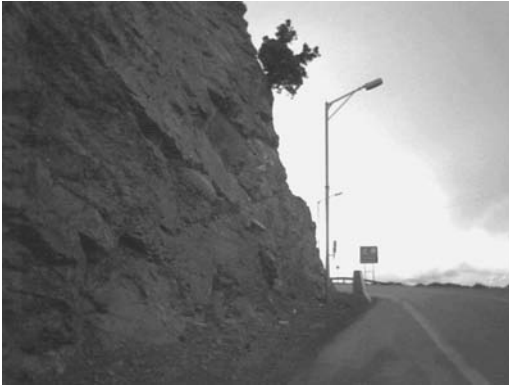
Figure 1. A photograph of the Khosh Yeylagh main road.
