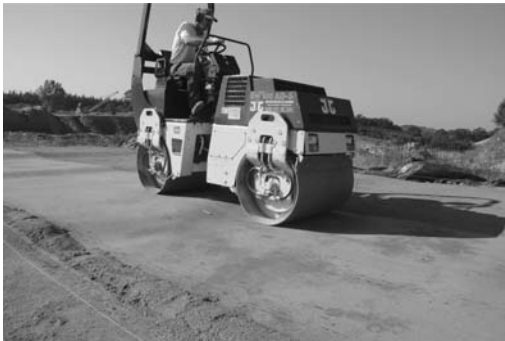
Figure 5. Roller compaction of Slotsgrus® at field test site. Photo: P. Kristoffersen, Forest & Landscape Denmark.
