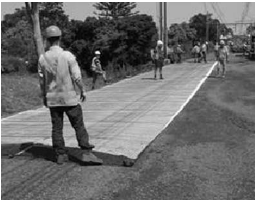
Figure 6. Installation of geogrids and geotextiles at Bulli site.
