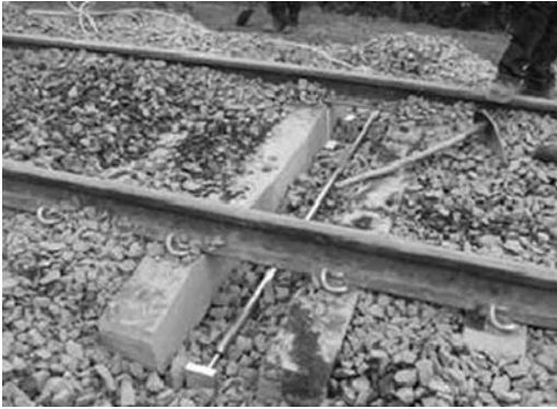
Figure 5. Installation of displacement transducers at Bulli site.
