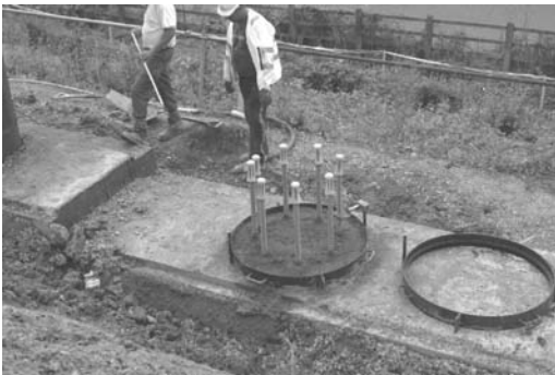
Figure 5. Use of Circular Former.
