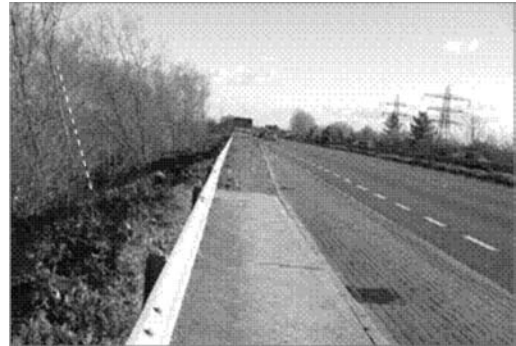
Figure 5. Photo taken for the embankment at Site-2, where Willow trees are leaning significantly.
