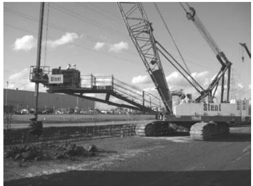
Figure 7. Piling Rig with Extended Frame.
