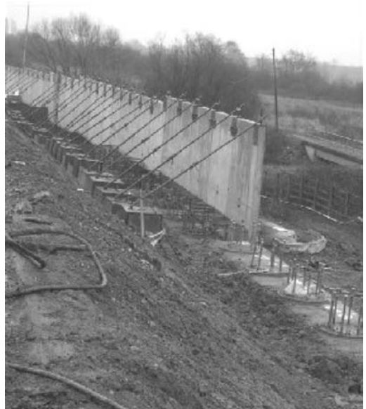
Figure 6. Precast Concrete Retaining Wall Units Being Positioned.
