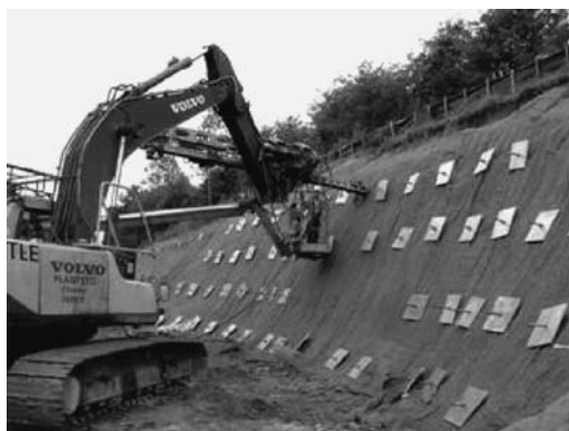
Figure 9. Drilling borehole.
