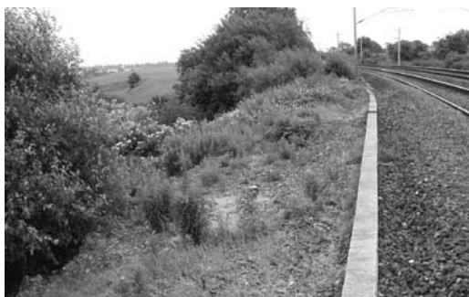
Figure 3. View southwards along Up-line slope.
