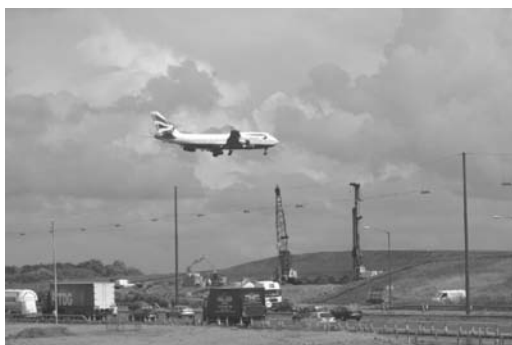
Figure 3. Piling Rig beneath Flight Path.
