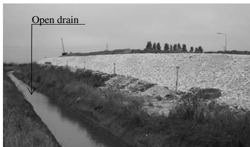
Figure 5. Final embankment height plus temporary surcharge in place (view westwards).
