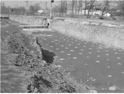
Figure 10. Situation before filling.
