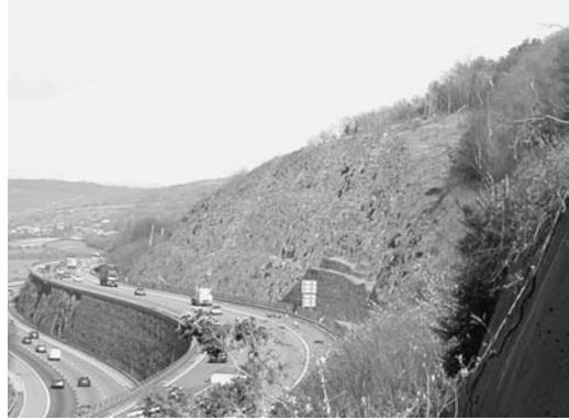
Figure 2. M5 Wynhol Viaduct rock slopes.
