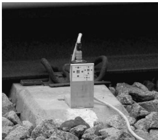
Figure 3. Instrumentation bracket attached to sleeper end showing PIV target with vertical geophone to the rear.
