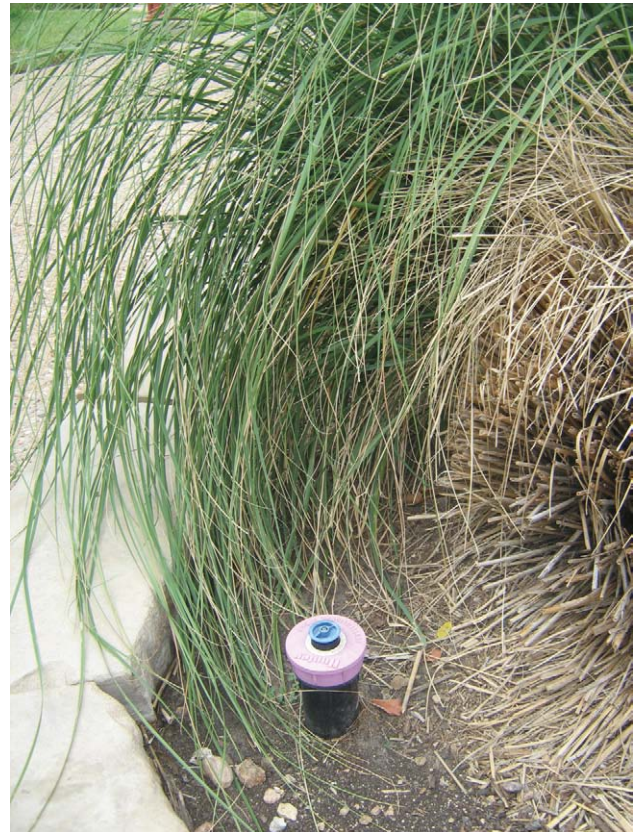
■ FIGURE 6.15 Purple irrigation equipment indicates reclaimed water use.
