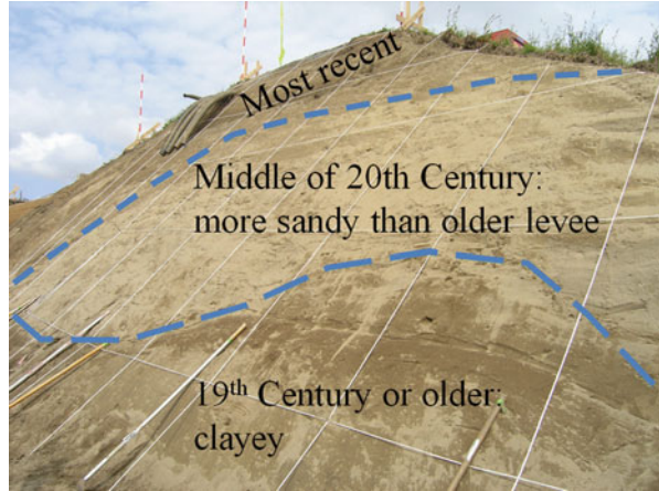
Fig. 6.21 Excavated cross section of Tone River levee at Iijima
