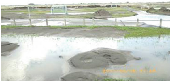
Fig. 6.4 Liquefaction and sand ejecta in front of the damaged levee in Sawara
