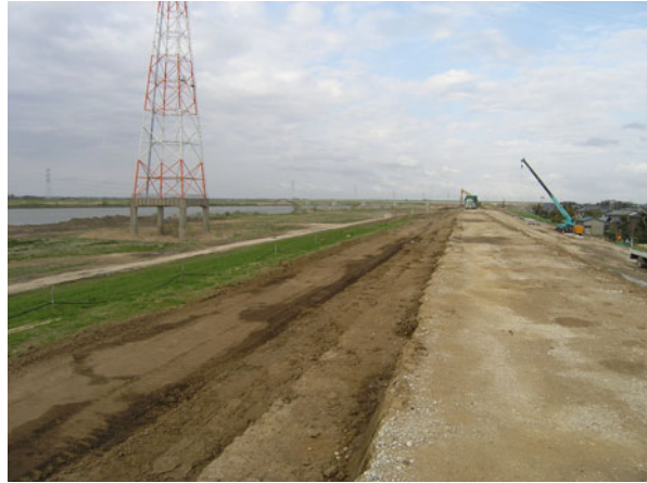
Fig. 6.19 River side of Tone River levee at Sakae without damage (entire restoration of the levee going on in April, 2012)
