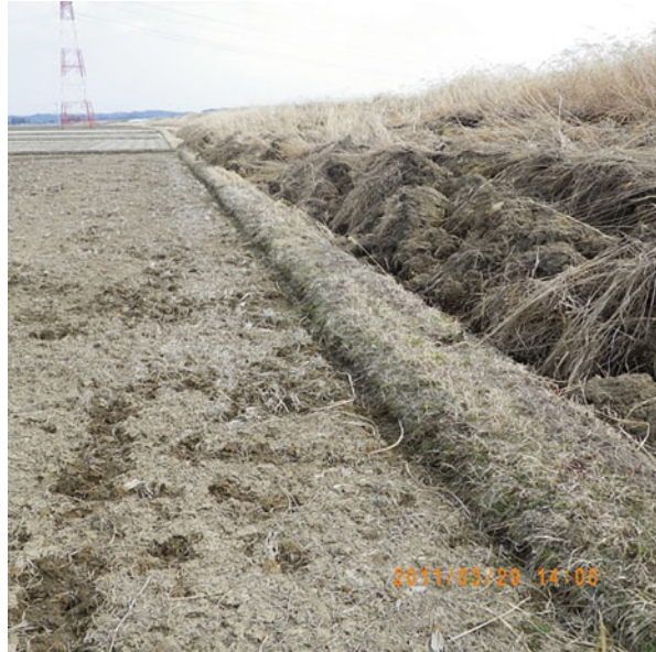
Fig. 6.30 Surface distortion of Naruse River levee with internal liquefaction (at Shimo Niida site)
