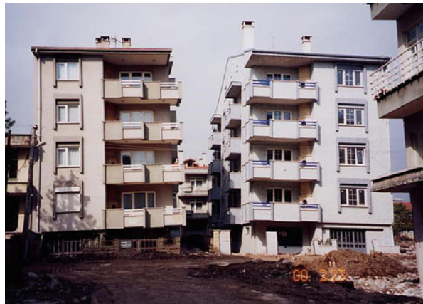
Fig. 5.14 Two buildings tilted away from each other in Adapazari City during the 1999 Kocaeli earthquake
