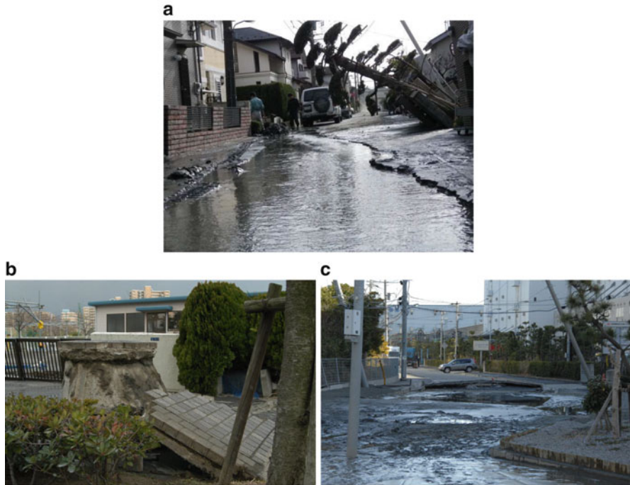
Fig. 4.22 Destruction of the ground due to liquefaction (Offered by Urayasu city office). (a) Ground devastation in a residential section. (b) Floating of sewage manhole. (c) Spreading of sand over the road
