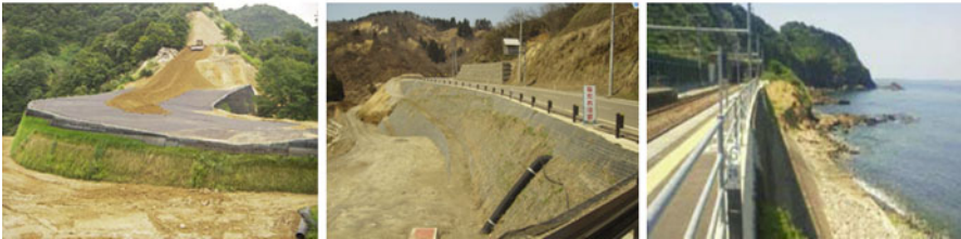
Fig. 12.4 Earthquake disaster rehabilitation by reinforced soil wall
