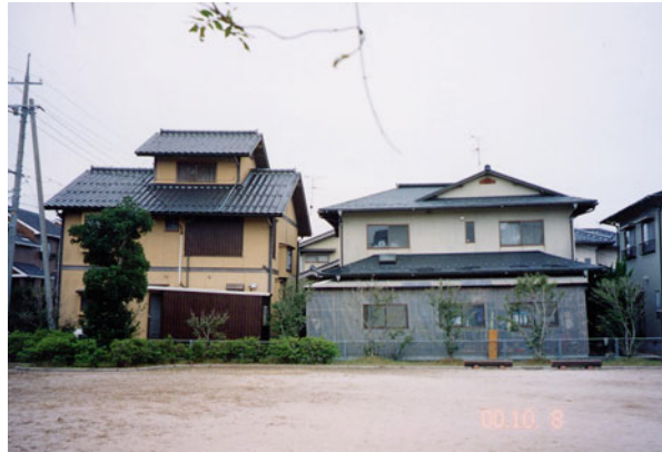
Fig. 5.13 Two houses tilted toward each other at Abehikona during the 2000 Tottoriken-seibu earthquake
