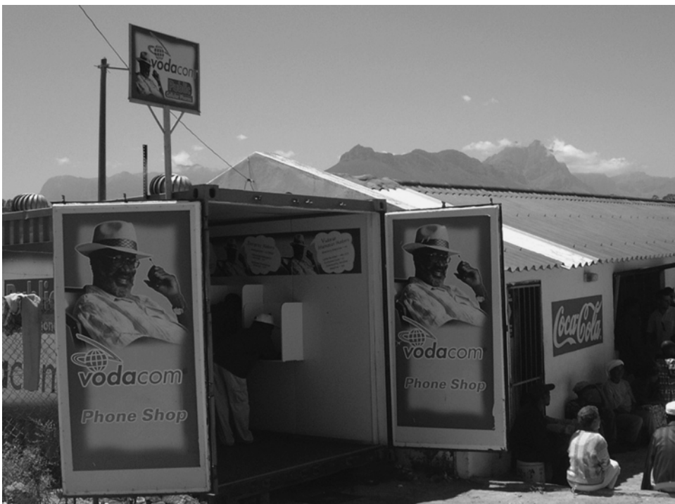
Figure 5.2 South African telecom container.
