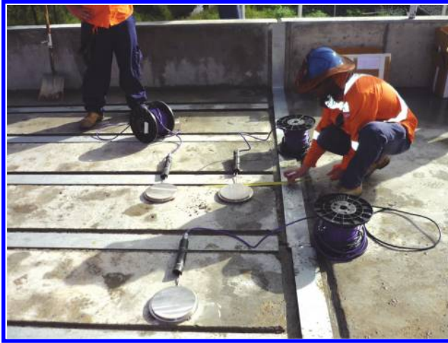
Figure C5 Installation of pressure cells at Mudies Creek bridge near Singleton.
