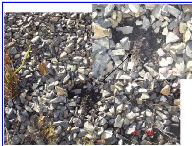
Figure C7 Intrusion of coal fines in to the shoulder ballast in a track near Rockhampton, Queensland.
