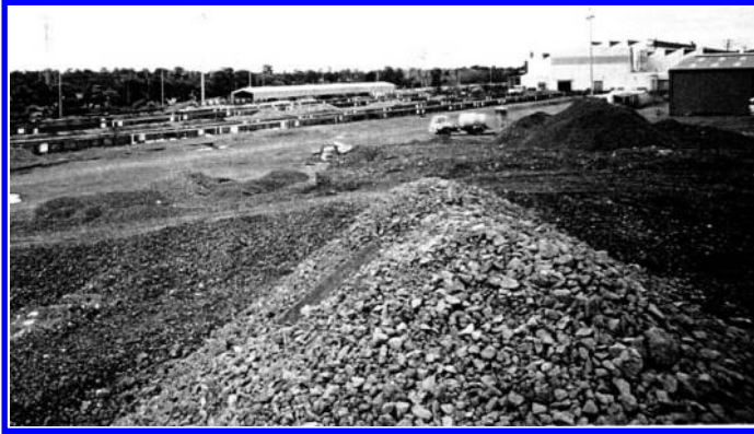
Figure 14.7 Stockpiles of waste ballast at Chullora (NSW).
