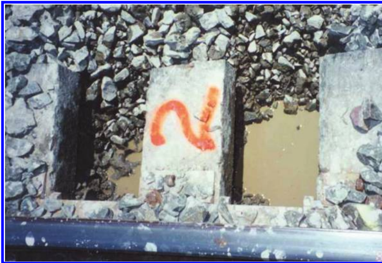
Figure 1.6 Ponding water in the load bearing ballast along a Sydney metropolitan line in Australia.
