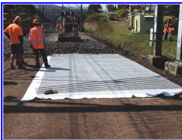
Figure C1 Laying the Geogrid over non-woven geotextile to form a geocomposite layer in fully instrumented rail track at Bulli town north of Wollongong City, New South Wales.
