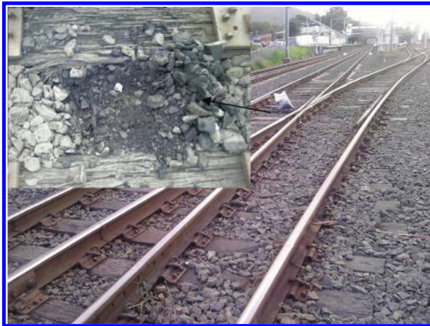
Figure C10 Pulverization of ballast plus coal fouling observed near v-crossing close to Thirroul, New South Wales.
