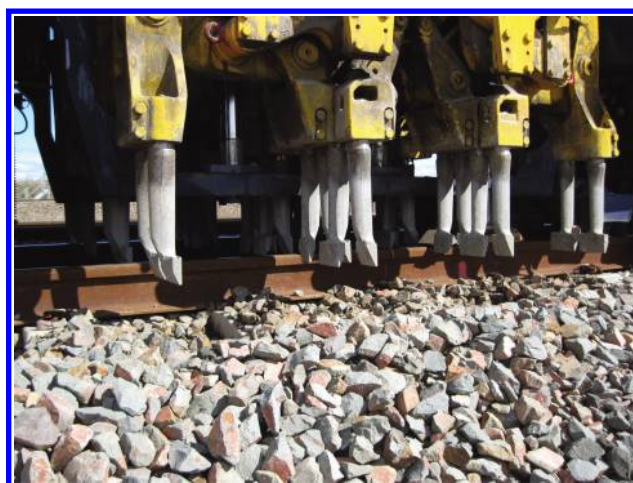
Figure C4 Automated tamping equipment at Singleton.
