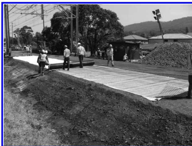
Figure 10.3 Placement of geocomposite over capping layer.
