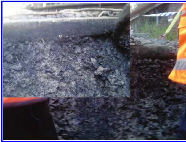
Figure C9 Coal and clay sediments fouling the ballast beneath the sleeper at a site in Thirroul, south of Sydney, observed during track maintenance.
