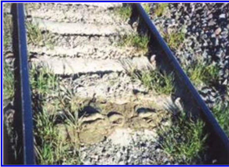
Figure 1.8 Dried slurry deposited around the sleepers.
