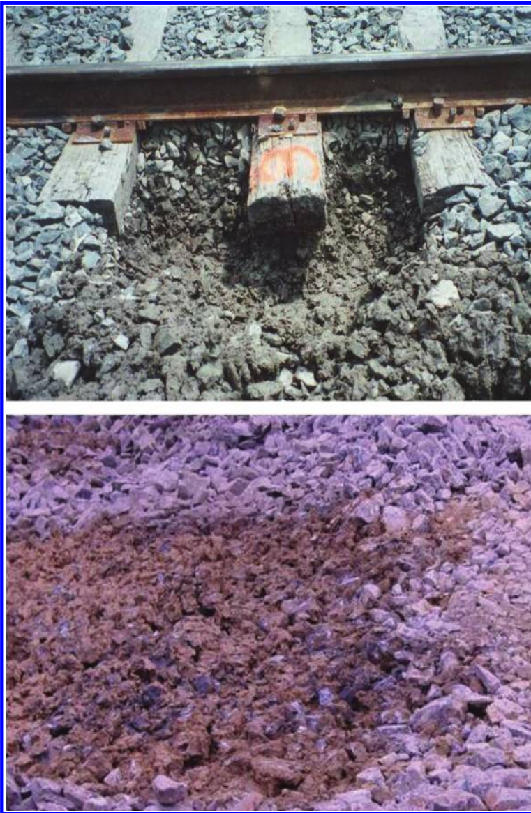
Figure 1.4 Fouled ballast.
