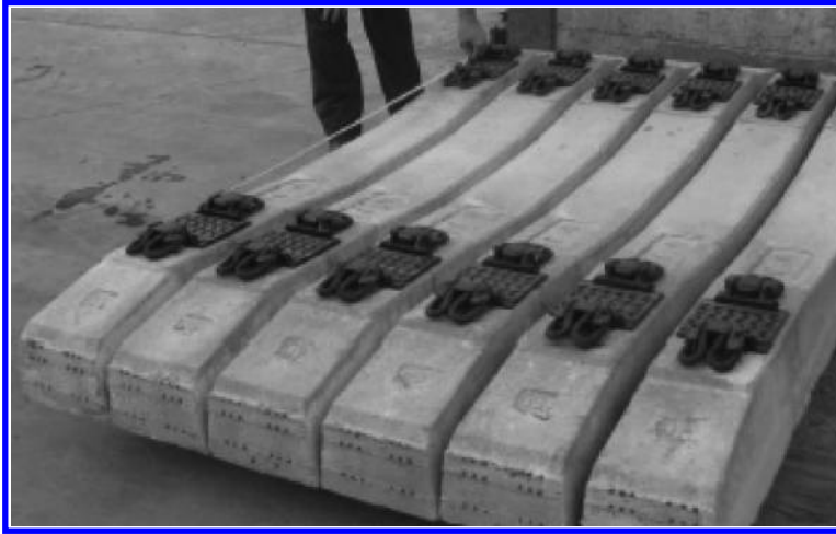
Figure 2.4 Concrete-frame sleeper used in track (Courtesy RailCorp).
