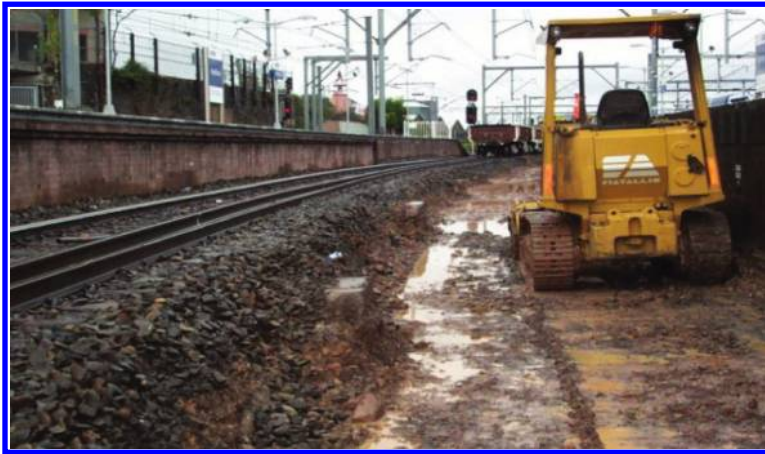
Figure 1.5 Insufficient drainage along a railway line in New South Wales, Australia.
