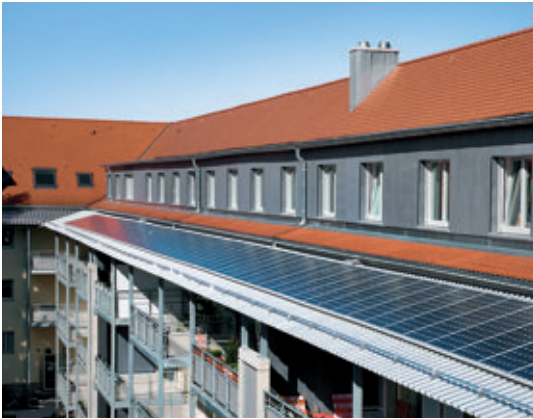
B 06.06 Energy evaluation B 06.07 Technical schematic of energy provision B 06.08 Photovoltaic array on the roof of the new balconies
