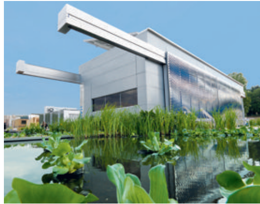
B 23.03 Team Virginia – Lumenhaus. The south facade with the layered, sliding facade elements and the projecting beams for “parking” the elements.
