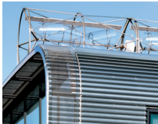
A 2.01 Rooftop wind turbines, five-story residential building in Chicago, Illinois, USA 2007, Murphy/Jahn.
