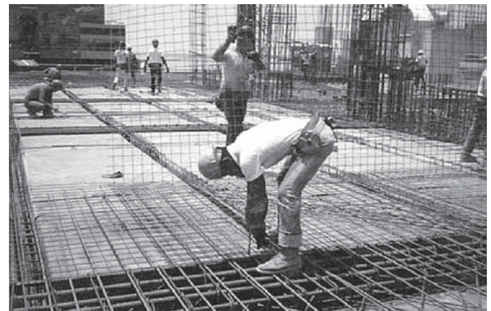
FIGURE 22.9 Welded wire reinforcement. (a) Welded wire reinforcement wire diameter and spacing and use in a concrete slab detail. (b) Welded wire reinforcement represented in a structural section. (c) Welded wire reinforcing being used on a construction project. © Cengage Learning 2012
