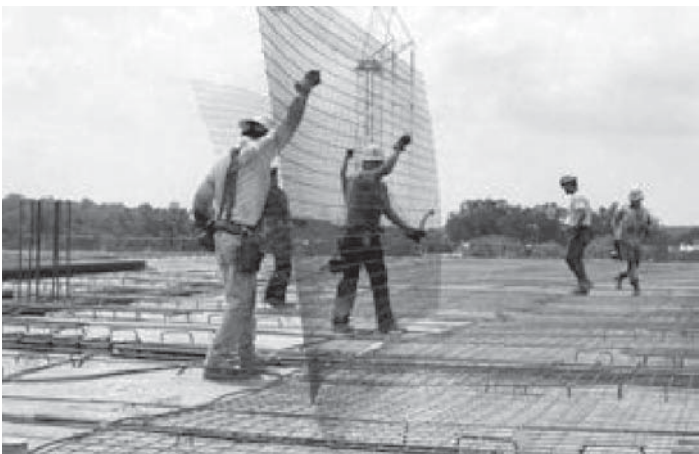
FIGURE 22.9 Welded wire reinforcement. (a) Welded wire reinforcement wire diameter and spacing and use in a concrete slab detail. (b) Welded wire reinforcement represented in a structural section. (c) Welded wire reinforcing being used on a construction project. © Cengage Learning 2012
