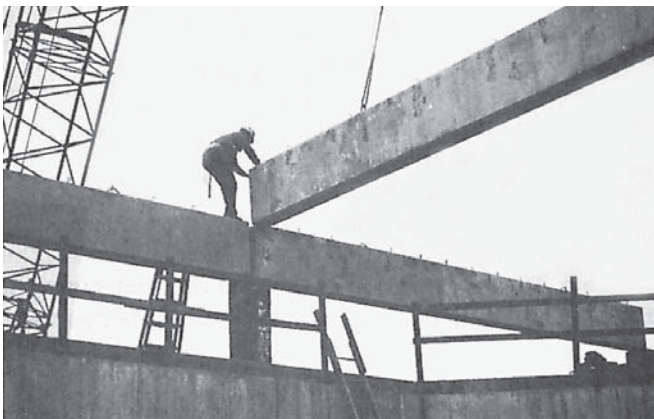
FIGURE 22.15 Precast concrete beams and panels are often formed off-site, delivered to the job site, and then set into place with a crane. © Cengage Learning 2012
