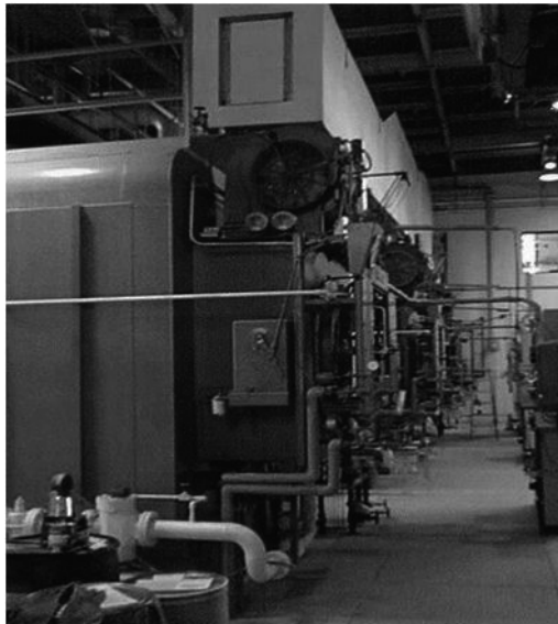
Figure 2-4. Multiple Power Boilers in the Powerhouse Area
