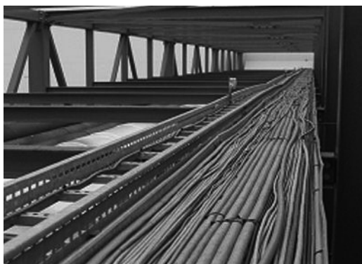
Figure 2-3. Cable Tray and Conduit for Instrumentation Wiring
