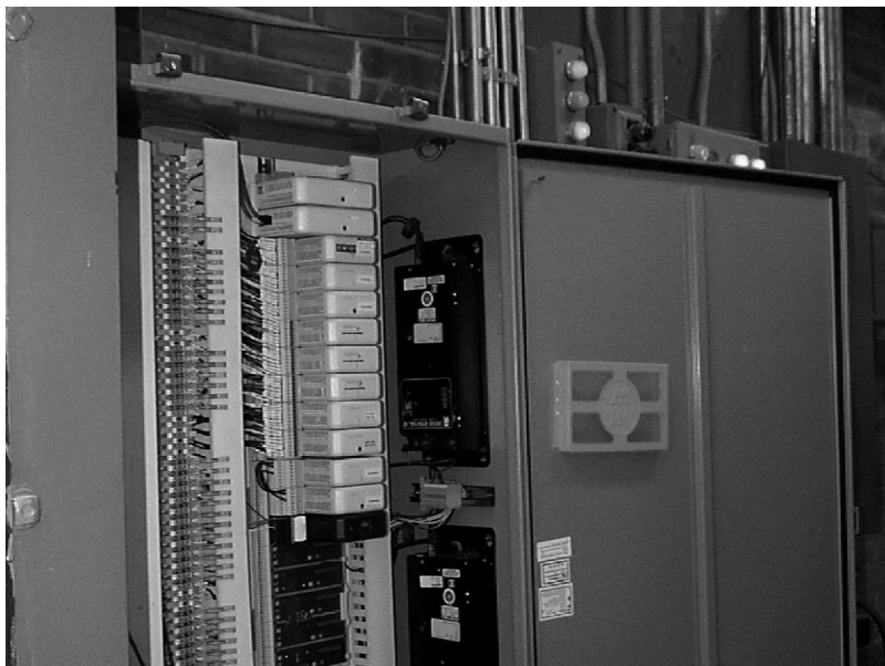
Figure 2-20. Field Wiring and Terminations
