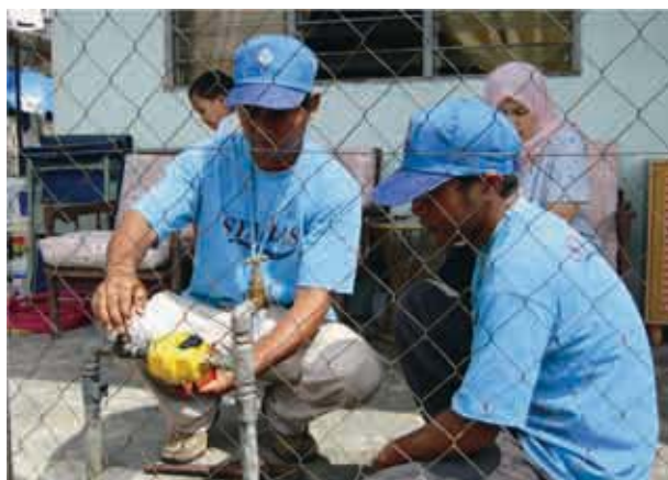
Meter replacement: Ensuring accurate billing through replacement of aging meters in Kuala Lumpur. Photo by Abdul Raof Ahmad, Corporate Communications and Public Affairs Division, SYABAS.
