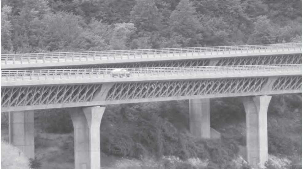
Figure 9.31 Viaduc des Glacières on the A40 motorway, France (Photo: Robert Benaim)
