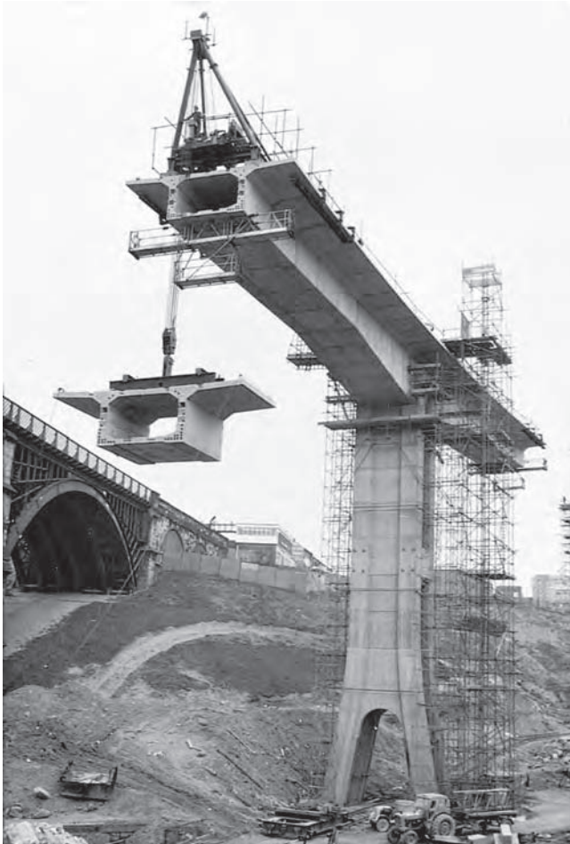
Figure 15.31 Byker Viaduct: erection using shear legs (Photo: J. Mowlem/North East Studios)
