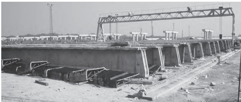
Figure 10.18 GSZ Superhighway, Pearl River Delta Viaducts: main casting yard (Photo: Benaim)
