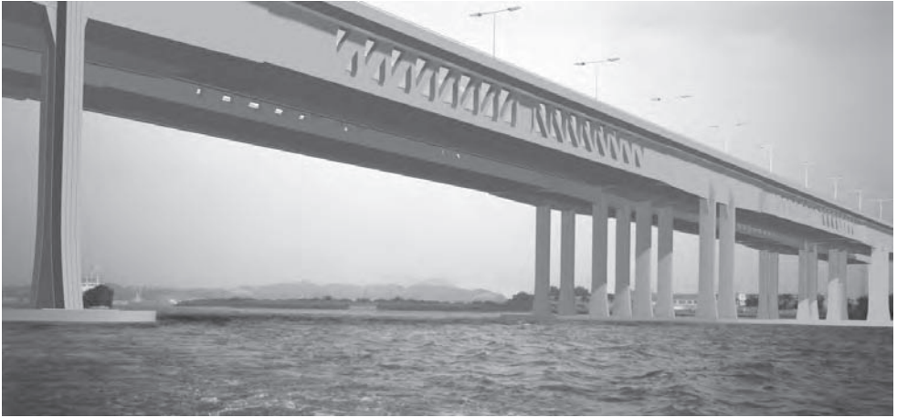
Figure 9.32 Dong Po South Bridge (Image: David Benaim)
