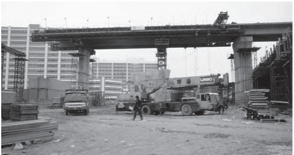
Figure 12.2 Contract 304 HKMTR: semi-mechanised falsework (Photo: Robert Benaim)
