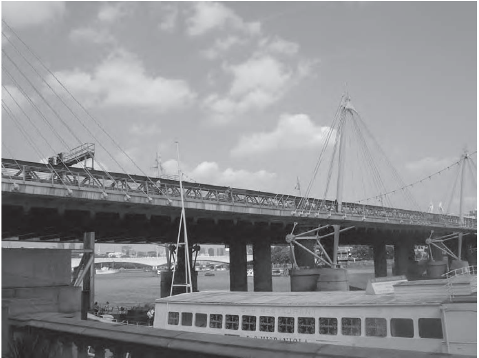
Figure 1.11 Hungerford Footbridge (Photo: Robert Benaim)
