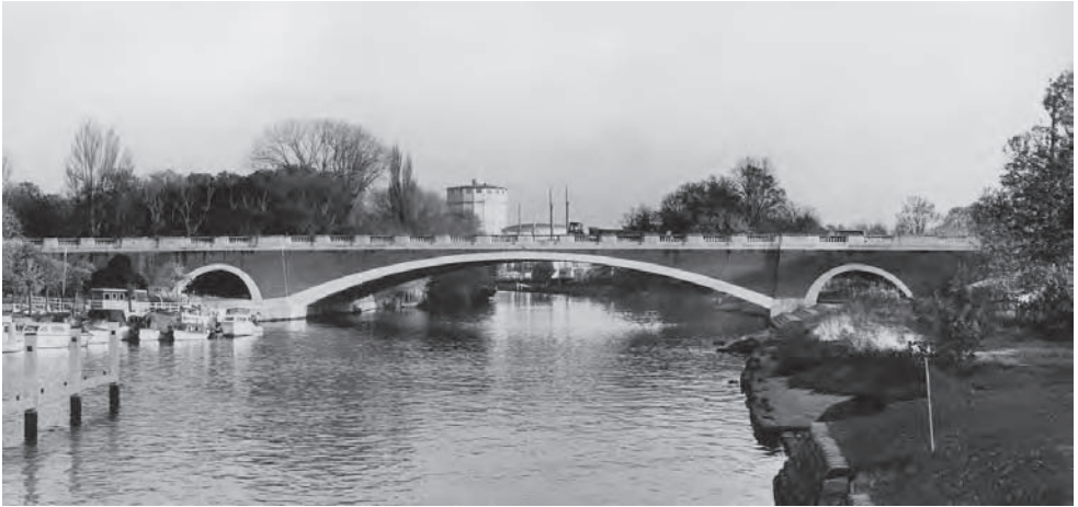
Figure 1.12a Runnymede Bridge: original Lutyens design (Photo: Arup)
