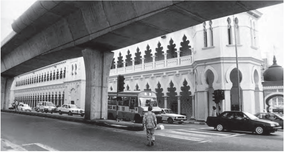
Figure 1.4 STAR Viaduct: typical pier (Photo: Benaim)
