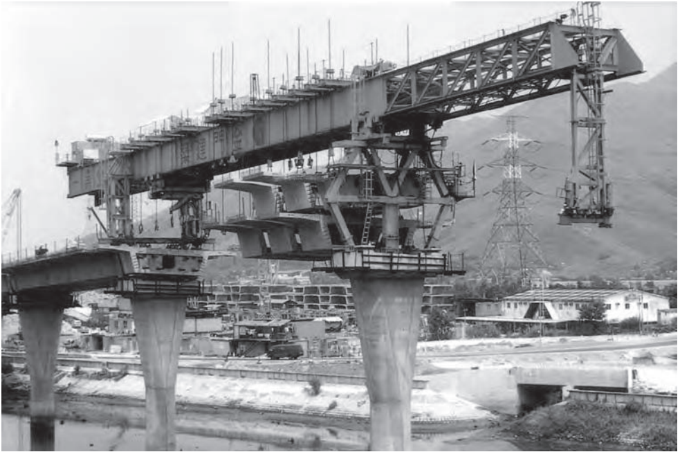
Figure 15.8 Route 3 Gantry (Photo: Benaim)
