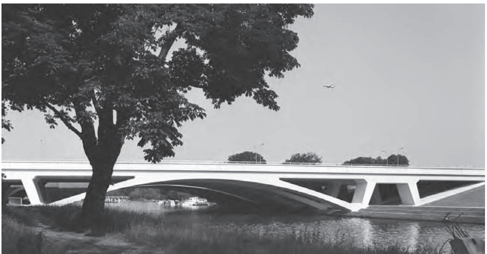
Figure 1.12c New Runnymede Bridge (Photo: Harry Sowden/Arup)
