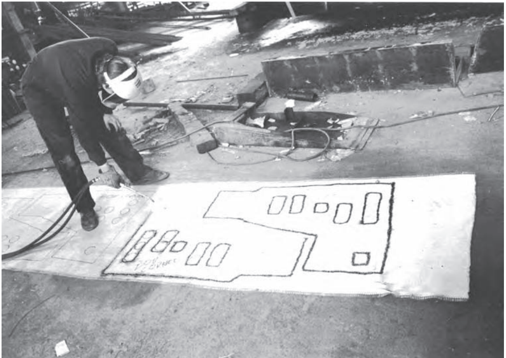
Figure 14.20 Byker Viaduct: preparing fibreglass steering packs (Photo: Robert Benaim)
