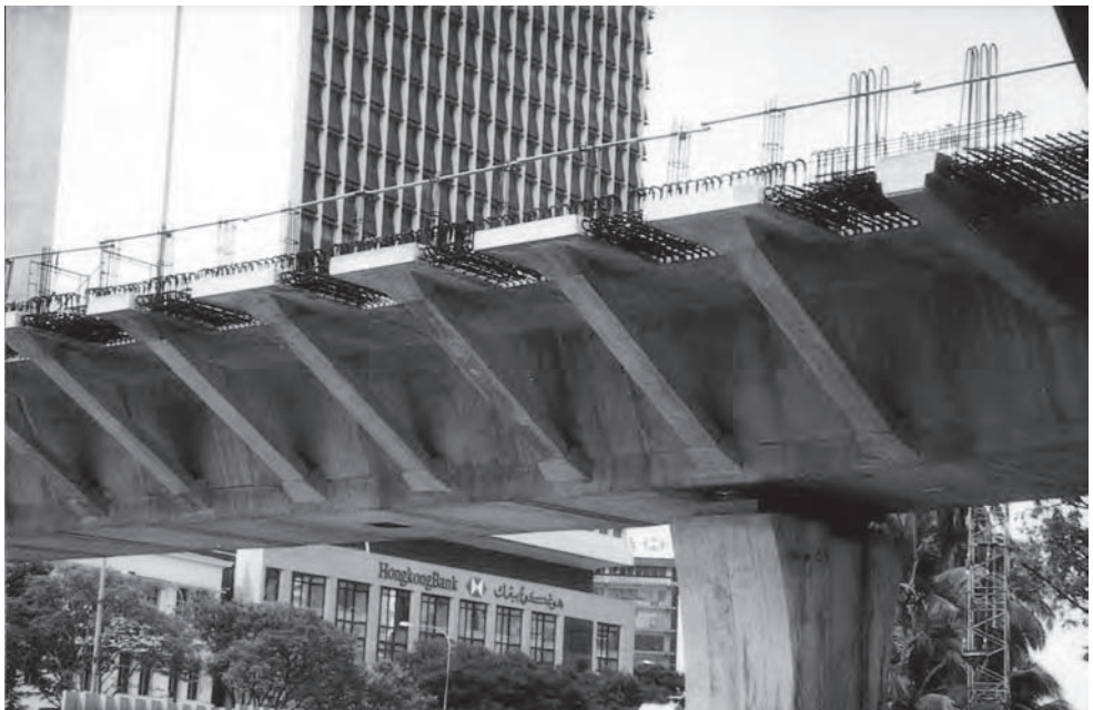
Figure 9.11 STAR Viaduct: stitches between precast segments (Photo: Benaim)
