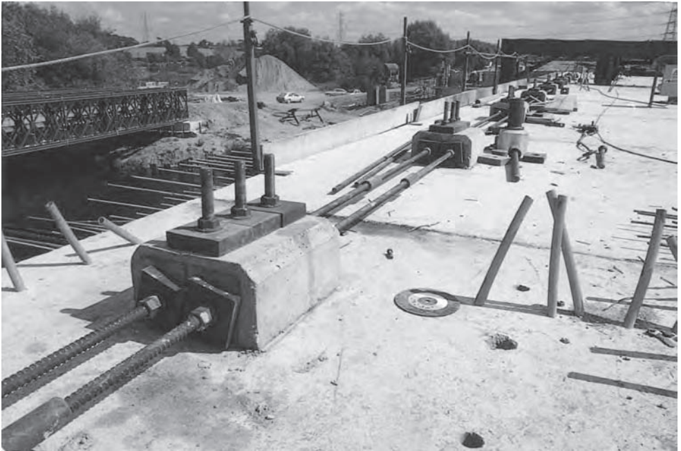
Figure 15.11a Temporary prestressing anchors: River Lea Viaduct, Stanstead Abbots Bypass, concrete blocks (Photo: Benaim)
