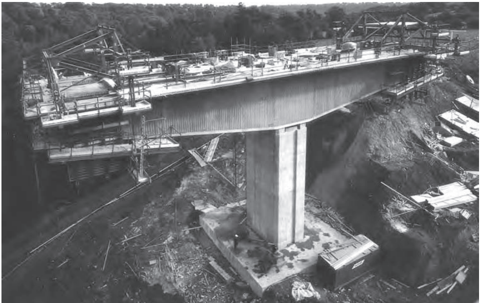
Figure 15.15 Travellers for River Dee Bridge, Newport, UK (Photo: Edmund Nuttall/Molyneux Photography)
