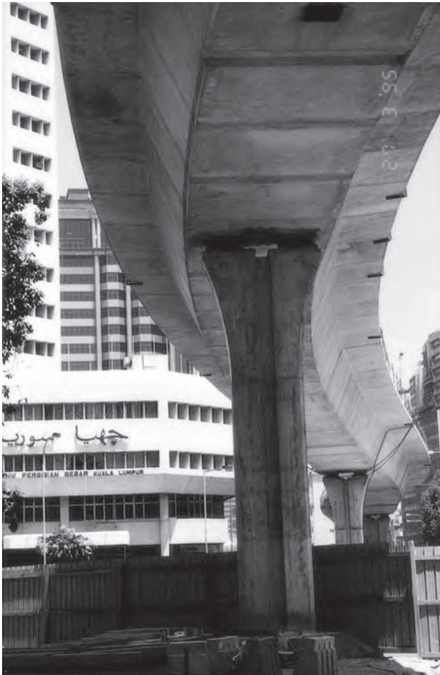
Figure 7.11 Pier of STAR Viaduct (Photo: Benaim)
