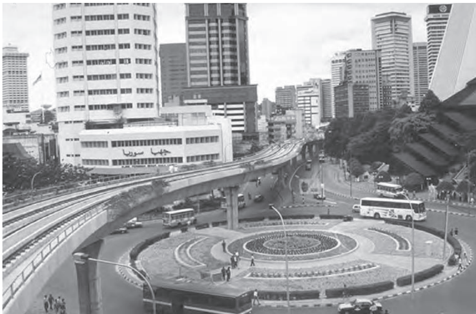
Figure 7.22 STAR Viaduct (Photo: Benaim)
