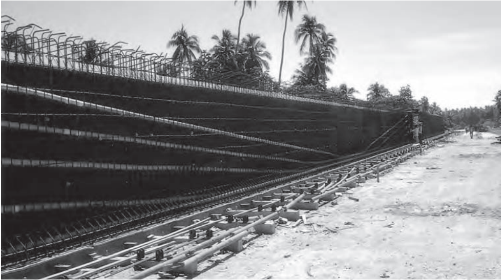
Figure 5.12 Cables in a typical beam (Photo: Benaim)
