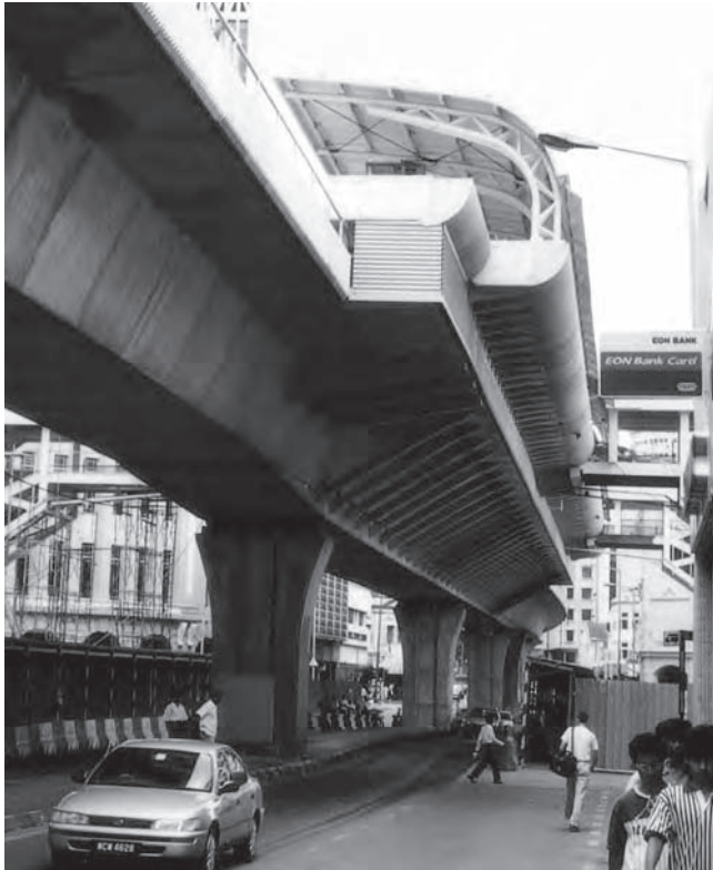
Figure 9.9 STAR Viaduct: elevated station (Photo: Benaim)
