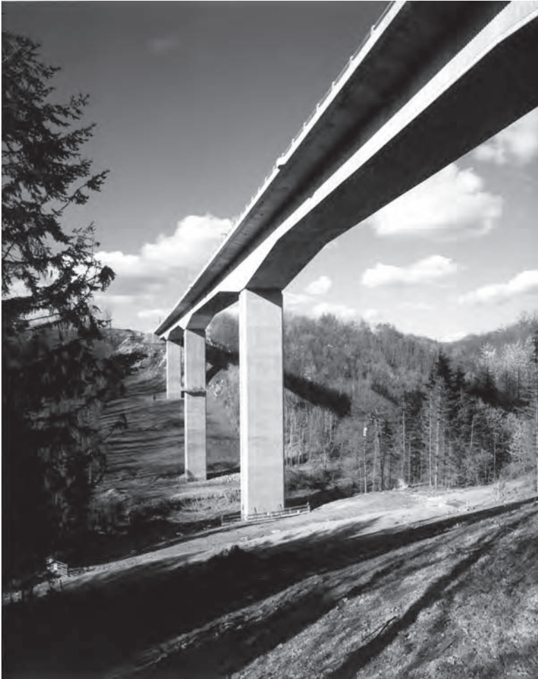
Figure 13.3 River Dee Bridge: effect of side cantilever on the appearance of a variable depth deck (Photo: Edmund Nuttall)
