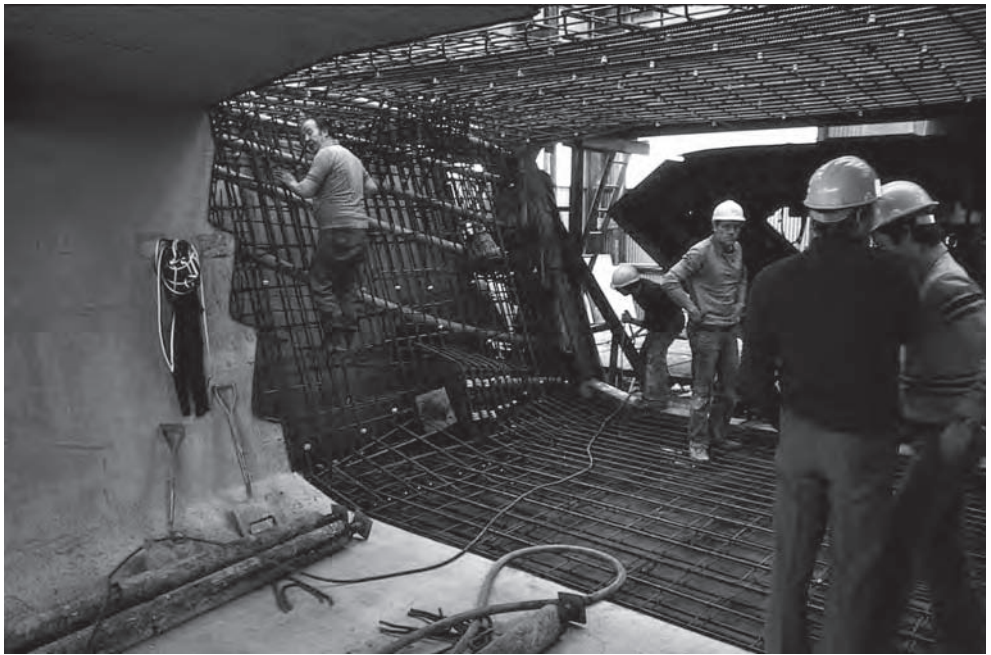
Figure 14.12 East Moors Viaduct: reinforcing cage (Photo: Benaim)
