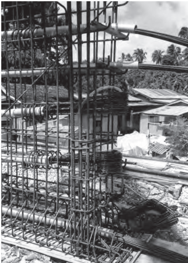
Figure 5.9e Typical prestress anchors: buried dead anchors (Photo: Benaim)
