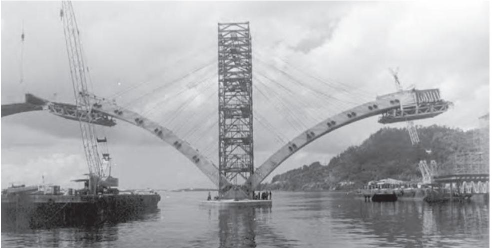
Figure 17.17 Bridge over Sungai Dinding: balanced cantilever construction of arch (Photo: Benaim)
