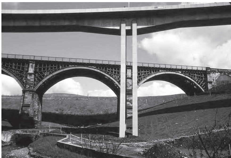
Figure 7.24 Byker Viaduct: valley piers (Photo: Robert Benaim)
