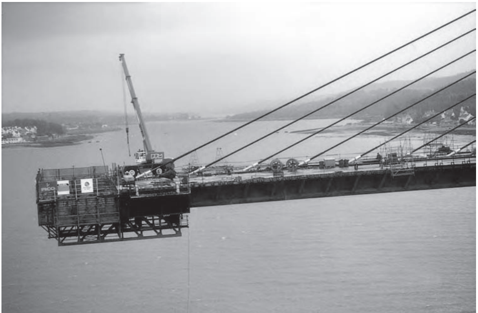
Figure 18.14 Pont sur l'Elorn: balanced cantilever construction (Photo: Robert Benaim)
