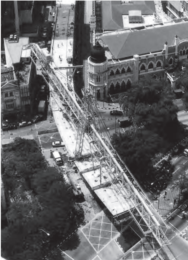
Figure 15.32 STAR Viaduct: gantry erection (Photo: Benaim)
