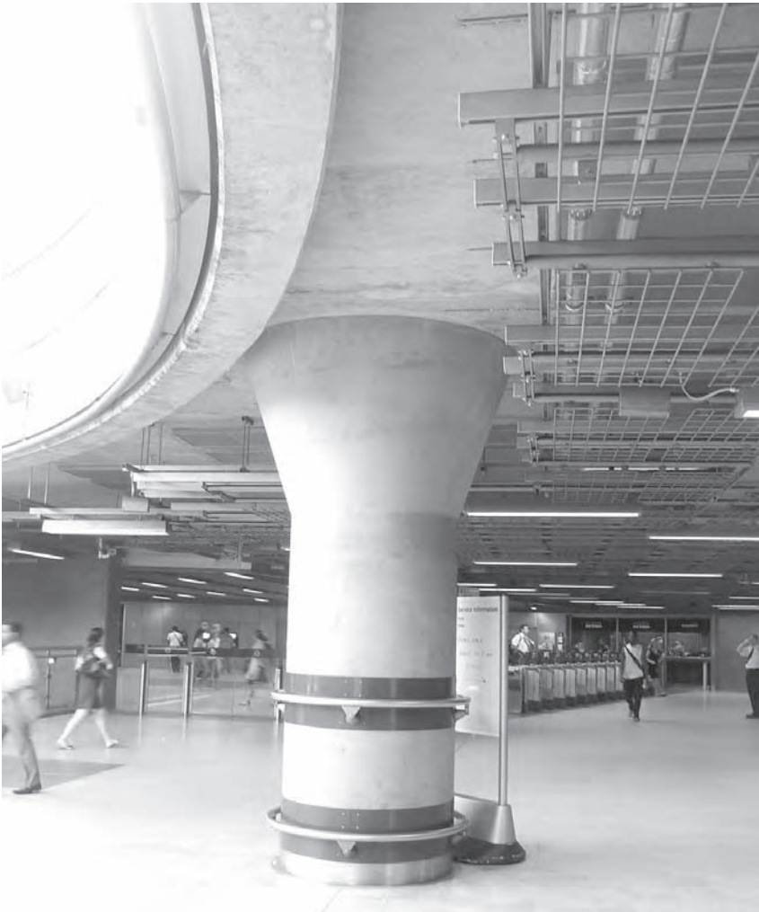
Figure 11.3 Canada Water underground station: roof slab carrying bus station (Photo: Robert Benaim)
