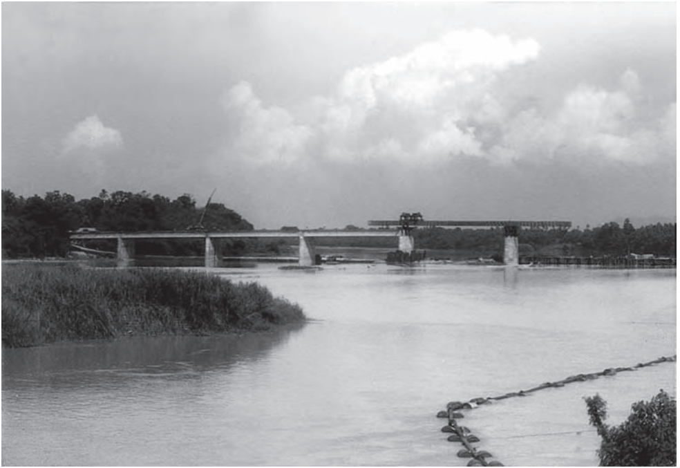
Figure 10.13 Sungai Kelantan Bridge (Photo: Robert Benaim)
