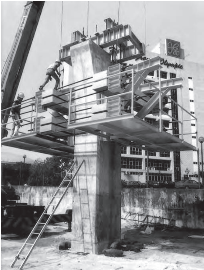
Figure 15.33 STAR Viaduct: load testing the pier head falsework (Photo: Benaim)
