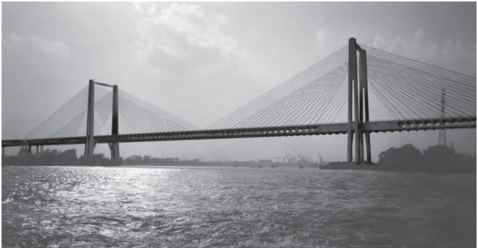
Figure 18.18 Project for Ah Kai Sha Bridge (Image: David Benaim)
