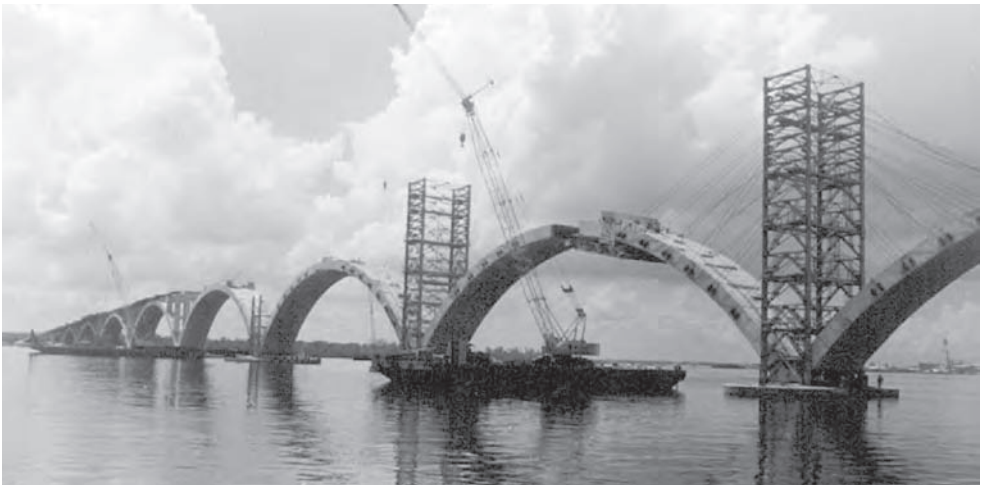
Figure 17.18 Bridge over Sungai Dinding: span-by-span erection of arches (Photo: Benaim)
