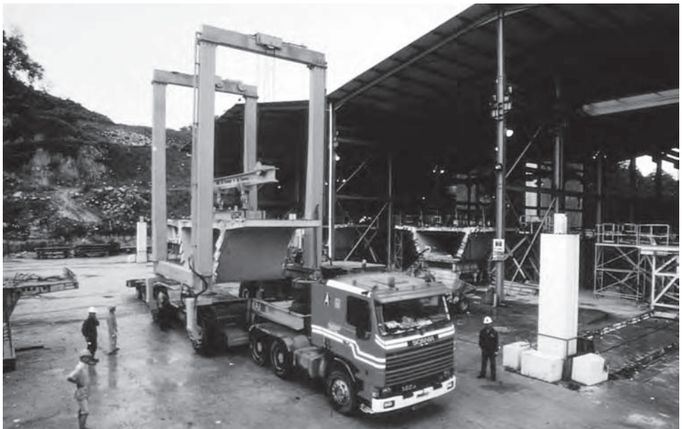
Figure 14.15 STAR: segment handler (Photo: Benaim)
