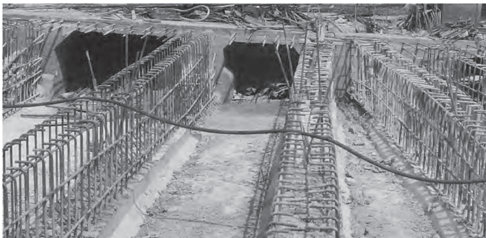
Figure 11.18 Multi-cell box girder under construction (Photo: Robert Benaim)
