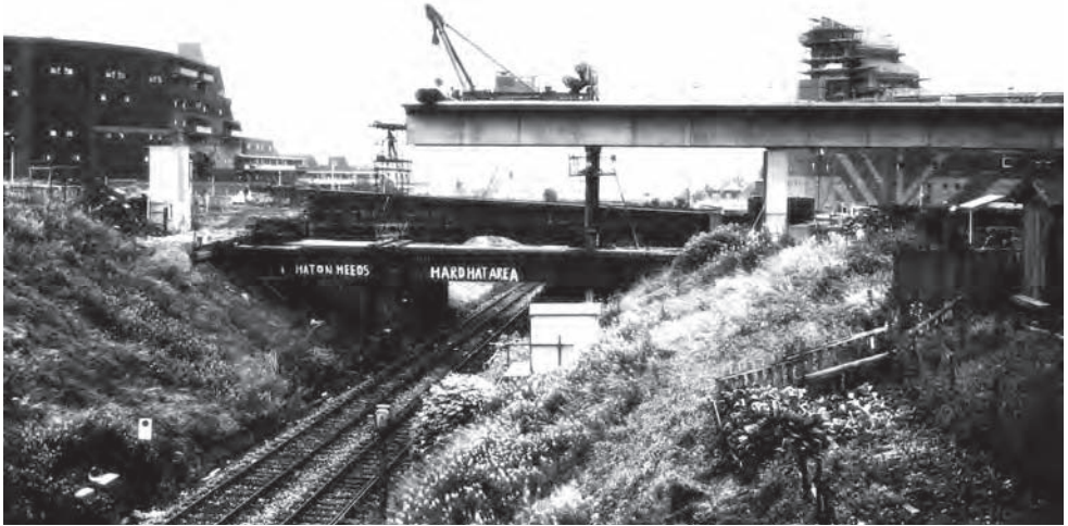
Figure 15.35 Byker Viaduct, Newcastle: progressive erection of decks (Photo: Arup)
