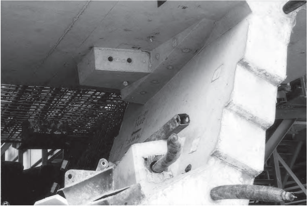
Figure 14.7 STAR: permanent and temporary anchorage blisters (Photo: Benaim)
