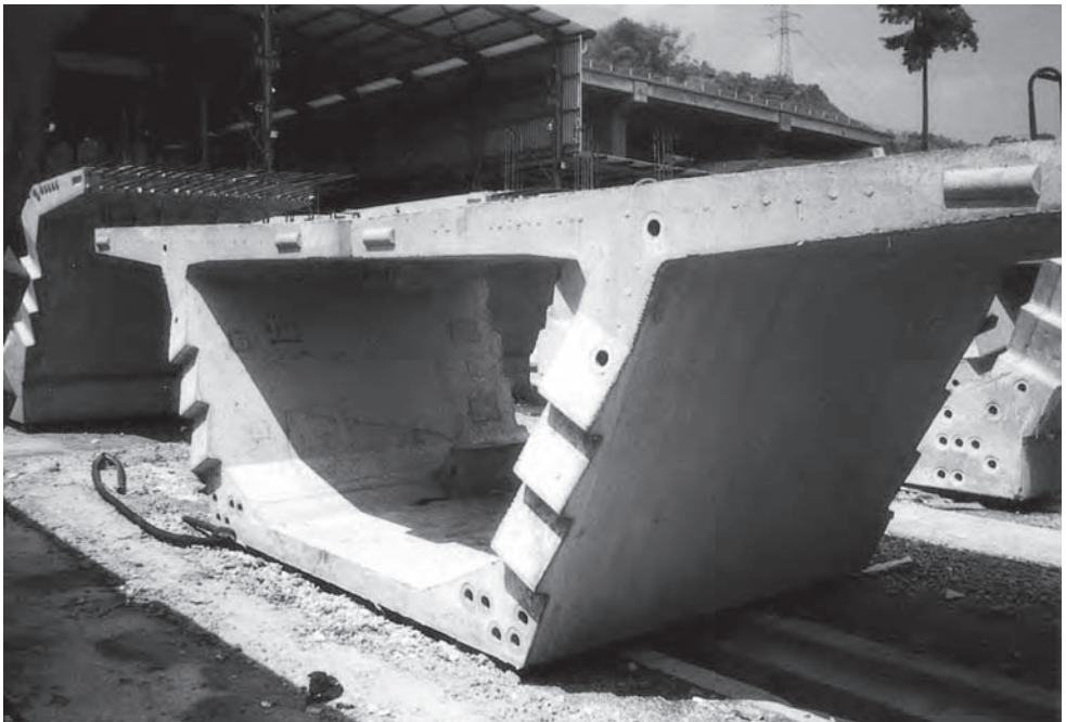
Figure 14.9 STAR: typical segment details (Photo: Benaim)
