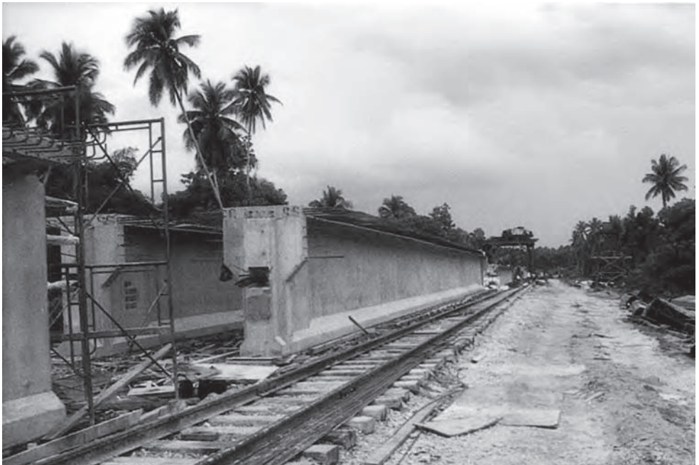
Figure 10.14 Sungai Kelantan Bridge: casting yard (Photo: Robert Benaim)
