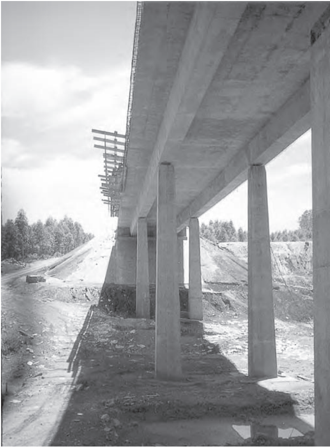
Figure 12.1 Doornhoek Bridge, South Africa: typical twin rib bridge (Photo: Arup)
