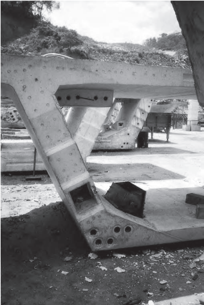
Figure 14.8 STAR: temporary blister cast-on after precasting (Photo: Benaim)
