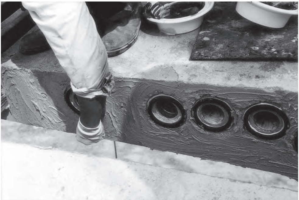
Figure 14.19 STAR: application of resin (Photo: Benaim)
