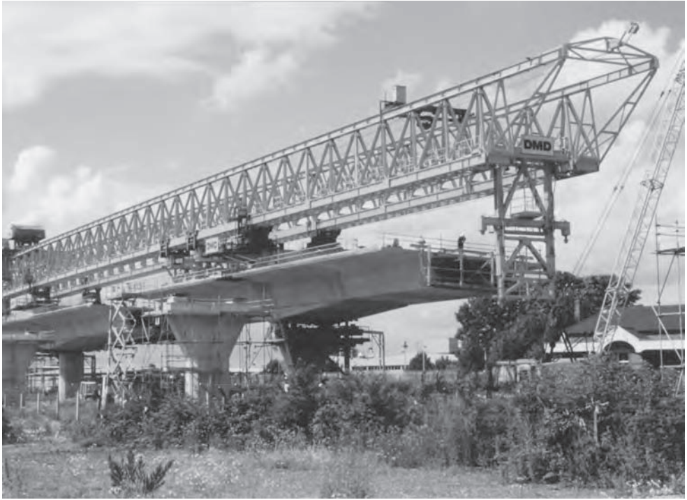
Figure 15.34 Dagenham Dock Viaduct: gantry erection (Photo: DEAL S.r.l.; www.deal.it )
