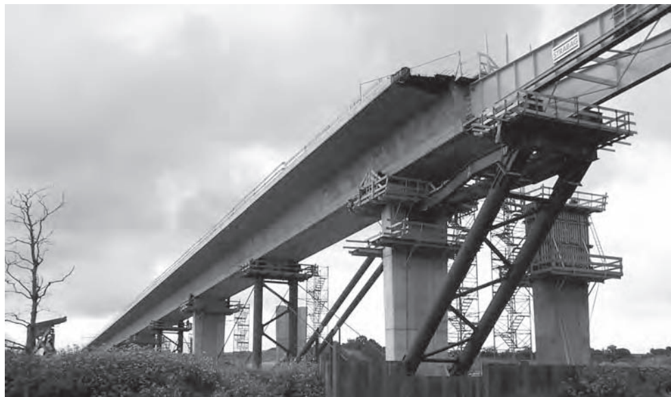
Figure 15.37 Blackwater Viaduct, Ireland (Photo: Strabag SE)
