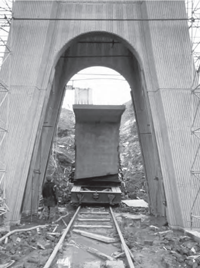
Figure 1.8 Byker Viaduct under construction (Photo: Arup)
