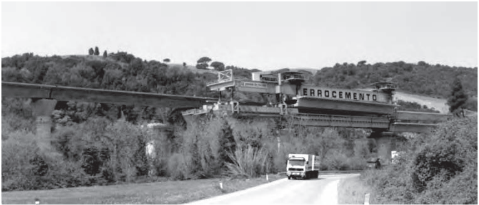
Figure 15.45 Poggio Iberna Viaduct, Italy: launching gantry (Photo: David Benaim)
