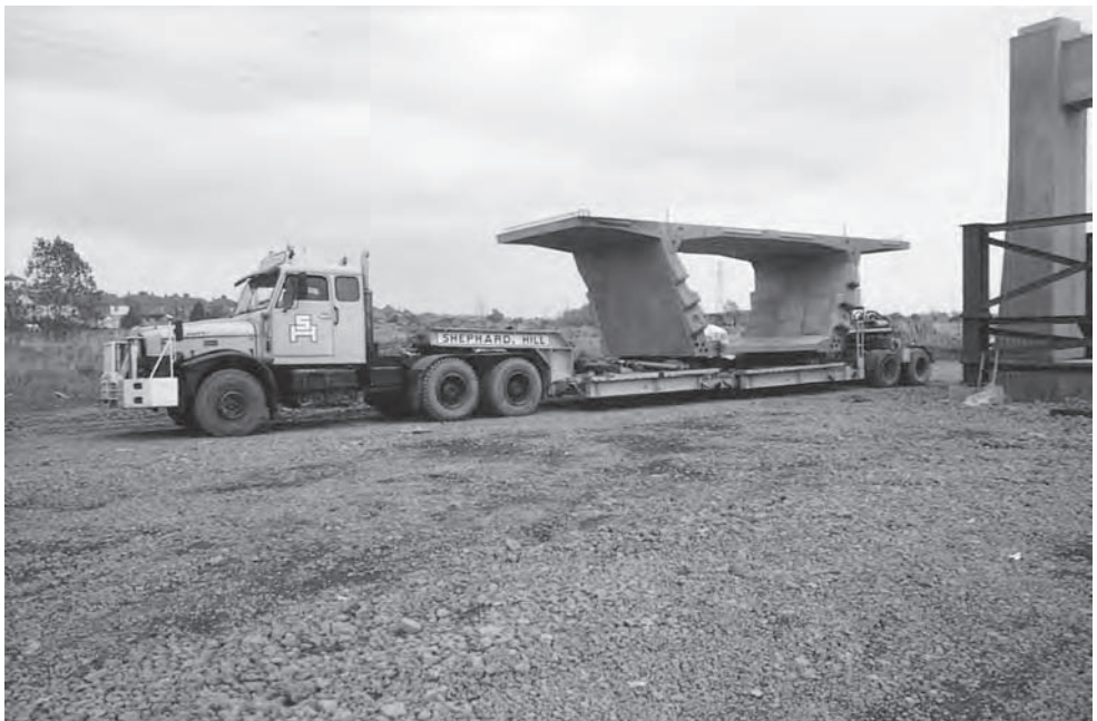
Figure 14.18 East Moors Viaduct: segment transport by low loader (Photo: Benaim)
