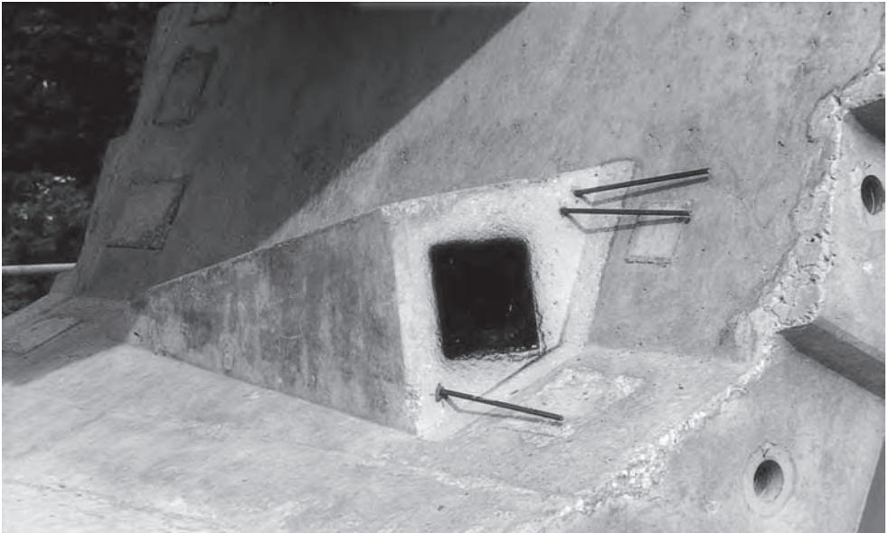
Figure 6.29c Anchorage blisters for tendons: internal blister (Photo: Benaim)
