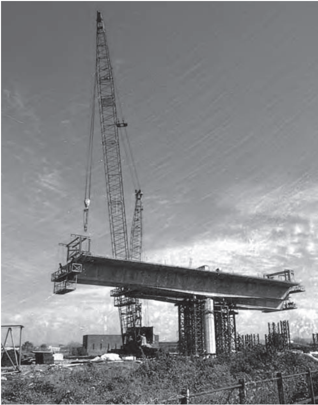
Figure 15.30 Grangetown Viaducts, Cardiff: erection by fixed crane (Photo: Robert Benaim)
