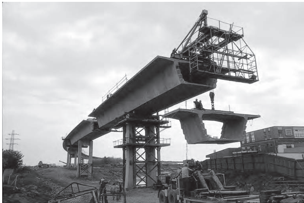
Figure 7.26 East Moors Viaduct (Photo: Benaim)
