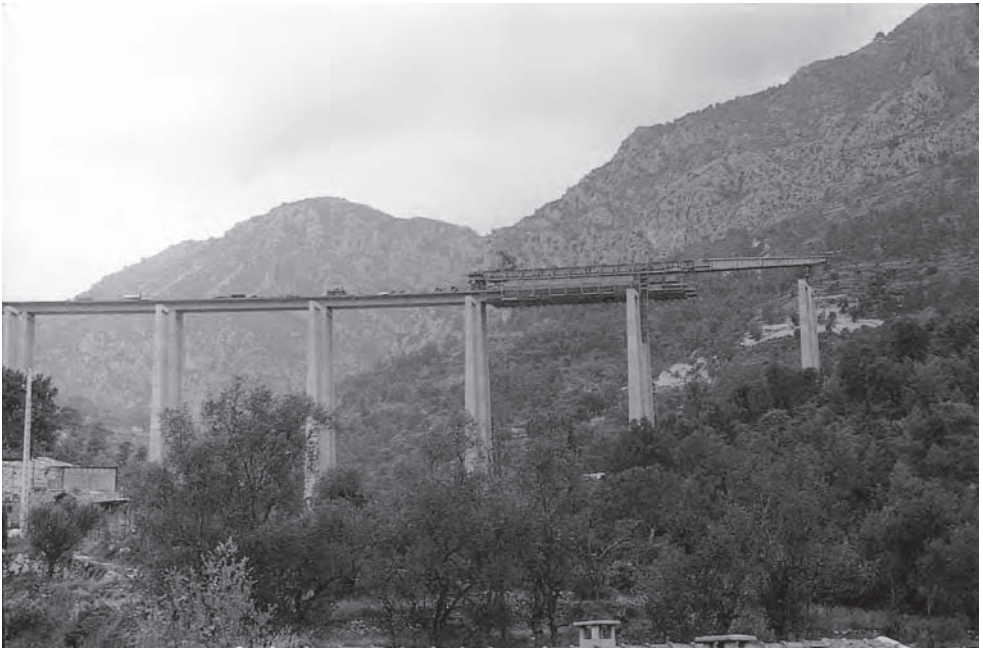
Figure 15.1 Autoroute A8, France: span-by-span construction of box decks (Photo: Robert Benaim)
