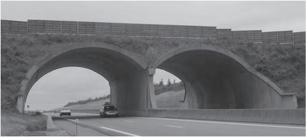
Figure 17.11 Bridge on A16, France (Photo: Robert Benaim)
