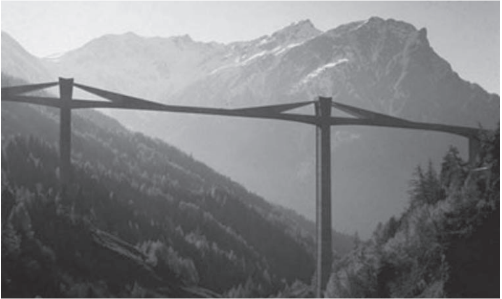
Figure 18.3 Ganter Bridge (Photo: Christian Menn)
