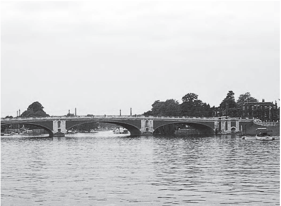
Figure 1.13 Hampton Court Bridge by Lutyens (Photo: Robert Benaim)
