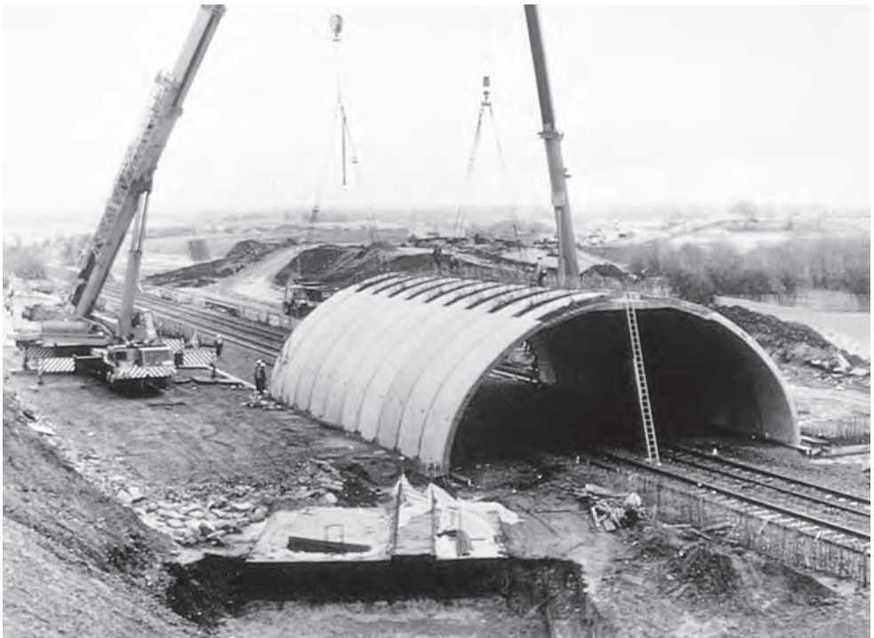
Figure 17.10 Maryville arch under construction (Photo: Benaim)
