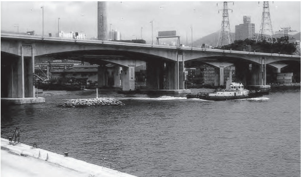
Figure 15.13 Kwai Tsing Bridge, Hong Kong (Photo: Benaim)
