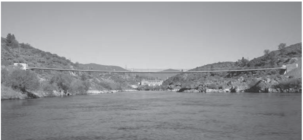
Figure 18.24 Redding Bridge (Photo: Jiri Strasky)
