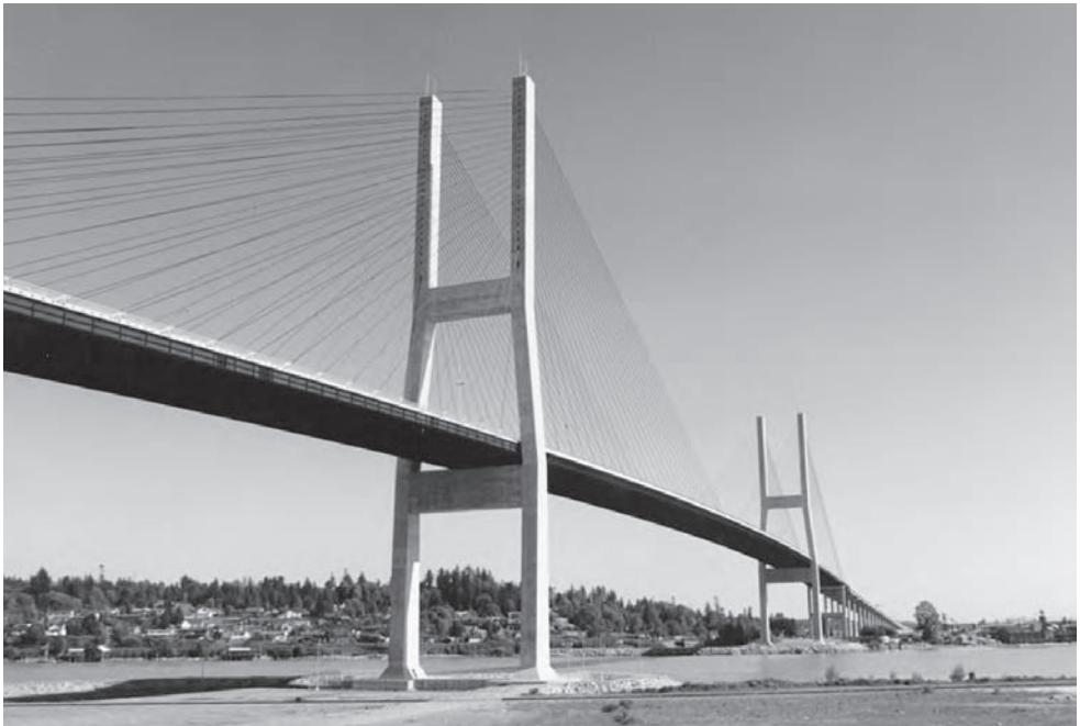
Figure 1.10 Alex Fraser Bridge towers (Photo: Henning J. Woolf/Buckland & Taylor)
