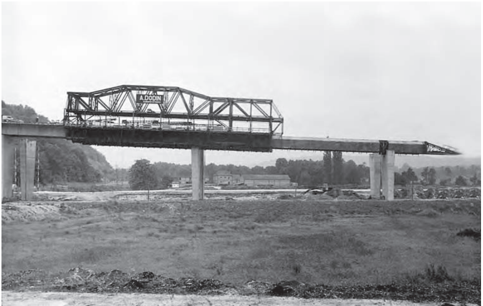
Figure 15.6 Viaduc d'Incarville: falsework truss being launched (Photo: Robert Benaim)
