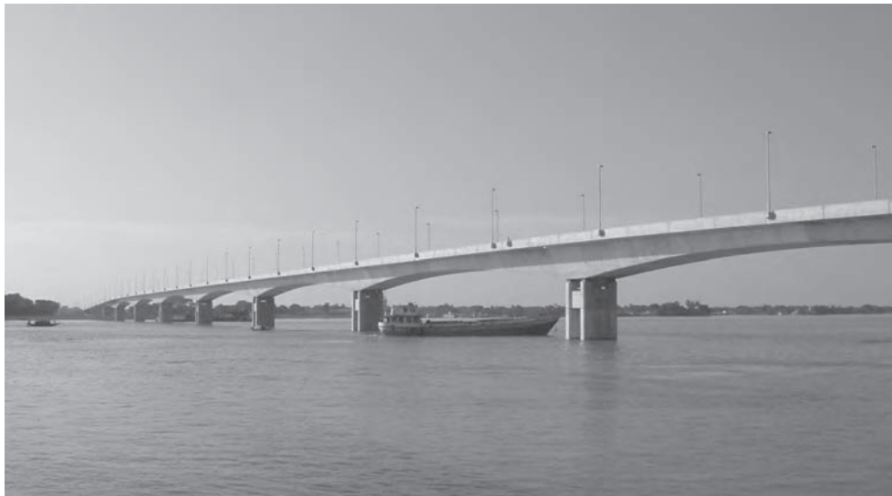
Figure 13.6 Bhairab Bridge, Bangladesh (Photo: Roads and Highways Department, Government of Bangladesh and Edmund Nuttall)
