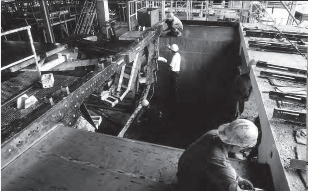
Figure 14.3 STAR: casting cell ready to receive reinforcement cage (Photo: Benaim)
