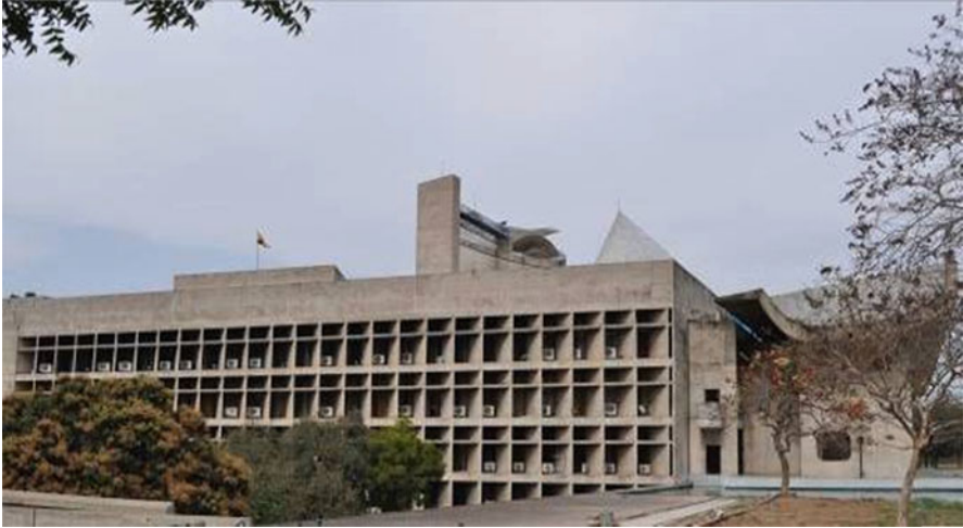
Fig. 10.5 The Assembly building in Chandigarh (Photo: Rob Roggema)
