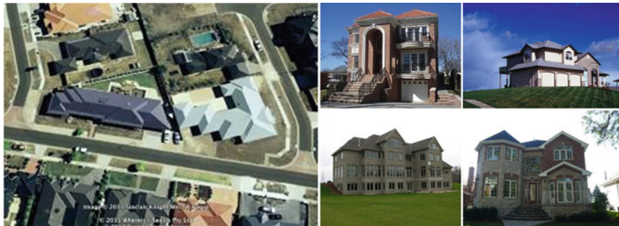
Fig. 1.4 Results of Australian urban design (Source: Google Earth and collected from internet, Rogema 2010)
