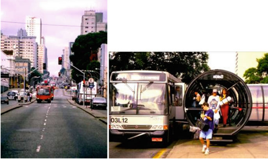
Fig. 10.25 Bus lane and bus stop, Curitiba (Photos: Rob Roggema)
