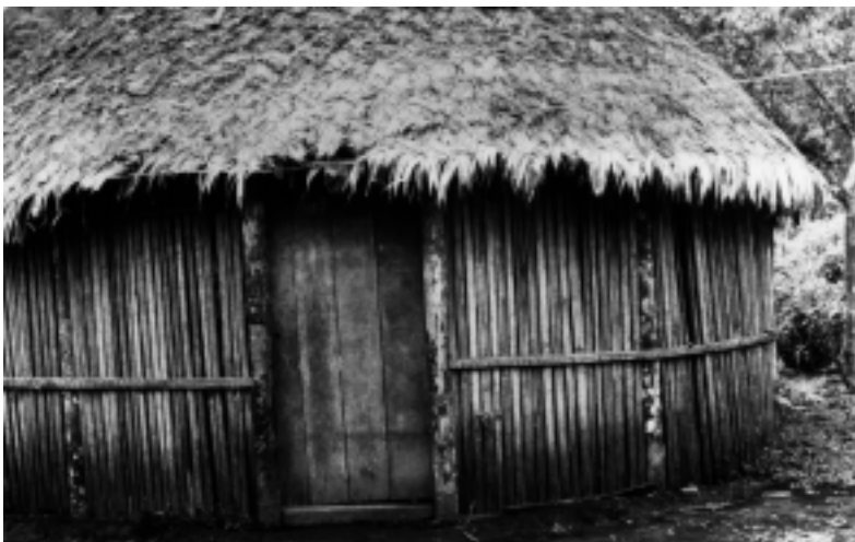
Traditional house built by Shuar people in Amazonian Ecuador. The posts are whole stems of Iriartea ; the walls are made of stems that have been split into narrow strips. The roof was made of thatch from a different palm species (photo by Patti Anderson).
