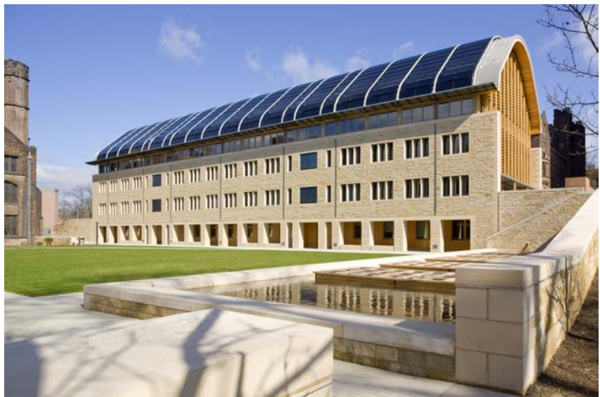
Figure 1.10 (A) Kroon Hall at Yale University in New Haven, Connecticut, is located on a former industrial area that included a decommissioned power plant, a derelict parking lot, and a network of service roads. A 100-kW photovoltaic array on the roof provides about 25 percent of the building's electricity needs. (Robert Benson Photography)
