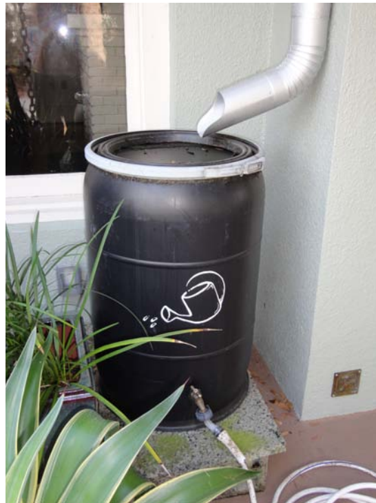
Figure 10.16 (B) Rain barrels collect roof runoff and store it for later nonpotable use. (Maxine Thomas, Florida Master Gardener/University of Florida–IFAS Extension Realtor ® )
