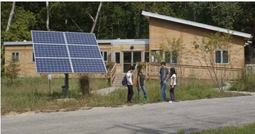
Figure 2.16 The Tyson Living Learning Center in Eureka, Missouri. Miscalculations initially resulted in this building falling short of energy performance goals. Due to the ambitious sustainability requirements of the Living Building Challenge, postconstruction adjustments were made by adding insulation in several areas, retrofitting storm windows, and adjusting the HVAC system. These improvements led to the project achieving the desired NZE performance by the end of its first year in operation. (David Kilper, WUSTL)
