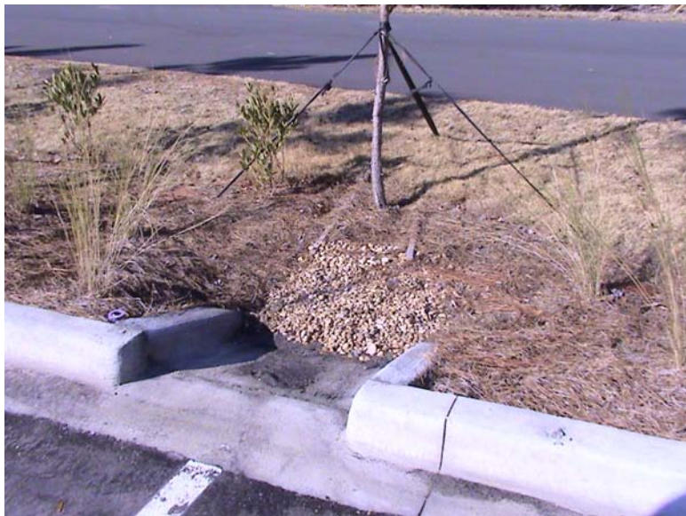
Figure 6.4 Bioswales surrounding the parking lot reduce stormwater runoff into nearby wetland areas. (D. Stephany)
