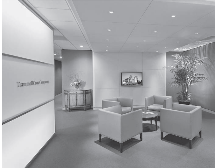
Figure 9.20 Fiberstars' EFO lighting, shown in Trammell Crow's office in Houston, Texas, is low-energy, lightweight, and ultrasafe because it does not conduct electricity. The manufacturer claims that a single EFO lamp uses 68 watts and replaces about 400 watts of halogen lamps. (Photograph courtesy of Fiberstars, Inc.)
