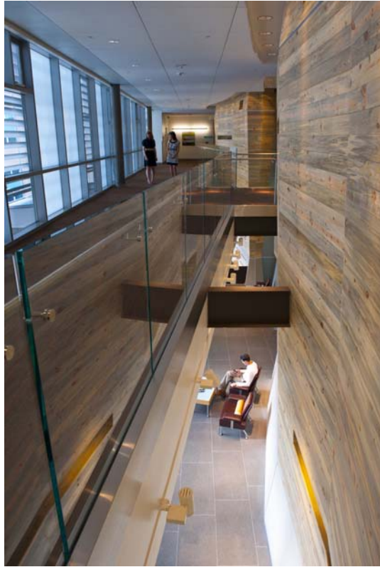
Figure 1.9 (C) The daylighting system for the NREL RSF was designed using extensive simulation. Shading devices were carefully placed on the exterior and interior to manage both direct and indirect sunlight, distributing it evenly to create a bright, pleasant working environment. (Source: National Renewable Energy Laboratory)
