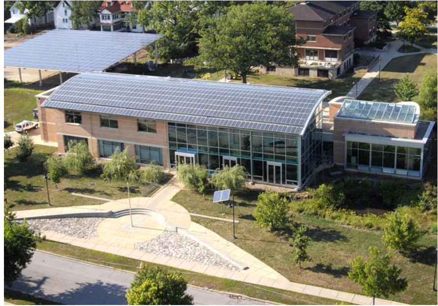
Figure 3.19 The Lewis Center for Environmental Studies at Oberlin College in Oberlin, Ohio, was built in the late 1990s and designed by an elite team of architects and other professionals, among them William McDonough, one of the leading green building architects, and John Todd, creator of the Living Machine, a waste treatment system that uses natural processes to break down the components of the building's wastewater stream. (Courtesy of Oberlin College)
