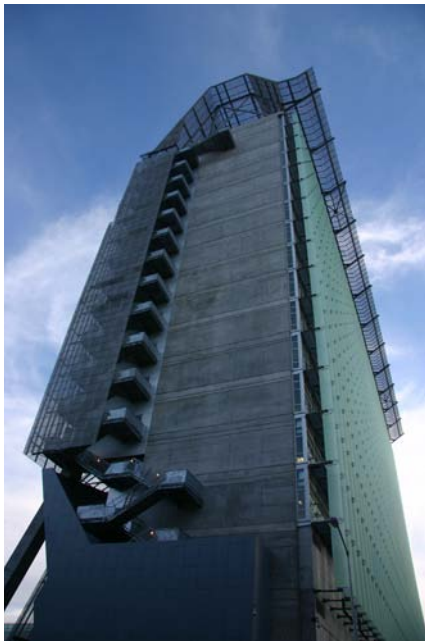
Figure 15.1 The Federal Building in San Francisco, California, designed by Morphosis Architects, is a breakthrough structure, with an outstanding passive design strategy coupled with active control systems. All building components are optimized in connecting the building to its surrounding environment for cooling, ventilation, and lighting. (Petros Raptis)
