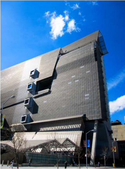
Figure 3.1 The Federal Building in San Francisco, California, exemplifies ecological design by employing local natural forces such as the prevailing winds and sunlight to provide cooling and daylighting. Detailed analysis of natural airflows induced by wind and thermal processes was accomplished using sophisticated computational fluid dynamics (CFD) modeling. (Illustration courtesy of Morphosis Architects)
