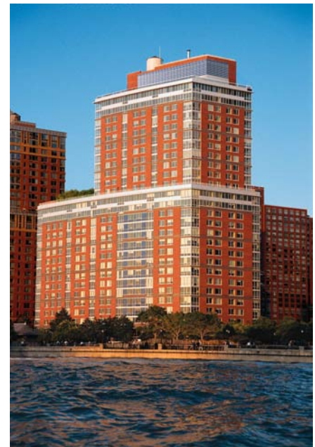
Figure 1.7 Solaire, a 27-story residential tower on the Hudson River in New York City, is the first high-rise residential building in the United States specifically designed to be environmentally responsible. (Photograph courtesy of the Albanese Development Corporation)
