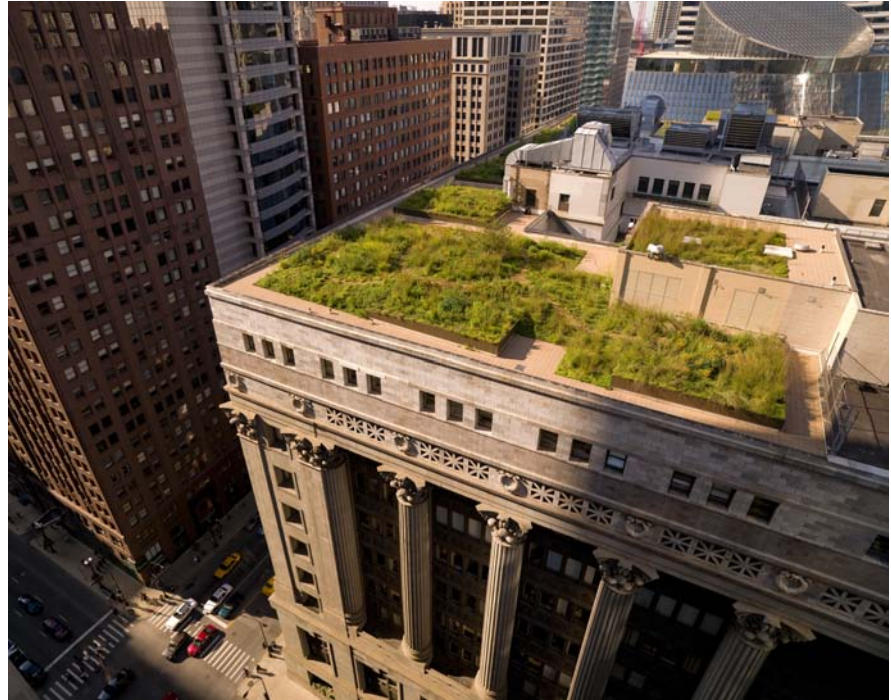
Figure 8.4 A roof garden on the Chicago City Hall containing over 20,000 plants and more than 150 species. (Source: City of Chicago)
