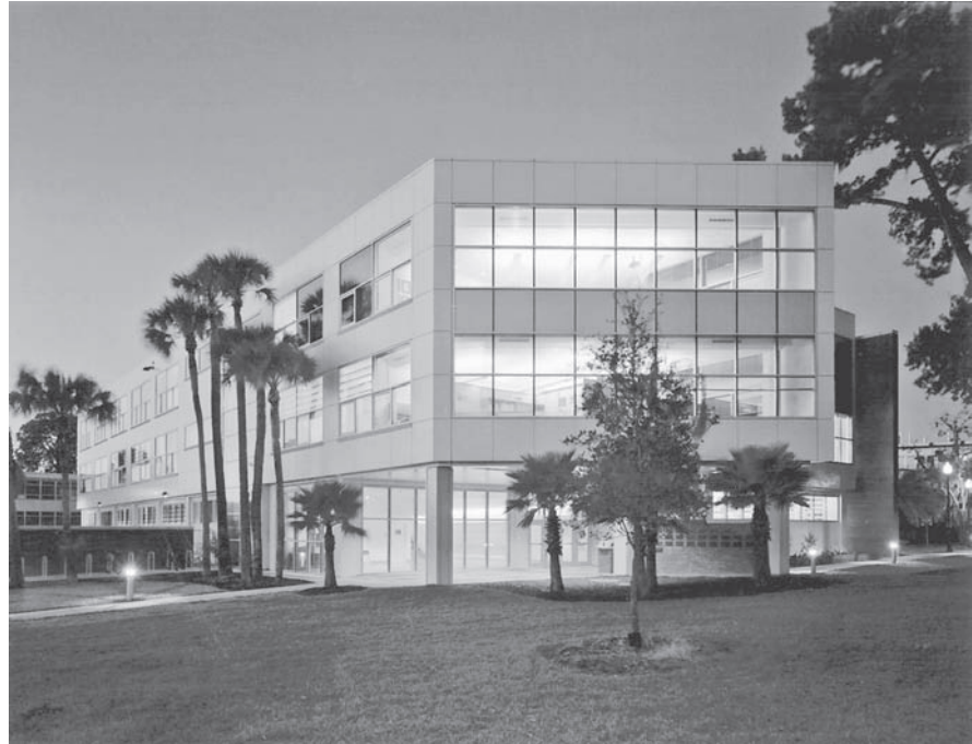
Figure 8.11 The exterior lighting system for Rinker Hall, a LEED-NC gold certified building at the University of Florida in Gainesville, was designed to minimize light pollution. The result is a pleasant evening view of the building that enhances the experience of passersby. (Photograph courtesy of Gould Evans Associates and Timothy Hursley)
