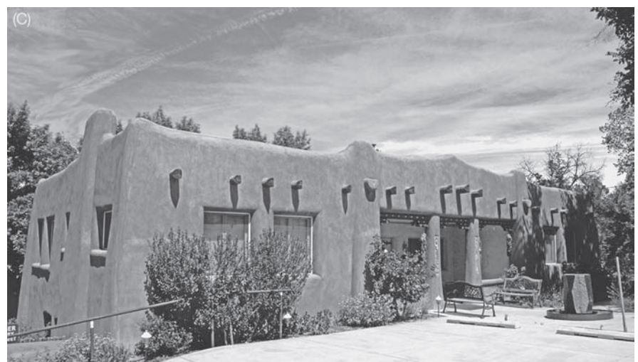
Figure 15.8 Examples of New Mexico adobe architecture. (A) As early as 350 AD, the Anasazi, the oldest-known inhabitants of New Mexico, began to build aboveground masonry structures, the foundations of which are visible here at the base of their cliff dwellings in Bandelier National Park. (B) Communities called pueblos flourished around 1250–1300 AD and contained intricate arrays of connected flat-roofed, multilevel adobe buildings. (C) A modern office building in Santa Fe, New Mexico, retains the appeal and function of traditional adobe architecture.
