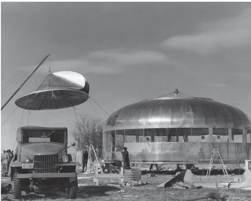
Figure 3.3 R. Buckminster Fuller’s Dynamic Maximum Tension, or Dymaxion House, in Wichita, Kansas, was the first serious attempt to create an autonomous house. It was designed for mass production, weighed just 3000 pounds (1364 kilograms) compared to the 150 tons (137 metric tons) of a typical house, featured a built-in wind turbine for generating power, and had a graywater system. (Courtesy, The Estate of R. Buckminster Fuller)
