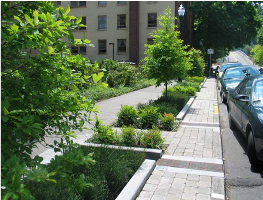
Figure 10.17 Several components are integrated into this sustainable stormwater management system in Portland, Oregon. All constraints and benefits are considered when selecting which components to use for any given site. (Source: City of Portland, Oregon)
