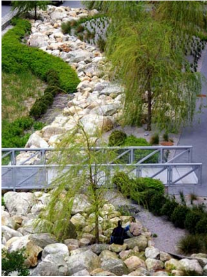
Figure 8.8 The stormwater bioretention system for the Stata Center, a Frank Gehry–designed building on the Massachusetts Institute of Technology campus in Cambridge, Massachusetts, is a multifunctional constructed wetland that detains runoff to reduce peak downstream flow. The plants and planting medium of the wetland clean the runoff and allow some groundwater infiltration. (Photo by Stuart Patton Echols)
