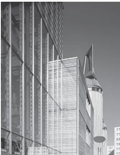
Figure 9.7 Wind catcher (upper right) on the Jubilee Campus of the University of Nottingham in the United Kingdom. The wind catcher pivots in the wind, with the vane indicating the direction of airflow. Wind flowing past the vane induces the convection of air through the structure. (Photograph courtesy of Hopkins Architects and Ian Lawson)
