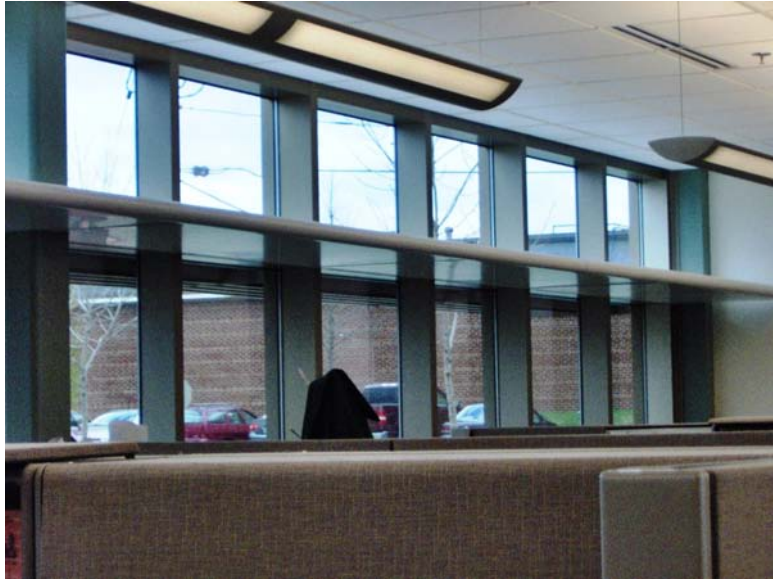
Figure 12.2 (C) A light shelf allows sunlight in while protecting users from glare that is often associated with tall windows. (Decorating with Fabric)
