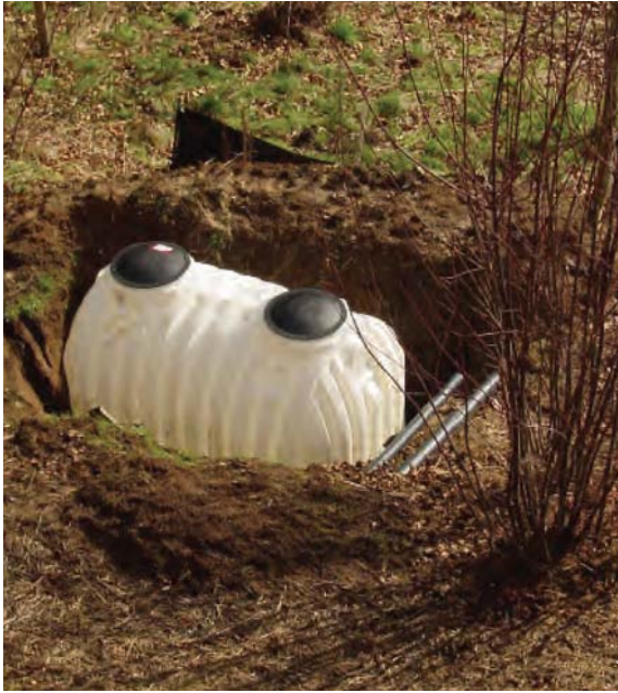
Figure 10.16 (C) Cisterns are similar to rain barrels except they are more permanent and constructed with more durable material. They can be installed above or beneath the ground, with sizes ranging from 100 to 10,000 gallons. (Source: City of Portland, Oregon)
