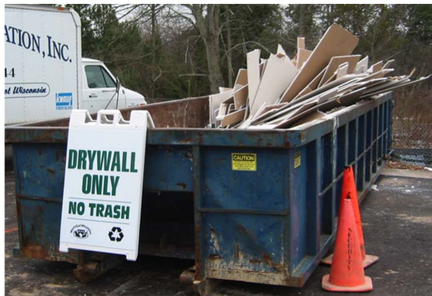
Figure 13.7 Example of proper waste separation to enhance the potential for materials reuse. (WasteCap Resource Solutions, Milwaukee, WI)
