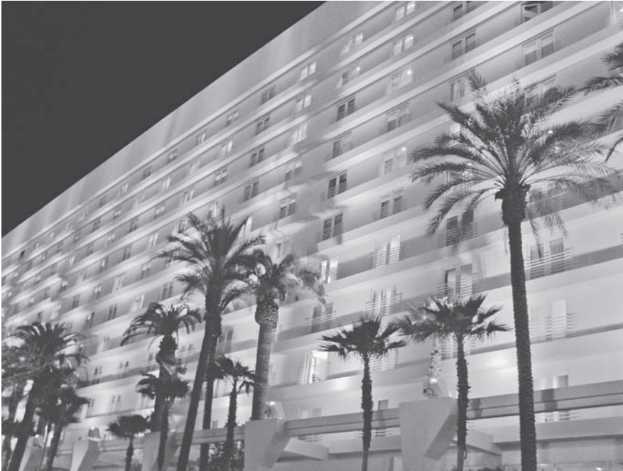
Figure 9.21 An intelligent LED lighting system by Color Kinetics and 4 Wall Entertainment illuminates the exterior of the Hard Rock Hotel and Casino in Las Vegas, Nevada, cutting annual energy costs by 90 percent. (Photograph courtesy of 4Wall Entertainment)
