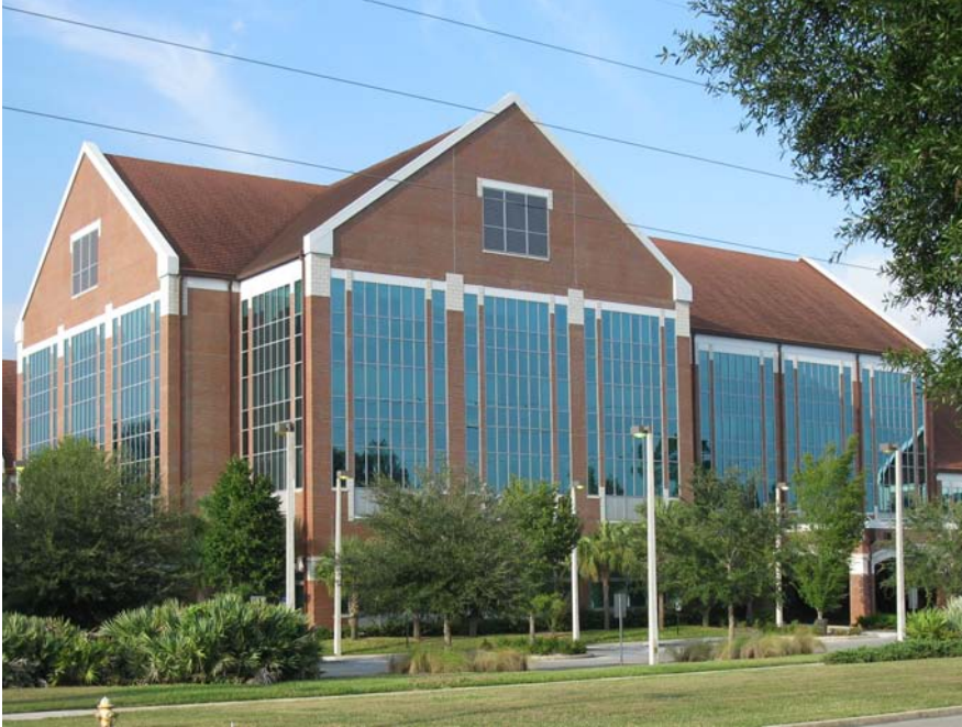
Figure 7.1 The project team for the Orthopaedics and Sports Medicine Institute at the University of Florida in Gainesville used the design-build delivery system to deliver this LEED-certified green building. (T. Wyman)
