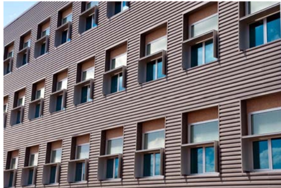
Figure 1.9 (D) The fenestration for the NREL RSF was designed to provide excellent daylighting while controlling glare and unwanted solar thermal gain through the use of shading devices, recessed windows, and electrochromic glass. Operable windows allow the occupants to control their thermal comfort and obtain fresh air. (Source: National Renewable Energy Laboratory)
