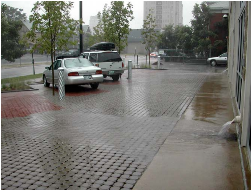
Figure 10.16 (K) Pervious pavers or unit pavers replace impervious surfaces and allow stormwater to soak into the ground. They typically are made out of precast concrete, brick, stone, or cobbles and form interlocking patterns with the gaps filled with either sand or gravel. (Photograph courtesy of Holly Piza)
