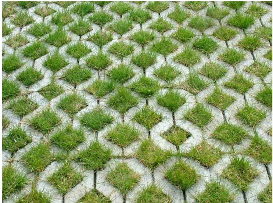
Figure 10.16 (M) Turf block, also known as grass grid or open-cell unit pavers , has gaps filled with soil and grasses allowing water to pass through. This option only accepts precipitate and not stormwater runoff; thus, suited for low traffic and infrequent car parking. Applications include patios, walkways, emergency access roads, street shoulders, and residential driveways. (Photograph courtesy of Western Interlock, Inc.)
