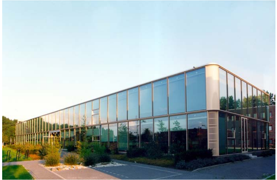
Figure 11.11 (A) The XX Office Building located in Delftech Park in Delft, Netherlands, has a ceiling-to-floor rectangular glass façade. Standard-sized glazing will be reused after the building is deconstructed. (J. M. Post, XX Architecten)
