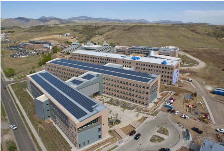
Figure 1.9 (A) The NREL Research Support Facility in Golden, Colorado, is a four-story NZE building that combines low-energy design with high-efficiency photovoltaics to produce all the energy it requires over the course of a year. (Source: National Renewable Energy Laboratory)
