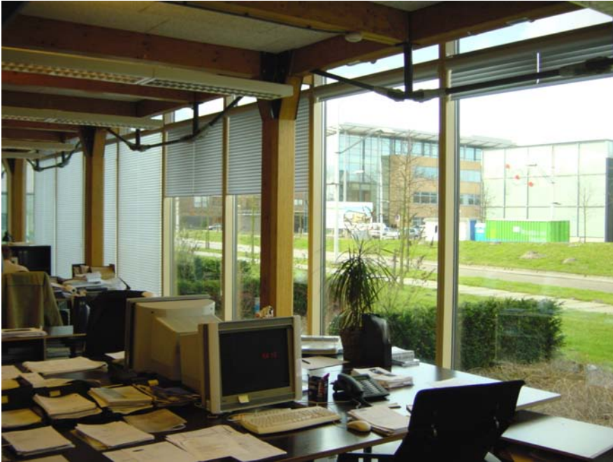
Figure 11.11 (C) The columns and beams in a completed office, are exposed and connected by stand-off steel rod lower chords and bolts to promote ease of construction and deconstruction. (J. M. Post, XX Architecten)
