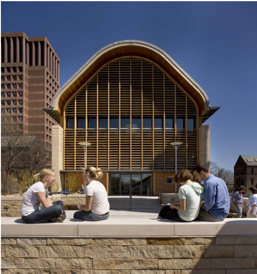
Figure 1.10 (D) The south side of the building is recessed, and window overhangs are integrated into the façade of the building to control glare and thermal loads while maximizing daylighting. (Photograph by Morley Von Sternberg)
