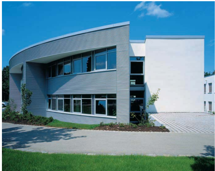
Figure 2.17 The signature exterior of OWP 11 in Stuttgart, Germany, is its metal façade, which is the outer layer of a well-insulated wall system that reduces internal heating and cooling loads to very low levels. (© Dietmar Strauß, Besigheim, Germany, and © Martin Duckek, Ulm, Germany)
