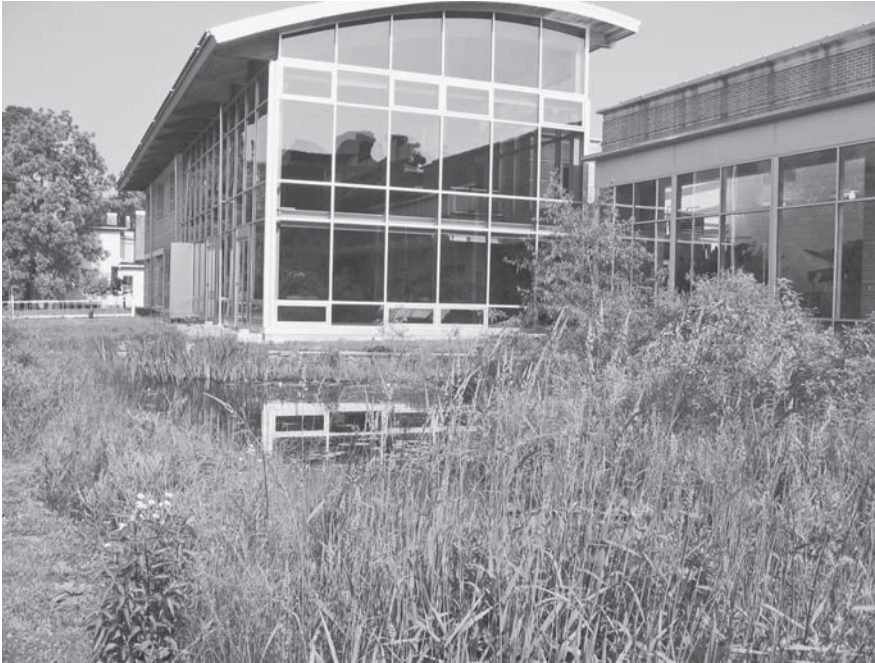
Figure 10.15 The Living Machine built into the Lewis Center for Environmental Studies at Oberlin College in Oberlin, Ohio, contains biological organisms that break down wastewater components into nutrients that are then fed into a constructed wetland inside the building. (Photograph courtesy of Oberlin College)
