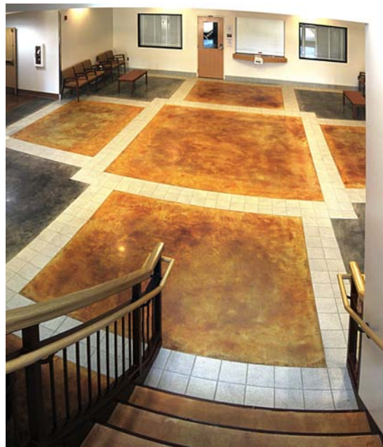
Figure 6.7 Polished, stained concrete floors were specified instead of far less durable floor coverings. These provide a long-lasting, very attractive option and reduce the quantity of materials needed for construction. (Photograph courtesy of Glen Roberts, St. Johns River State College)
