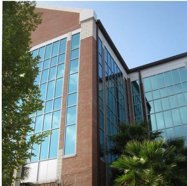
Figure 9.14 Low-E glazing on the Orthopaedics and Sports Medicine Institute at the University of Florida in Gainesville. The advent of high-technology glazing allows the design of buildings that admit visible light for daylighting but reflect infrared radiation. DOE-2.1 and daylighting simulations confirmed that daylighting and low-E glass produced greater savings than focusing solely on the thermal resistance of the building envelope. (T. Wyman)
