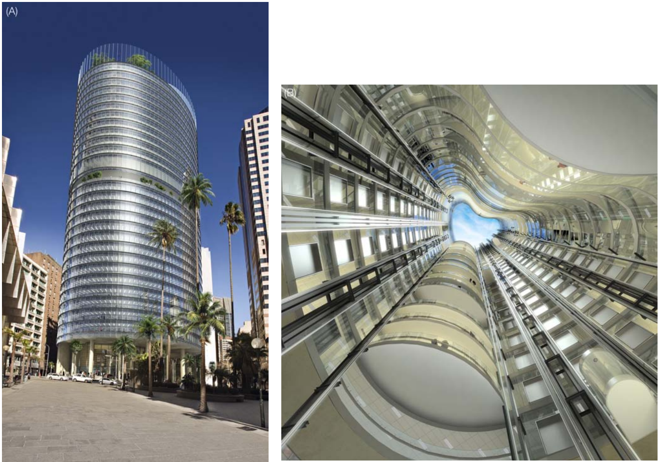
Figure 4.8 (A) The property at 1 Bligh Street in Sydney, Australia, is one of the most advanced buildings in the world, with a double-skin façade, solar-powered air-conditioning system, and a blackwater recycling system. (B) The naturally ventilated 28-story atrium assists in providing spectacular daylighting for all floors. [Images supplied courtesy of ingenhoven + architectus (Sydney)]
