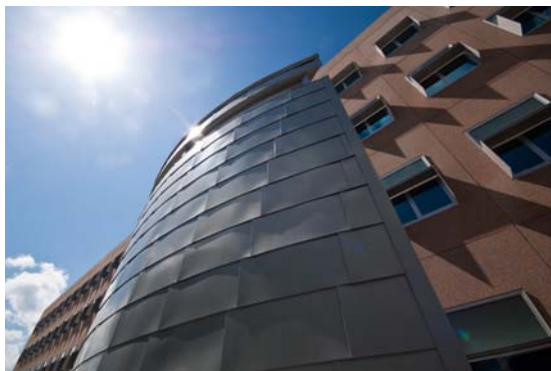
Figure 1.9 (B) Ground view of the air intake structure that conducts outside air into the thermal storage labyrinth in the crawl space of the NREL RSF. (Source: National Renewable Energy Laboratory)
