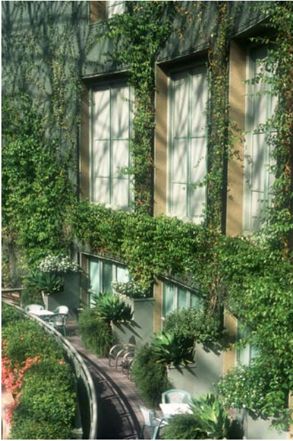
Figure 8.6 A vertical landscape at Universal City Walk in Universal City, California, provides a changing evergreen façade, which extends to a height of 75 feet (23 meters). (greenscreen®)
