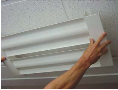
Figure 9.35 Chilled-beam systems are aluminum-finned copper assemblies through which water circulates, providing radiative cooling or heating and inducing airflow by convective effects. (Courtesy of Interface Engineering)
