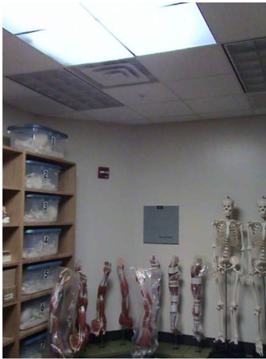
Figure 6.8 A storage room on the second floor of the Health Sciences Building uses natural light that is projected into the room through solar tubes installed on the roof. (D. Stephany)
