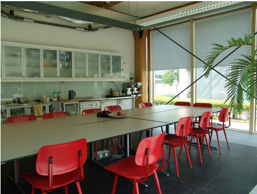
Figure 11.11 (D) Ceiling-to-floor window screens control the amount of daylight entering the building. (J. M. Post, XX Architecten)
