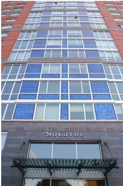
Figure 9.25 BIPVs in the Solaire building in New York City's Battery Park. The BIPVs are the speckled surfaces between the windows. (Photograph courtesy of the Albanese Development Corporation)
