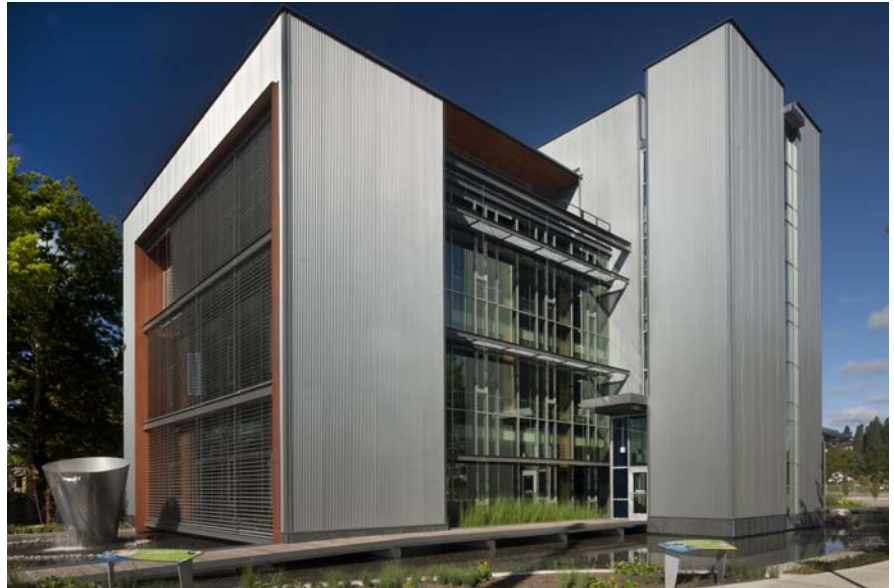
Figure 10.19 (A) The new Regional Services Center for Olympia's LOTT Clean Water Alliance stands as an icon in the neighborhood and welcomes the public for hands-on water treatment education. A reclaimed water pond edges two sides of the building, enticing visitors to become engaged in the process. (© Nic Lehoux)
