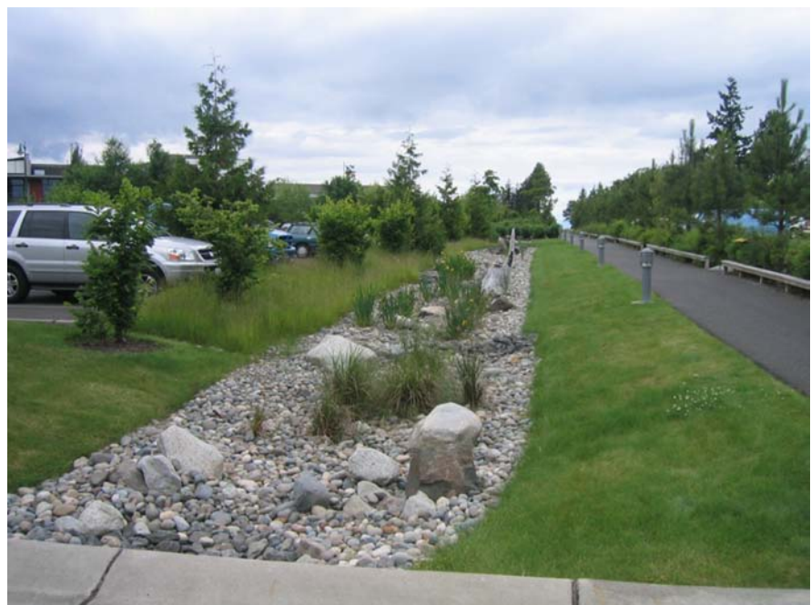
Figure 8.9 The stormwater system design for Chambers, Washington, employs a long water trail that exhibits a variety of water treatments. These include a wetland and a lined bed with river stone and plants interspersed with pieces of driftwood to emphasize the water theme. (Photo by Stuart Patton Echols)
