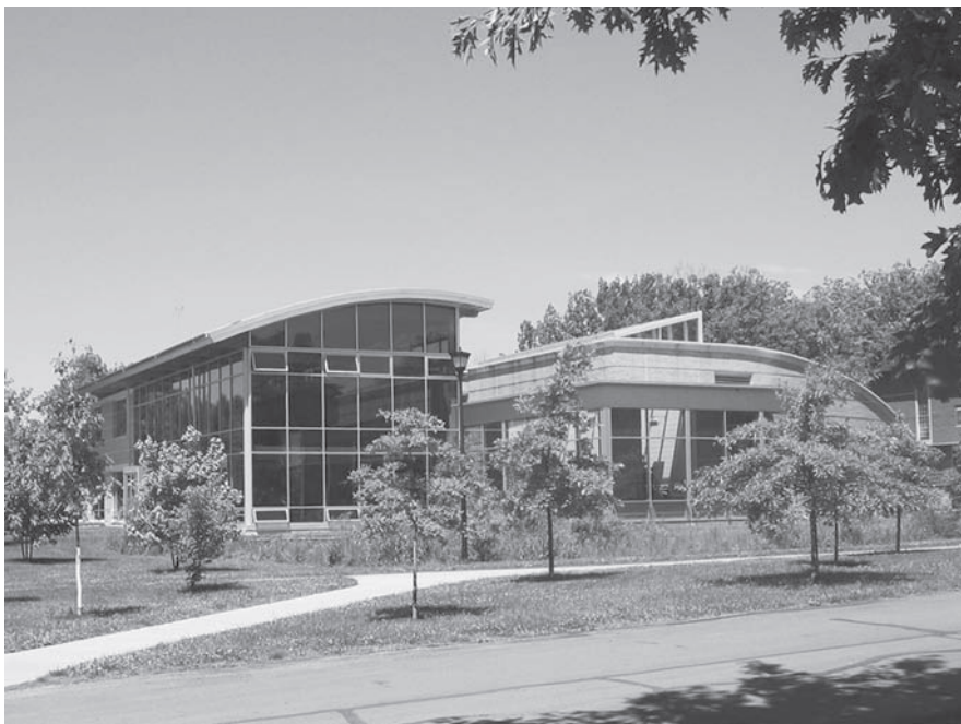
Figure 1.8 The Lewis Center for Environmental Studies at Oberlin College in Oberlin, Ohio, was designed by a team led by William McDonough, a leading green building architect, and including John Todd, developer of the Living Machine. In addition to the superb design of the building's hydrologic strategy, the extensive photovoltaic system makes it an NZE building. (Photograph courtesy of Oberlin College)
