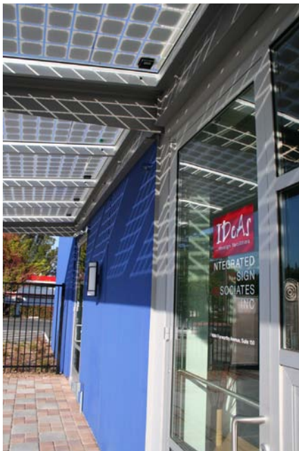
Figure 9.17 The IDeAs Z 2 office building in San Jose, California, is an NZE facility that was achievable through well-conceived approaches to reducing plug loads and upsizing electrical wiring.
