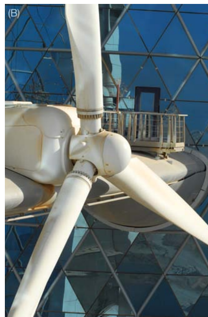
Figure 9.26 Three wind turbines, each 29 meters in diameter, provide 10 to 15 percent of the power needed to operate the Bahrain World Trade Center, which opened in 2007 in Manama, Bahrain. (Courtesy of Atkins)
