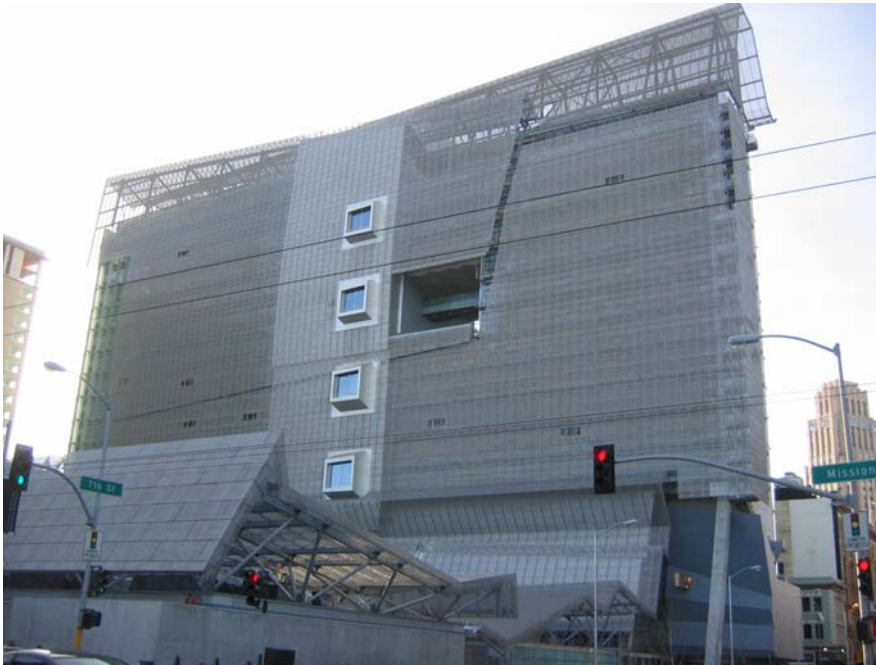
Figure 15.2 The folded, perforated metal skin covering portions of the San Francisco Federal Building assists in the flow of air through the structure and provides an interesting and appealing appearance for the structure, both at the ground level and at the upper façade. (Photograph courtesy of Jenna Hildebrand)
