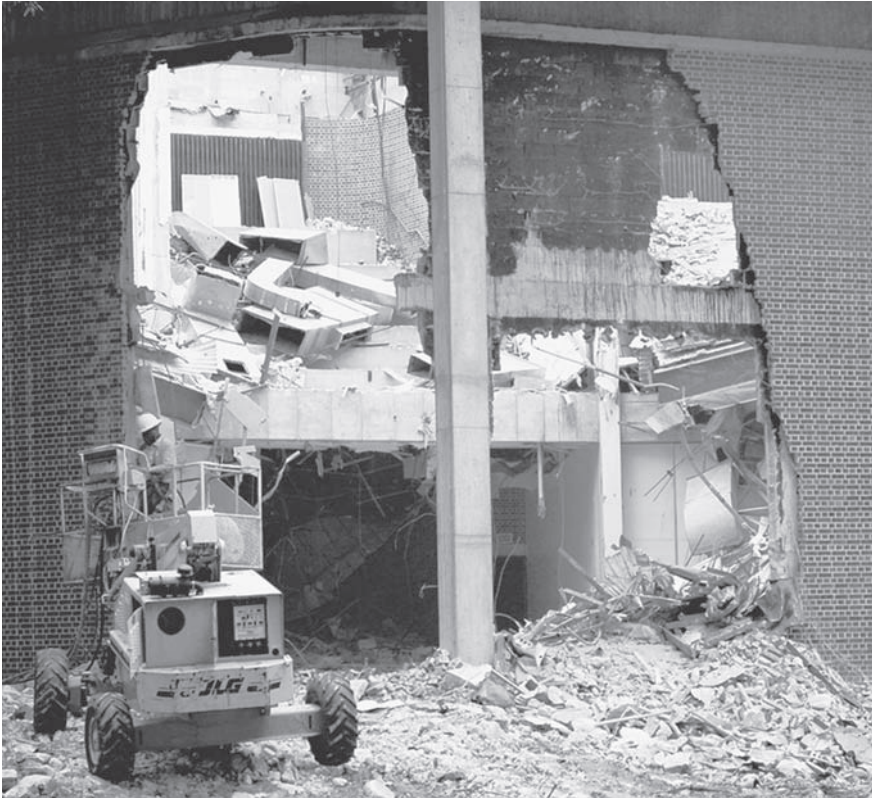
Figure 2.9 Annual construction and demolition waste in the United States is estimated to be about 160 million tons (145 million metric tons), or about one-half ton per capita. Buildings are not generally designed to be disassembled, and the result is that only a small percentage of demolition materials can be recycled. The partial demolition of the Levin College of Law library at the University of Florida in Gainesville in mid-2004 illustrates the quantities of waste typically generated in renovation projects, on the order of 70 to 100 pounds per square foot (344 to 489 kilograms per square meter). (Photograph courtesy of M. R. Moretti)
