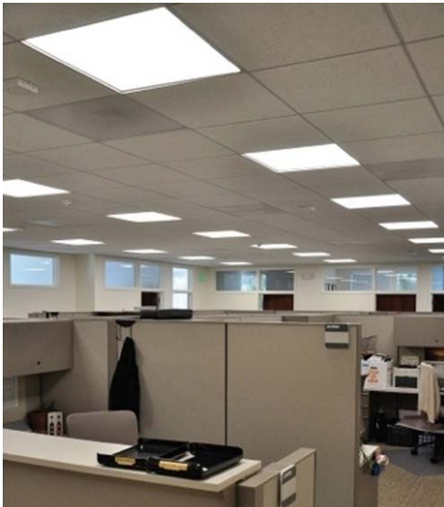
Figure 9.22 LED lighting is now available as architectural grid lay-in lighting that measures 2 feet by 2 feet. (Photograph courtesy of Lunera Lighting, Inc.)
