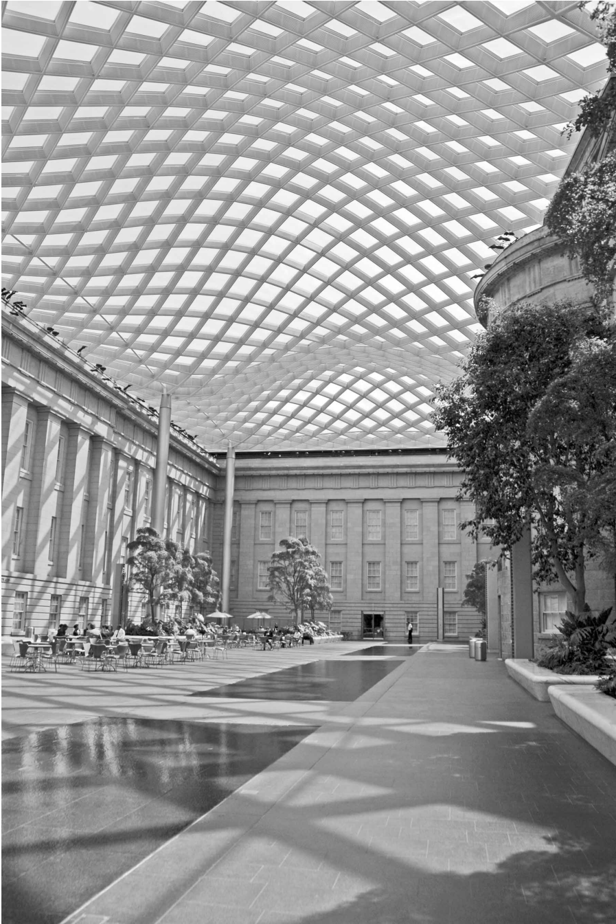
FIGURE 35. THE ROBERT AND ARLENE KOGOD COURTYARD, NATIONAL PORTRAIT GALLERY, WASHINGTON, D.C. (2007). FOSTER + PARTNERS, LONDON. (Courtesy Magenta Livengood.) The undulating roof of 864 glass panels floods a 28,000-square-foot interior public courtyard with daylight. Multiple coatings on the glass prevent the ultraviolet rays from entering and making the space expensive to air condition. The ceiling reflects people and events at night, creating an enlivened atmosphere with images that bounce between the glass and the shallow basins of water.
