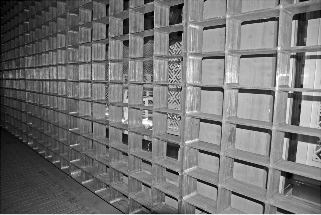
FIGURE 75. BLUR BUSINESS HOTEL AND CULTURAL FACILITY, BEIJING, CHINA (2006). STUDIO PEI-ZHU, BEIJING. (Courtesy Magenta Livengood.) Walls made of fiber-reinforced polymer plastic (FRP) hang off a retained existing concrete structure. The semi-transparent panel façade glows at night, providing a beacon-like lantern of subtle attraction that is compatible with the historic district near the Forbidden City.
