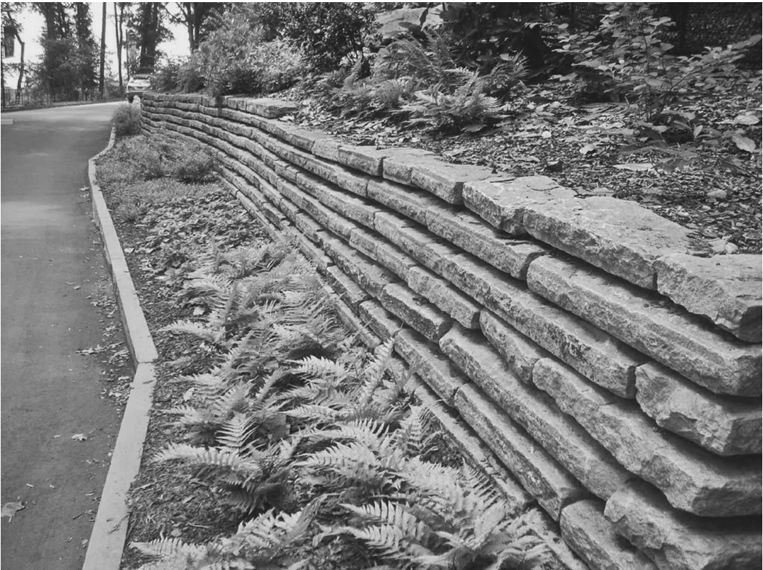
FIGURE 47. ATLANTA BOTANICAL GARDEN, ATLANTA, GEORGIA (2009). AECOM, ALEXANDRIA, VIRGINIA. (© AECOM.) Granite curbs were salvaged from an existing road to be demolished. They were repurposed in the garden as dry stacked retaining walls.
