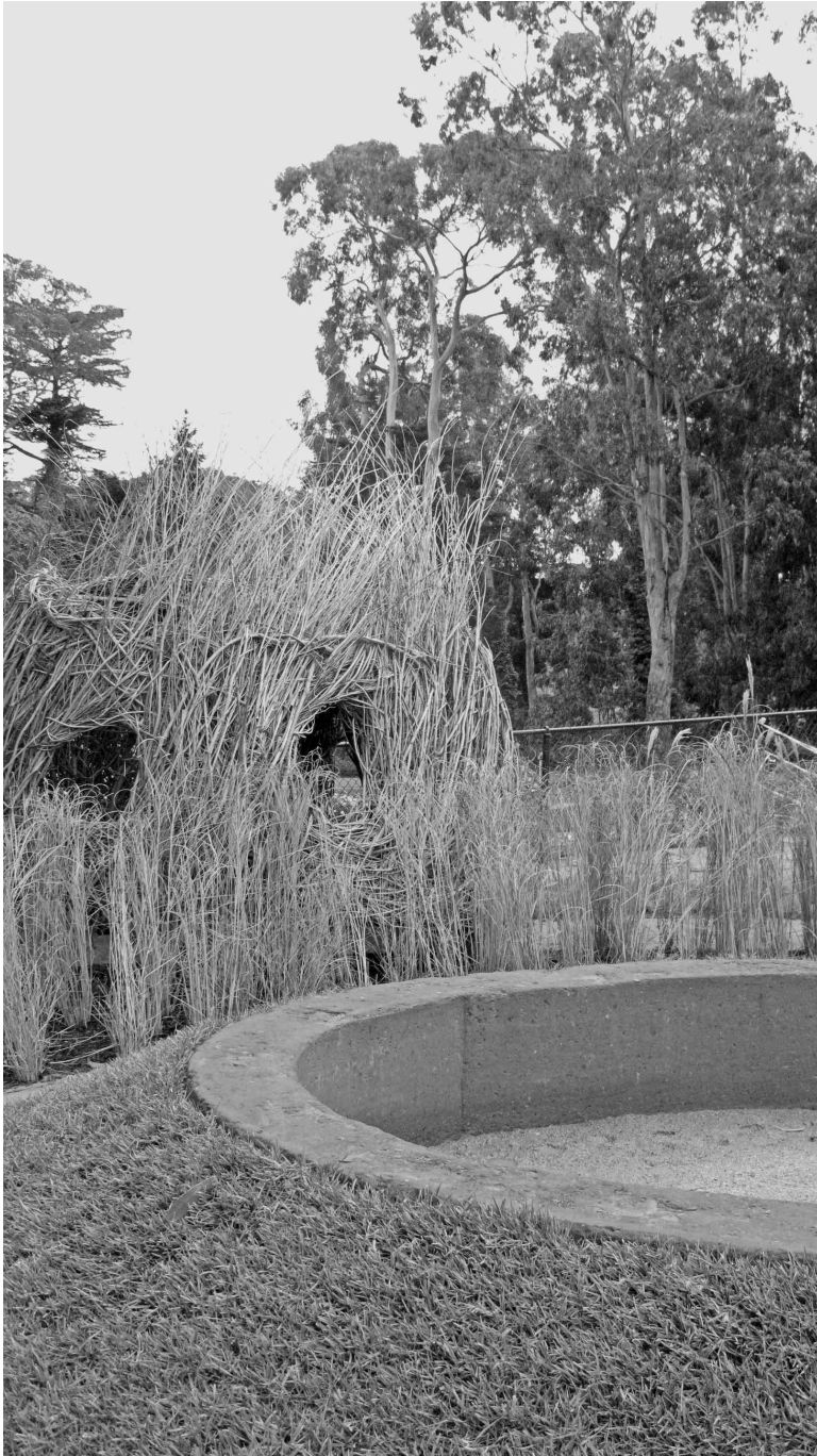
FIGURE 65. COW HOLLOW PLAYGROUND, PRESIDIO, SAN FRANCISCO (2009). SURFACEDSIGN, INC., SAN FRANCISCO. (Courtesy Roderick Wyllie.) Permanent construction is not allowed on the historic Presidio grounds and no footing depth can exceed eighteen inches, making rammed earth a suitable material and construction technique for the seat wall. The earthen wall and sand-colored decomposed granite paving surface unite two materials ideal for kid-friendly durability.
