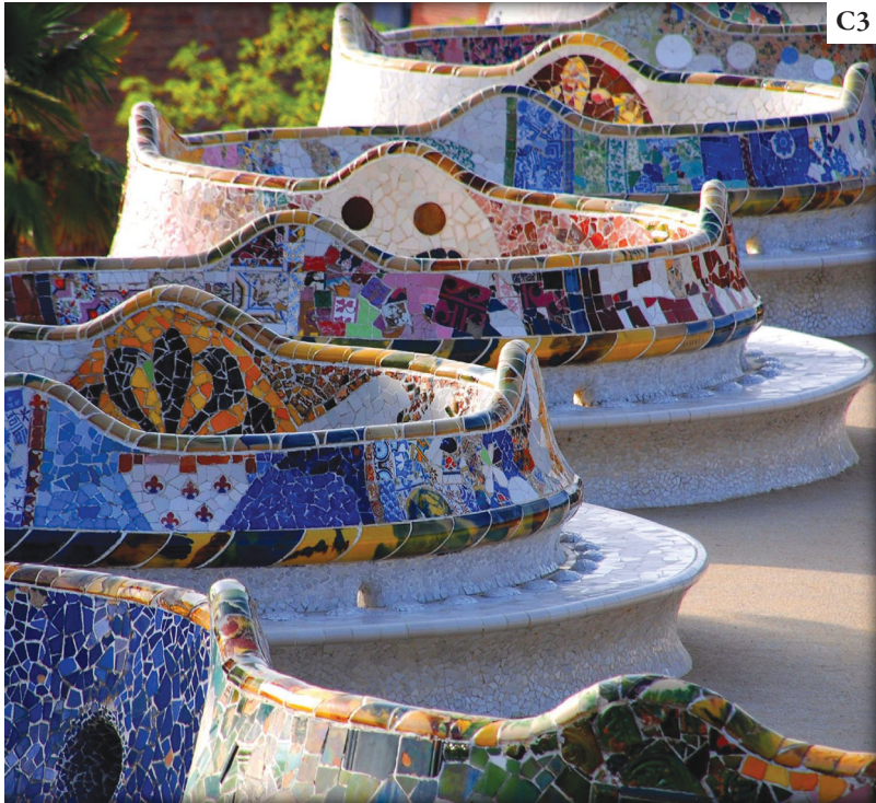
FIGURE 31. GÜELL PARK, BARCELONA (1900–1914). ANTONIO GAUDÍ, BARCELONA. (Courtesy Franz St., Austria.) The elevated terrace in the center of the park has a serpentine-shaped edge with a continuous railing and bench covered in broken multicolored ceramic tile in a mosaic technique called trencadís . This project became a UNESCO World Heritage Site in 1984.
