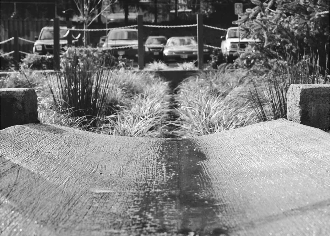
FIGURE 5. MOUNT TABOR MIDDLE SCHOOL RAIN GARDEN, PORTLAND, OREGON (2006). KEVIN ROBERT PERRY, CITY OF PORTLAND, OREGON. (Courtesy Kevin Robert Perry.) The striated finish of the concrete water basin captures the idea of water when dry as well as directing the flow in the rain.
