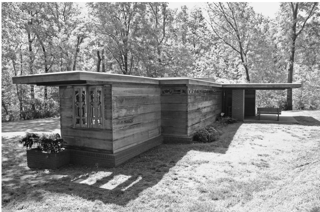
FIGURE 58. POPE-LEIGHEY HOUSE, ALEXANDRIA, VIRGINIA (1939). FRANK LLOYD WRIGHT, TALIESIN, WISCONSIN. (Courtesy Magenta Livengood.) The original cypress siding survives even though the house has been disassembled and relocated. The original wood beams for the roof cantilevers have been replaced with steel.
