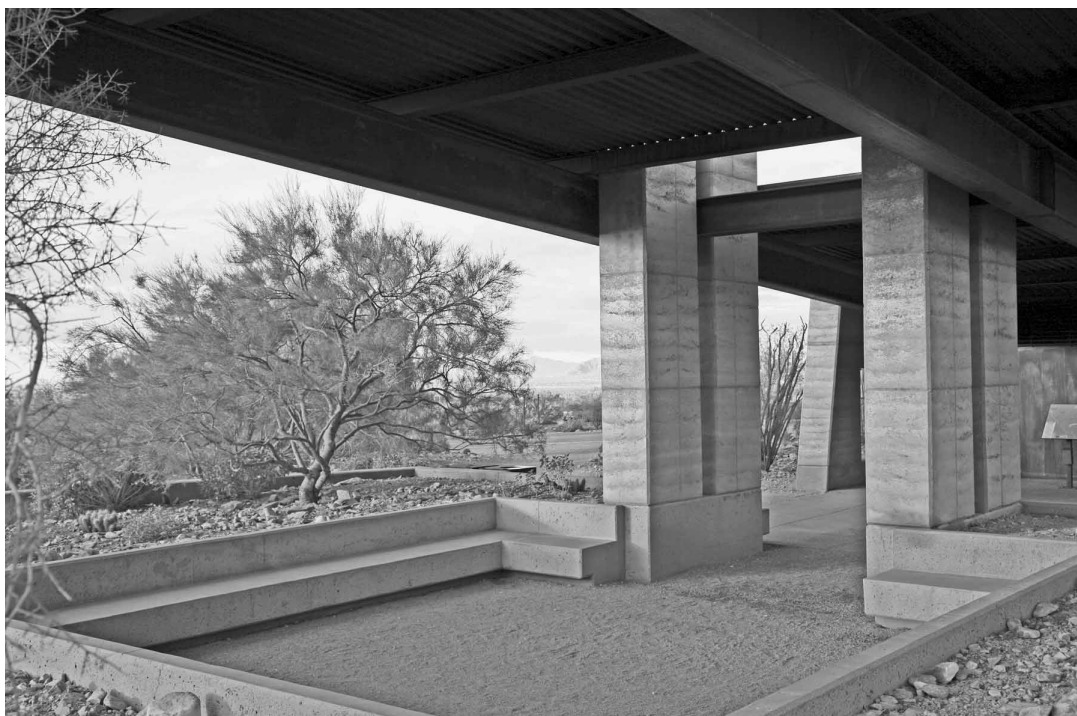
FIGURE 4. McDOWELL SONORAN PRESERVE TRAILHEAD, LOST DOG WASH, OUTDOOR CLASSROOM, SCOTTSDALE, ARIZONA (2006). WEDDLE GILMORE ARCHITECTS, SCOTTSDALE, ARIZONA, AND FLOOR ASSOCIATES, INC., PHOENIX, ARIZONA, LANDSCAPE ARCHITECTS. (© Bill Timmerman.) Pre-cast concrete benches serve as retaining walls, and their form and smooth surfaces invite sitting. The finish contrasts with the rammed-earth columns and rugged landscape of the Sonoran desert. The building incorporates many sustainable elements, including photovoltaic cells, composting toilets, grey water systems, and rainwater conservation and harvesting for irrigation.
