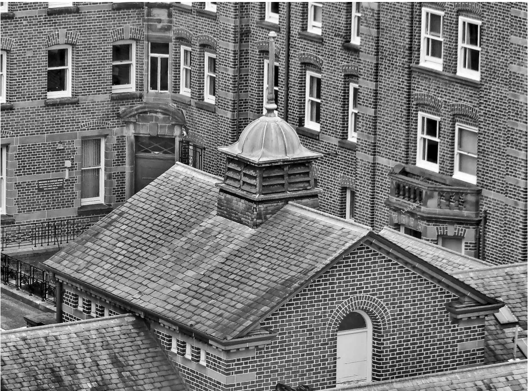
FIGURE 68. ROYAL VICTORIA HOSPITAL, BELFAST, NORTHERN IRELAND (1906). W. HENMAN AND T. COOPER, BIRMINGHAM. (Courtesy John D. McDonald.) The first major public building designed to be mechanically air conditioned had tall ceilings and thin wings, allowing the natural daylight to penetrate deep inside the building and avoiding the need for heat-producing artificial lighting during the day. Small buildings housed the mechanical fans that moved the air through wet hanging strips of fabric to dedicated chambers that circulated the cooler air throughout the building (Banham 1969, 82–83).
