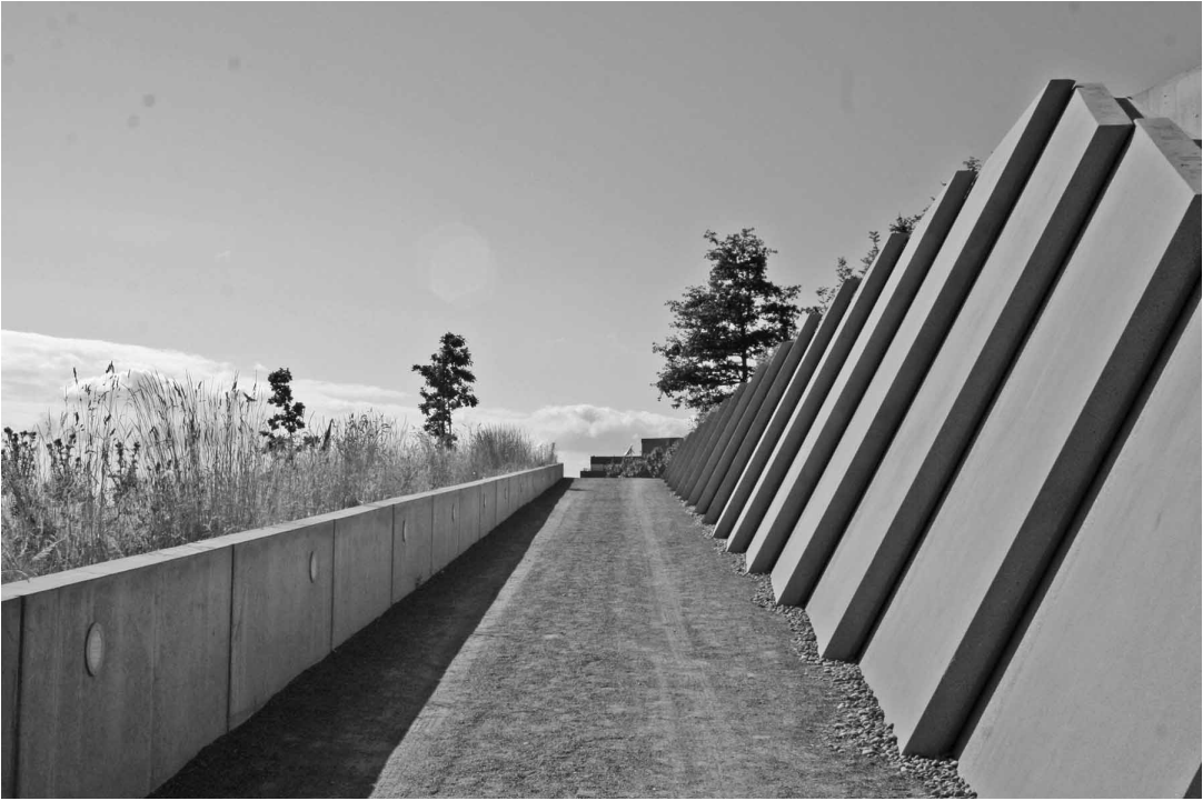
FIGURE 7. OLYMPIC SCULPTURE PARK, SEATTLE ART MUSEUM, SEATTLE, WASHINGTON (2007). WEISS/MANFREDI, ARCHITECTS, NEW YORK. (Photograph by Brett Weidl. Courtesy Hoerr Schaudt Landscape Architects.) Staggered pre-cast concrete panels cover gabion retaining walls. Their overlapping assembly and sloped position take advantage of its form, allowing the thickness of the concrete to be minimized. The wall extends to a highway embankment, where the pattern is especially interesting at night when car headlights cast a bright light on the panels otherwise in shadow, and the illuminated edges follow the passing movement.
