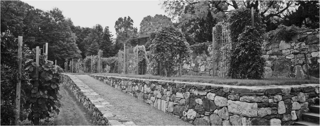
FIGURE 44. M. VICTOR AND FRANCES LEVENTRITT GARDEN AT THE ARNOLD ARBORETUM, HARVARD UNIVERSITY, BOSTON (1998). REED | HILDERBRAND LLC, WATERTOWN, MASSACHUSETTS. (Photograph by Alan Ward. Courtesy Jeri Reed | Hilderbrand.) Fieldstone retaining walls level the land and refer to New England’s history of cleared farm fields edged with dry stone fences.
