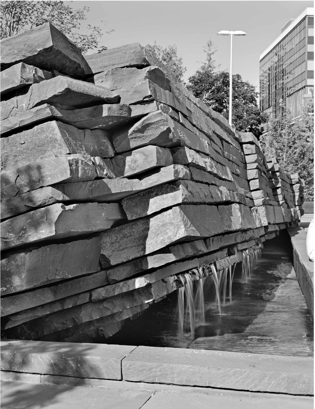
FIGURE 46. BAILEY PLAZA, CORNELL UNIVERSITY, ITHACA, NEW YORK (2004–2007). MICHAEL VAN VALKENBURGH ASSOCIATES, INC., LANDSCAPE ARCHITECTS, P.C., CAMBRIDGE/NEW YORK. (Photograph by Elizabeth Felicella. Courtesy Michael van Valkenburgh Associates.) The campus is surrounded by glacially formed gorges. The plaza used local stone alternating between thermal-flamed Portage bluestone and natural cleft bluestone to achieve an intimate scale with the range of textures and colors. The fountain stone is laid with gaps so that the water can fall into the basin, enhancing a feeling of contemplation and repose.
