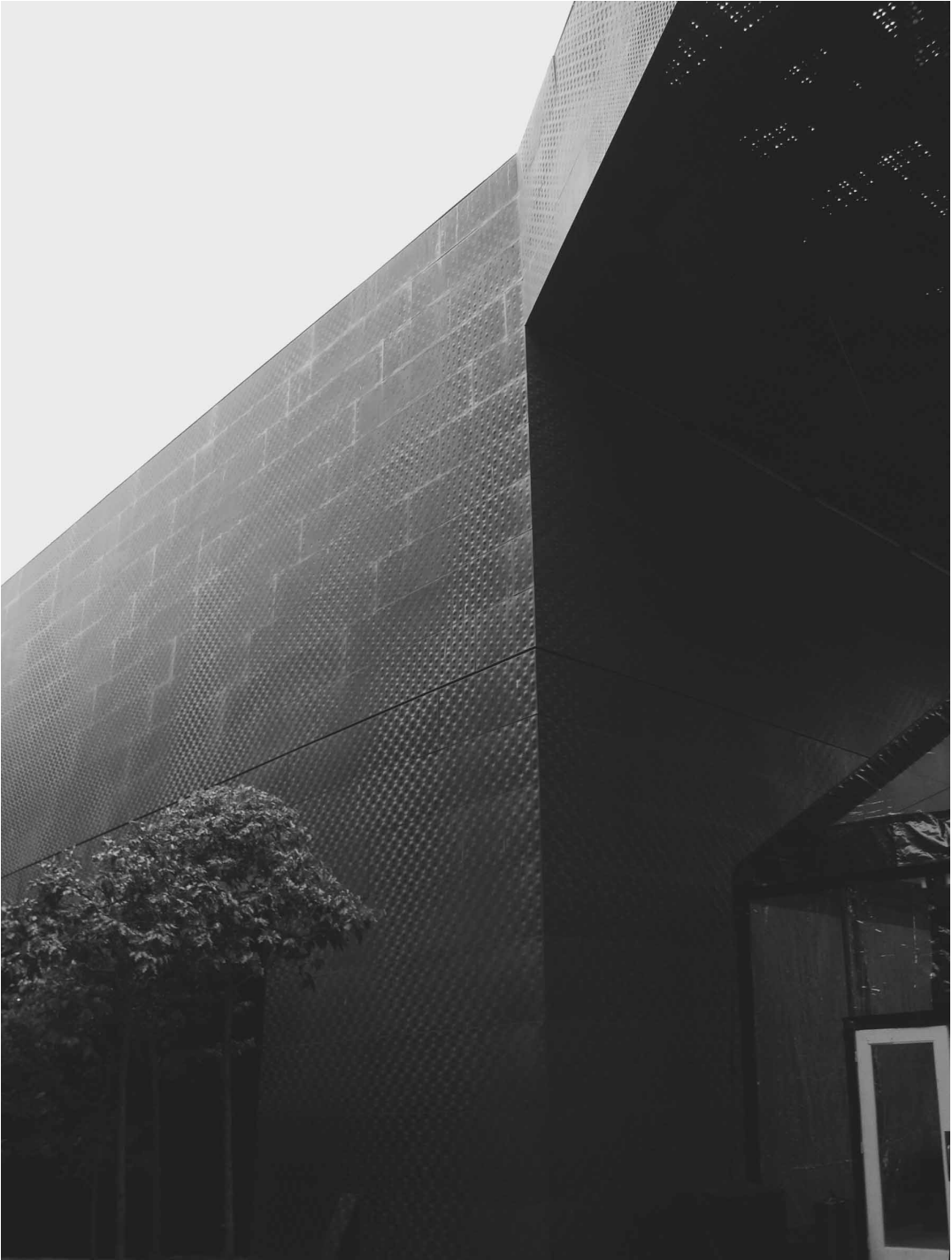
FIGURE 19. M. H. DE YOUNG MEMORIAL MUSEUM, SAN FRANCISCO (2005). HERZOG & DE MEURON, BASEL. (Courtesy Magenta Livengood.) Thin oxidized copper panels, variably perforated and dimpled, are used to enclose space to varying degrees and to provide a backdrop to the native eucalyptus trees.
