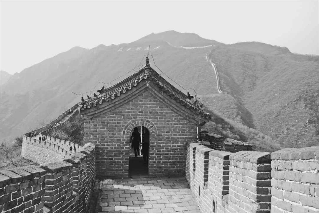
FIGURE 24. GREAT WALL OF CHINA, NORTHERN BORDER, CHINA (FROM THE SEVENTH CENTURY BCE, WITH THE MAJORITY OF THE WALL RECONSTRUCTED DURING THE MING DYNASTY [1368–1644], WITH ONGOING REPAIR). (Courtesy Magenta Livengood.) The wall and guardhouse structures were constructed of stone and brick over rammed and tamped earth infill. It became a UNESCO World Heritage Site in 1987.
