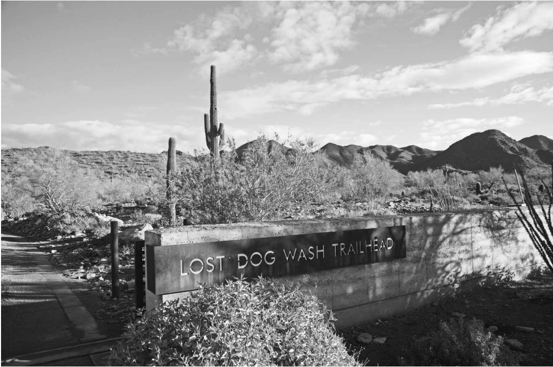
FIGURE 61. MCDOWELL SONORAN PRESERVE, LOST DOG WASH TRAILHEAD SIGN, SCOTTSDALE, ARIZONA (2006). WEDDLE GILMORE ARCHITECTS, SCOTTSDALE, ARIZONA, AND FLOOR ASSOCIATES, INC., PHOENIX, ARIZONA, LANDSCAPE ARCHITECTS. (Photograph © Bill Timmerman.) The rammed-earth wall takes advantage of local soils, and the colors and textures blend with the surrounding desert landscape.
