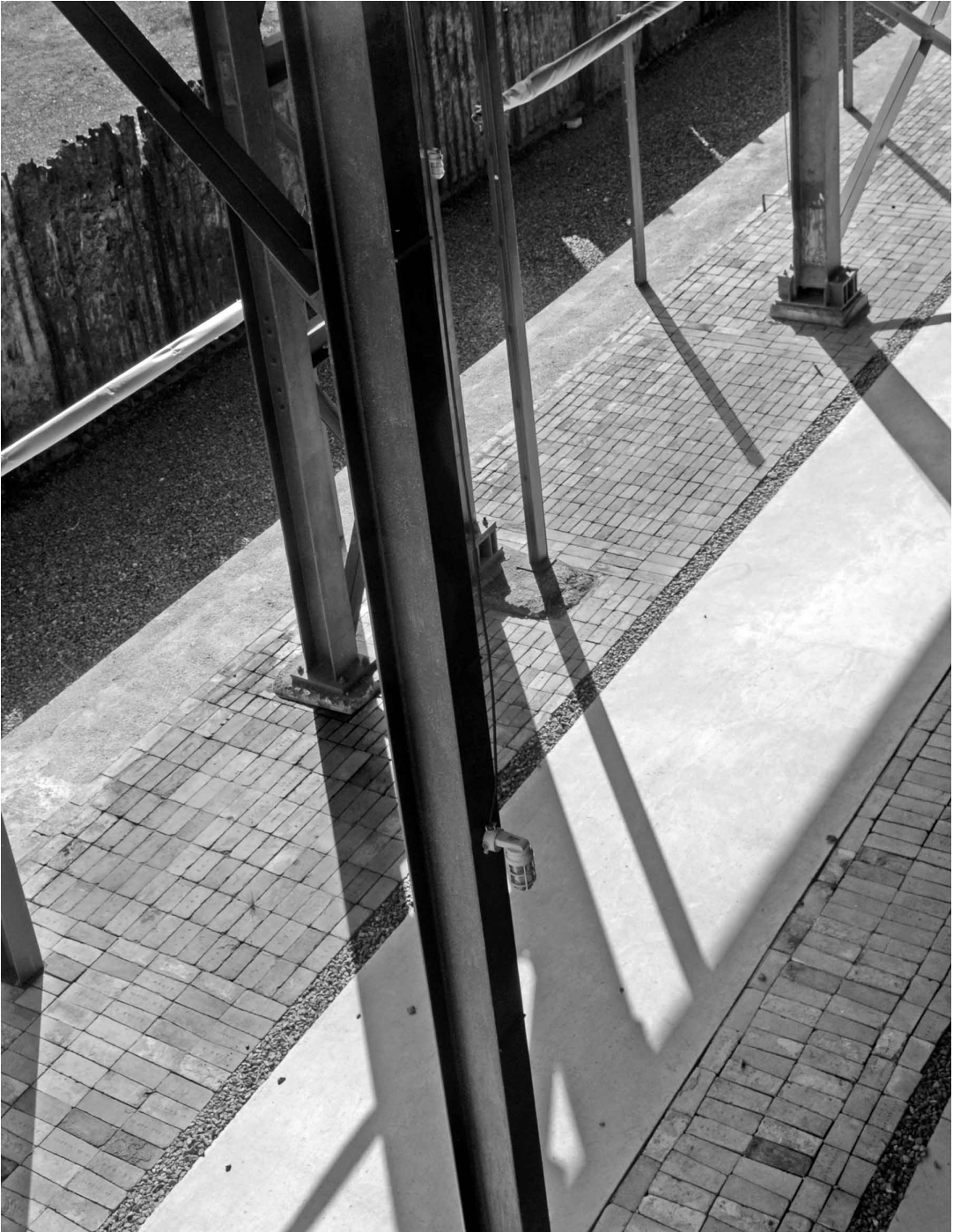
FIGURE 22. MUSEO DEL ACERO HORNO (MUSEUM OF STEEL), MONTERREY, MEXICO (2007). SURFACEDESIGN, INC., SAN FRANCISCO, AND HARARI ARQUITECTOS. (Courtesy James A. Lord.) Refractory bricks from the decommissioned blast furnace were downgraded and repurposed as a surface paving material.
