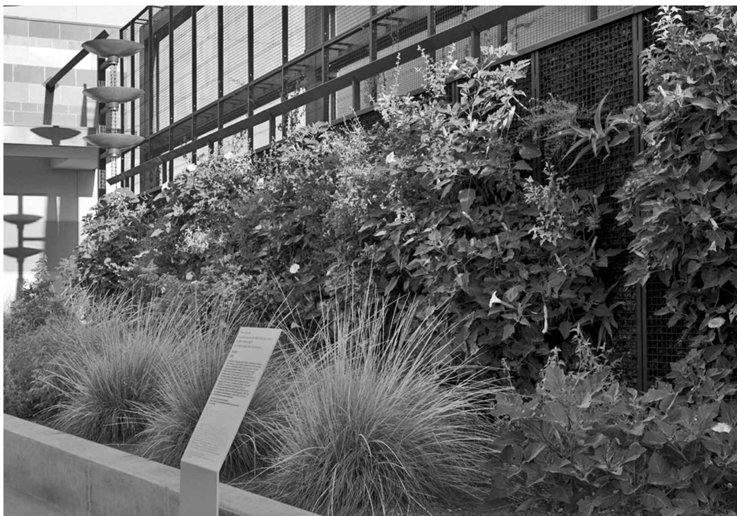
FIGURE 78. PHOENIX CONVENTION CENTER, PHOENIX (2011). TEN EYCK LANDSCAPE ARCHITECTS, PHOENIX. (© Bill Timmerman.) The 1,400-square-foot living wall uses air-conditioning condensate that is UV treated and purified to irrigate the plants. It is also a screen, blocking views of the parking garage at street level.
