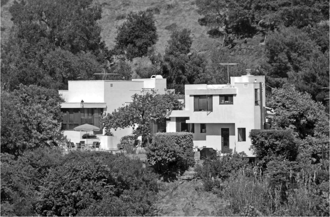
FIGURE 67. LOVELL HEALTH HOUSE, LOS ANGELES (1927–1928). RICHARD NEUTRA, LOS ANGELES. (Courtesy Magenta Livengood.) This was the first steel-frame house in the United States. Neutra conducted extensive research leading to a design that incorporated passive ventilation, among other elements and systems now considered essential for sustainable design.
