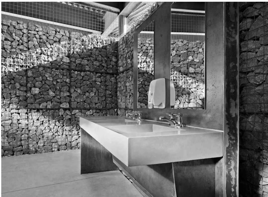
FIGURE 49. REST ROOMS, GEORGE “DOC” CAVALLIERE PARK, SCOTTSDALE, ARIZONA (2012). WEDDLE GILMORE ARCHITECTS, SCOTTSDALE, ARIZONA, AND FLOOR ASSOCIATES, INC., PHOENIX, ARIZONA, LANDSCAPE ARCHITECTS. (© Bill Timmerman.) Local stone was placed piece by piece in steel gabion cages that were used for building enclosures and retaining walls. Their color blends with the surroundings, and the construction technique requires no maintenance.
