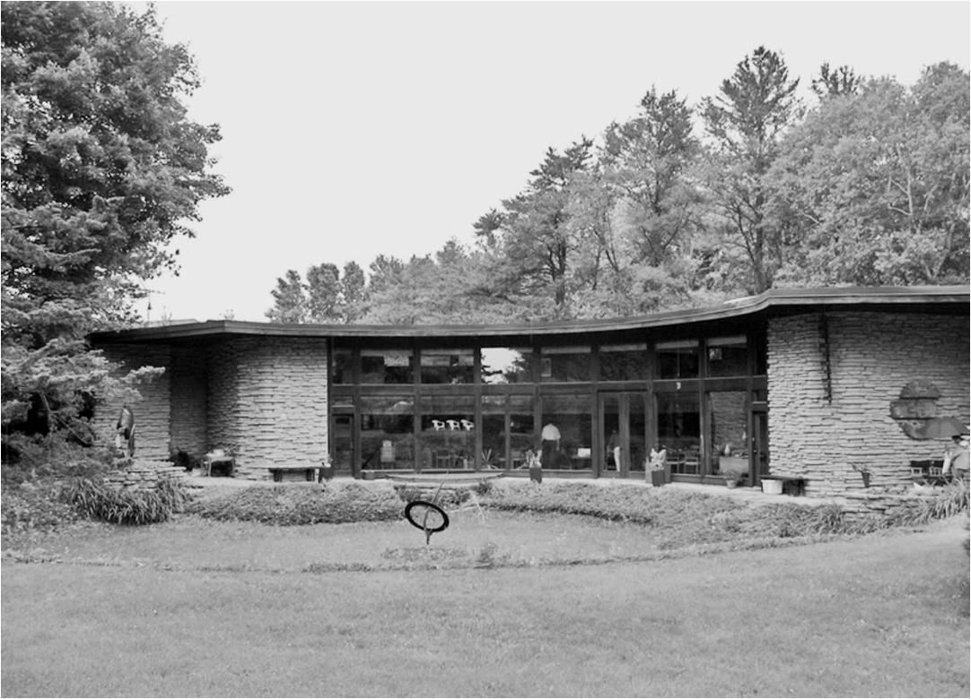
FIGURE 13. FLW SOLAR HEMICYCLE, RESIDENCE OF KATHERINE AND HERBERT JACOBS, MIDDLE-TOWN, WISCONSIN (1944). FRANK LLOYD WRIGHT, TALIESIN, WISCONSIN. This house employed many design elements recommended today for sustainable design: careful siting for passive radiant solar heating and natural cooling, with a concrete slab and limestone walls that absorb daylight and radiate heat at night; earthen berms to the south, west and north that divert cold winter winds; a fourteen-foot-high south-facing glass wall that allows winter sunlight to enter, with large roof overhang to shade the sunlight during the summer; and cross ventilation flowing from windows on the lower level to the north-facing clerestory windows on the upper level. This house was designated a National Historic Landmark Building in 2003.
