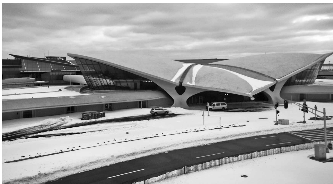
FIGURE 3. TWA FLIGHT CENTER, JOHN F. KENNEDY INTERNATIONAL AIRPORT, NEW YORK (1956–1962). SAARINEN AND ASSOCIATES, ARCHITECTS, HAMDEN, CONNECTICUT. Saarinen captured a sense of flight in the flowing forms of the concrete roof shell. The large and clear-span interior spaces have proved to be ideal for changing terminal services. This building was placed on the National Register of Historic Places in 2005.
