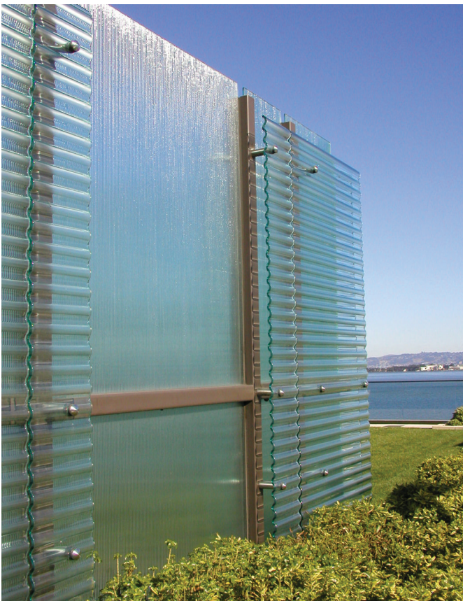
FIGURE 34. GAP HEADQUARTERS, SAN FRANCISCO (1998–2001). OLIN, PHILADELPHIA AND LOS ANGELES. (© OLIN.) Textured glass walls are layered to conceal the mechanical equipment and to provide screens that block the wind and the noise for people sitting in the roof garden. Situated next to a noisy freeway and on the flight path of San Francisco International Airport, this design provides acoustic and thermal benefits.
