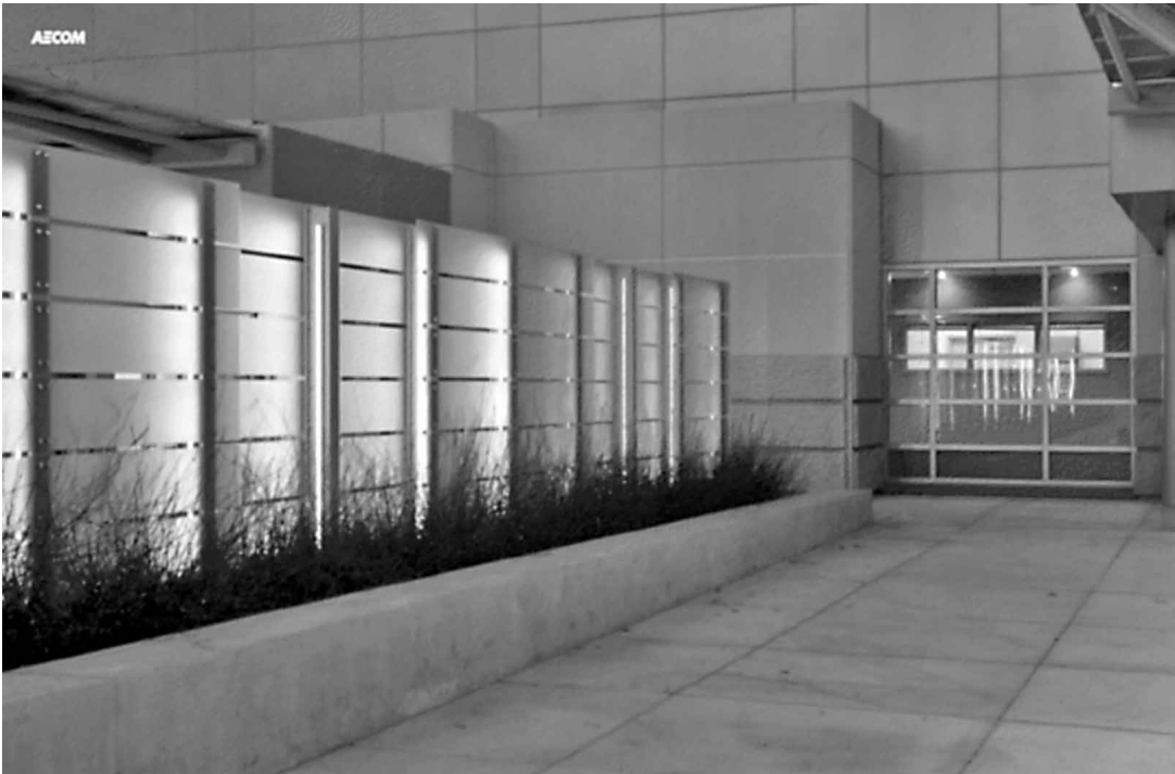
FIGURE 71. EL CAMINO HOSPITAL, MOUNTAIN VIEW, CALIFORNIA (2009). AECOM, U.S. WEST, SAN FRANCISCO. (Photography by David Lloyd, © AECOM.) Emergency rooms are places of high anxiety. Illuminated acrylic panels were used for a screen wall to project a sense of calm and care. They provide a backdrop for plants, which are reminders of growth and life.
