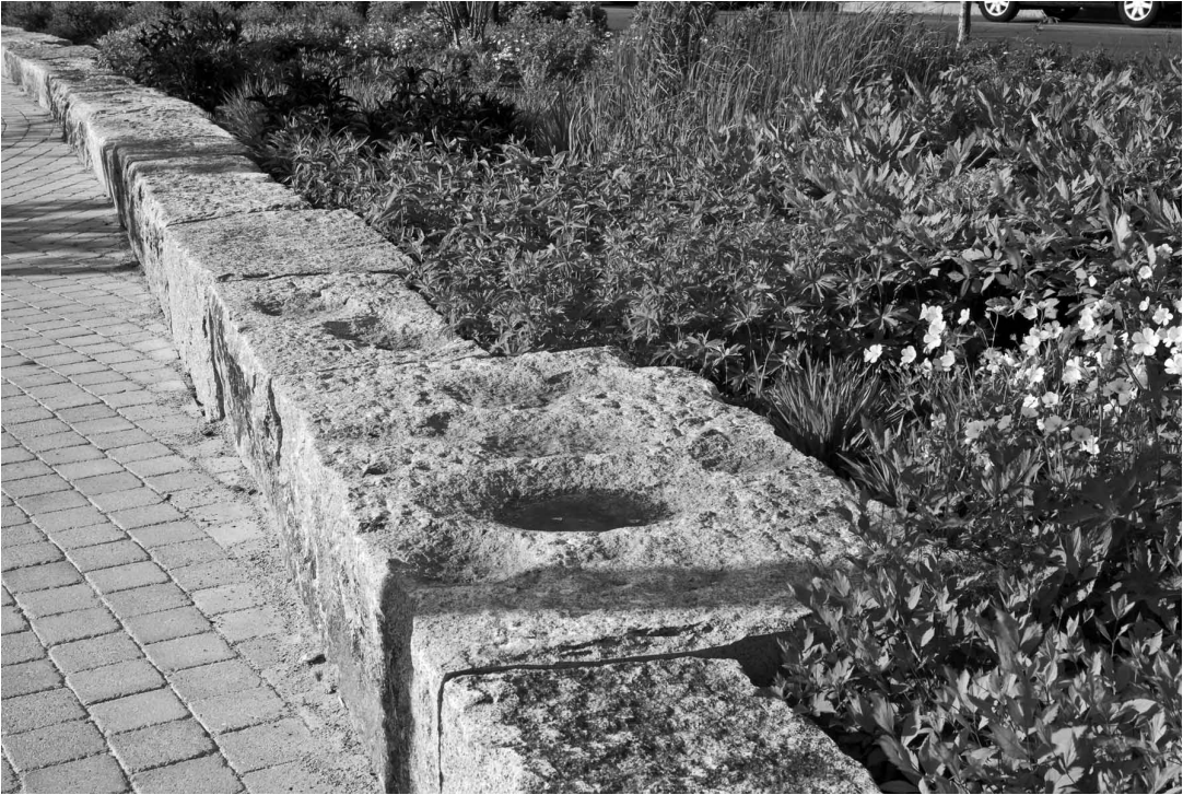
FIGURE 50. WHARF DISTRICT PARK, BOSTON (2008). AECOM (FORMERLY EDAAW, VIRGINIA) AND COPLEY WOLFF DESIGN GROUP. (Photograph by Dixi Carrillo, © AECOM.) Granite stock-piled from a waterfront redevelopment that was part of the Big Dig was salvaged and reused as seats and retaining walls. The front and top surfaces were aligned and the stone sides were cut for a tight, mortared fit. Once installed, the sharp front top edge was sanded round for more comfortable use.
