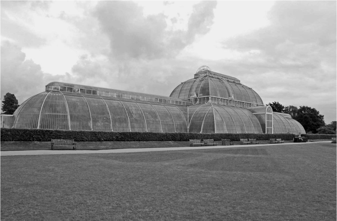
FIGURE 37. THE PALM HOUSE, KEW ROYAL BOTANIC GARDENS, LONDON (1844–1848). DECIMUS BURTON AND RICHARD TURNER, LONDON. (Courtesy Magenta Livengood.) This important surviving Victorian-era glass-and-iron structure was designed to create a suitable habitat for the exotic palm collection.
