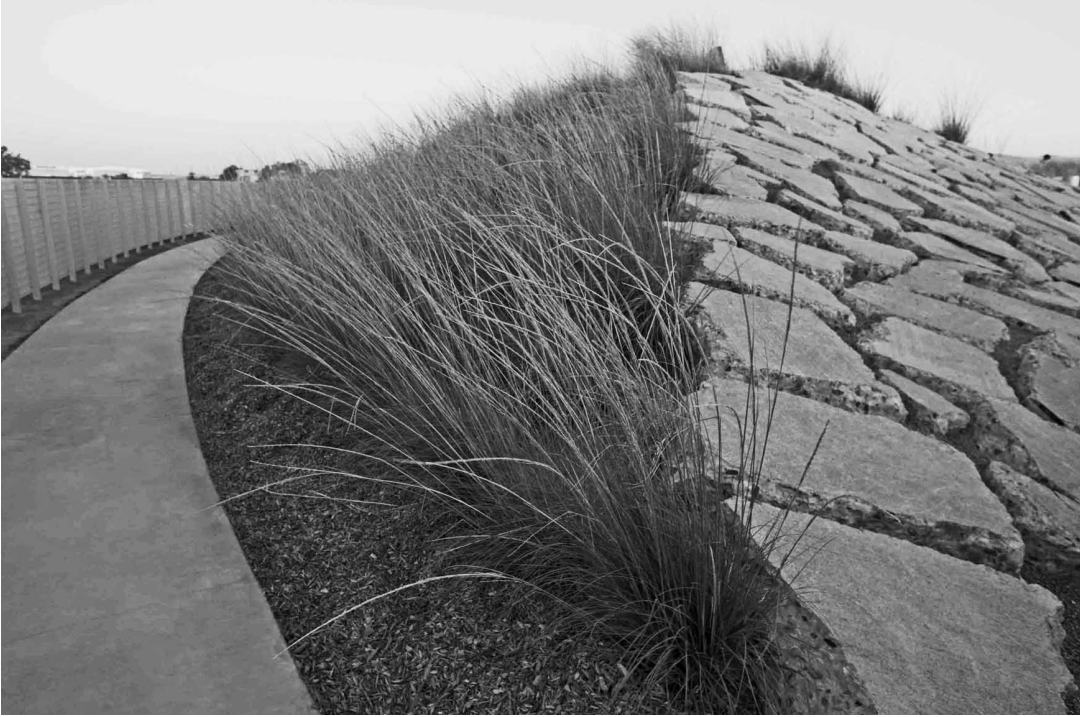
FIGURE 8. ORANGE COUNTY GREAT PARK, CALIFORNIA (PHASE ONE, 2010–2013). WORKSHOP: KEN SMITH LANDSCAPE ARCHITECT, NEW YORK. (© Tom Lamb/Lamb Studio.) Approximately 600 acres of concrete runway paving from the existing airport was repurposed for several uses on site, including fragments stabilizing earthen mounds.
