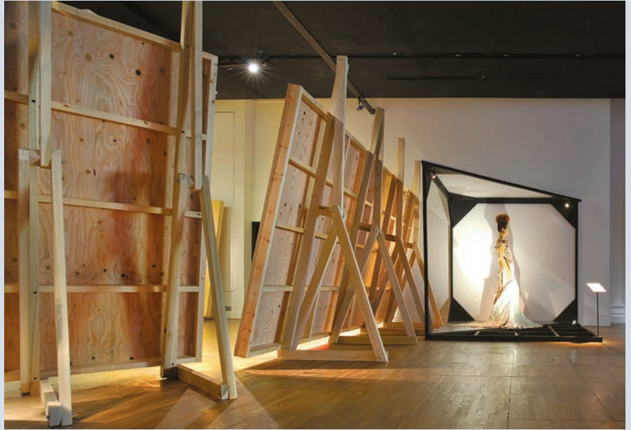
Above A single-sided structure leans back on the support structure for stability.
