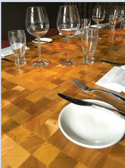
Left End-grain squares, glued to a plywood base board, provide both regular and irregular patterning.
