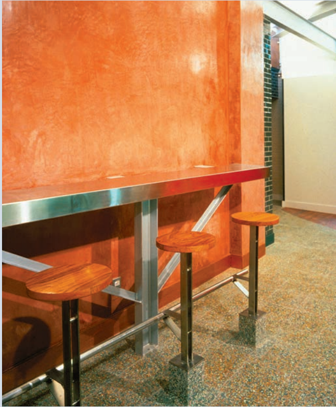
Above The stainless-steel wall shelf is supported on substantial steel sections and the footrest on the stools' paired steel stems.
